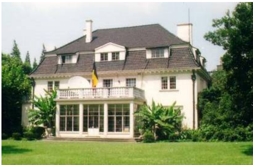
Fig. 23. French Consulate – Type 2 protection, protect mainly the exterior of the buildings, internal lobby, staircase and interior decoration. (from Presentation by Wujiang, Deputy Director of Shanghai Urban Planning Administration Bureau. 2007.)
