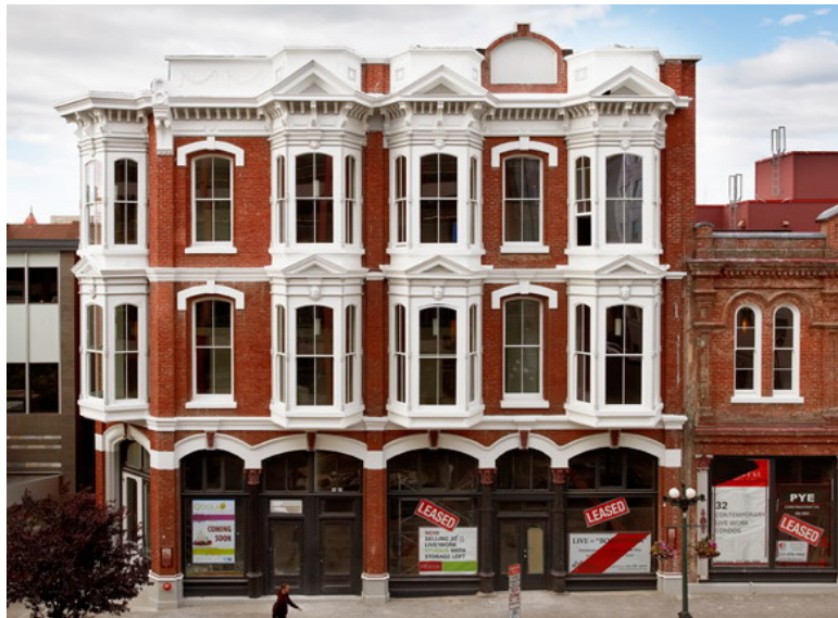
Fig. 6. The rehabilitation of the Oriental Hotel in Victoria benefitted from the city's Tax Incentive Program.
