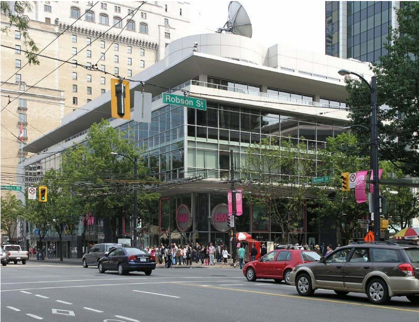
Fig. 1 The former Vancouver Public Library (1957, altered 1996) has been designated (protected) under the Recent Landmarks Program.
