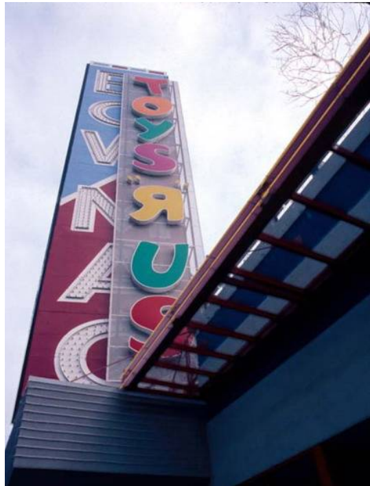
Fig. 12. The landmark BowMac sign (1959) was conserved and overlaid with a new, non-conforming sign for Toys 'R' Us.
