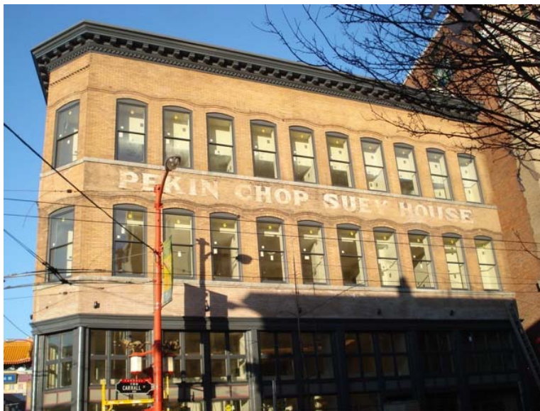
Fig. 5. The exterior of the Chinese Freemasons Building in Vancouver was restored with assistance from the former Commercial Heritage Properties Incentive Fund.
