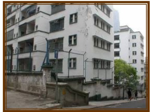
沿士丹頓街和鴨巴甸街的圍牆上的 原有花崗石基座和柱 Granite plinths & pillars of fenced walls along Staunton Street & Aberdeen Road
