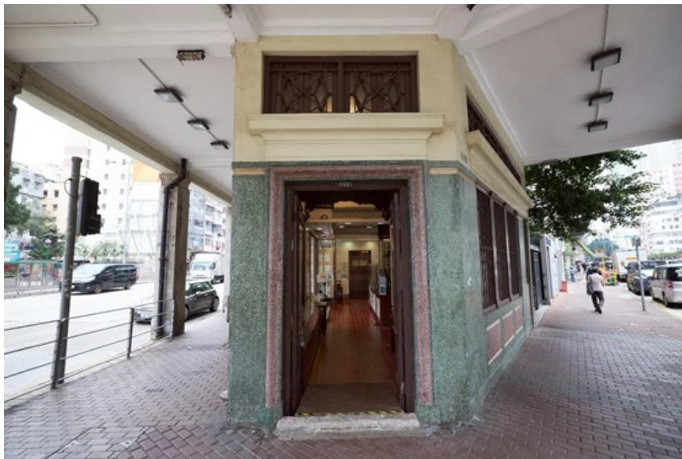
Entrance of the shop, finished with terrazzo exterior walls and timber windows with iron grilles on the top.
