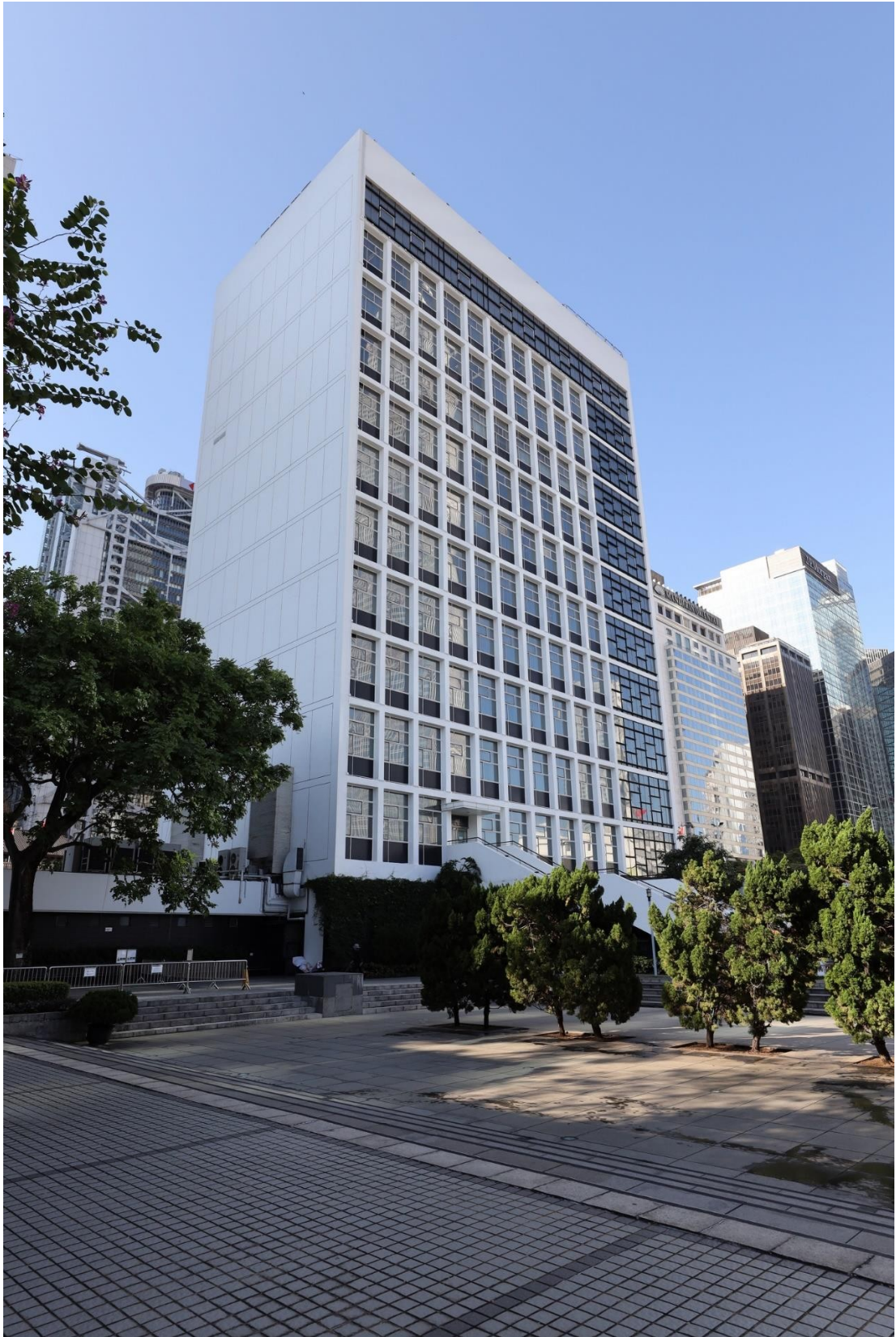
The north façade of High Block with “an uncomplicated repetitive fenestration in a concrete frame”; while the east façade is plastered white.
