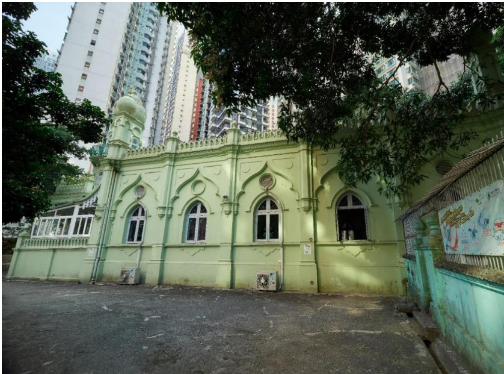
Side elevation of Jamia Mosque with pointed arch windows and simple motifs.
