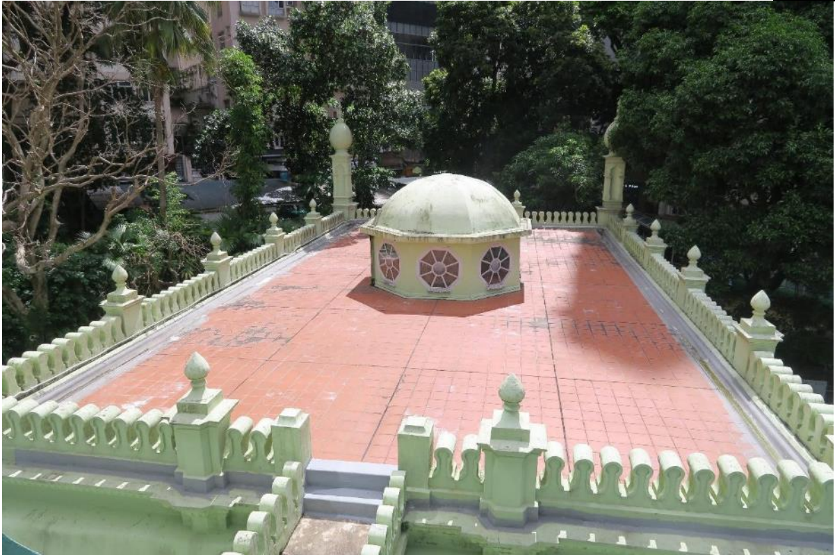
The roof parapets decorated by rounded merlons, with pedestals crowned by finial at intervals.
