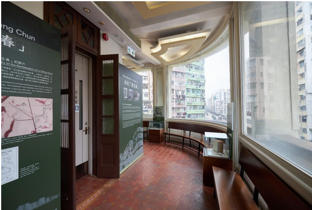
Original elements such as floor tiles and timber doors are preserved at the verandah on the 3/F.
