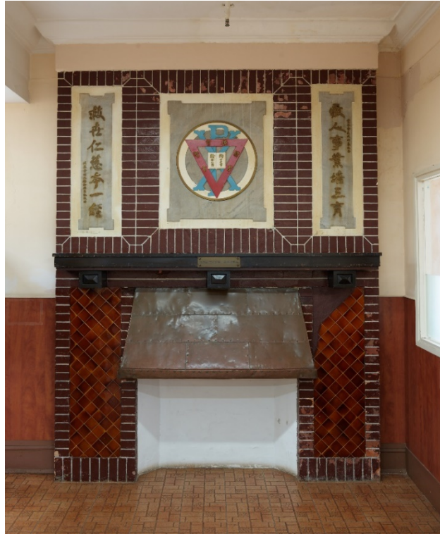
The fireplace on ground floor. The emblem of YMCA and couplets backed with marble plate and slabs are on top of the mantel.
