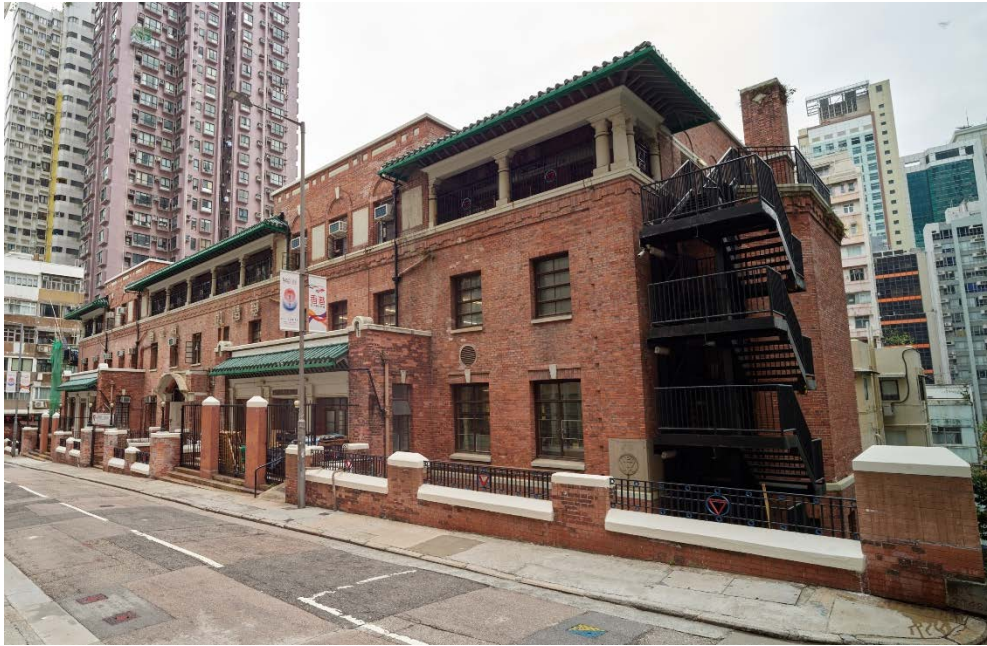
Tuscan columns and green glazed tiled eaves at the front elevation of the Central Building
