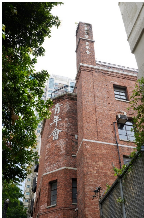
The side and rear elevations of the Central Building looking from Ladder Street. The Chinese name of YMCA are installed at prominent positions.
