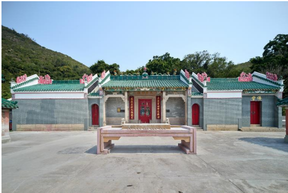
The front façade of Tin Hau Temple, Joss House Bay
