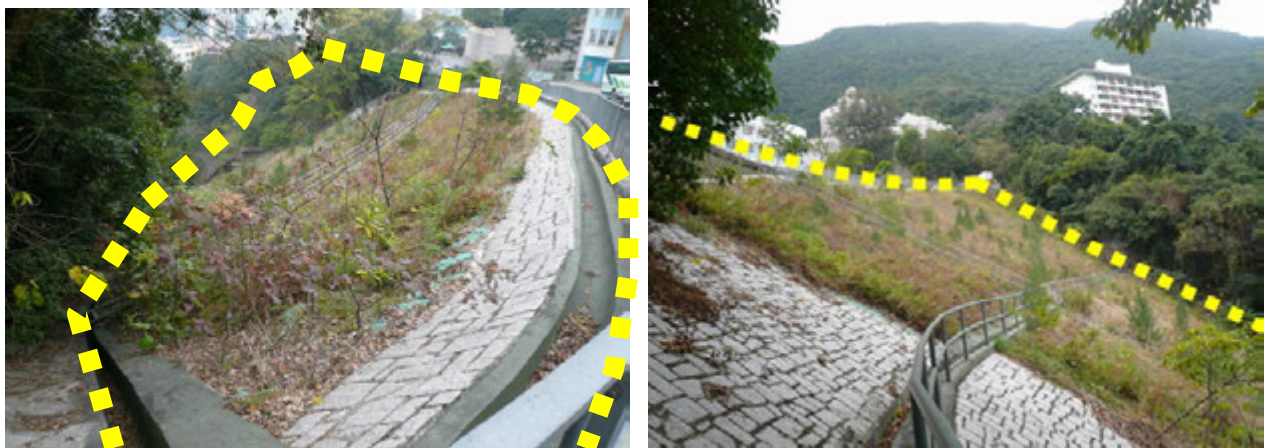
View on the man-made slope as at January 2008
