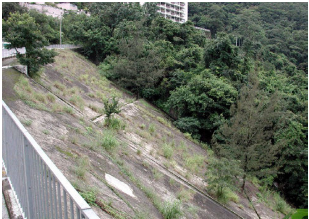
View on the slope when stabilisation works began in 2002
