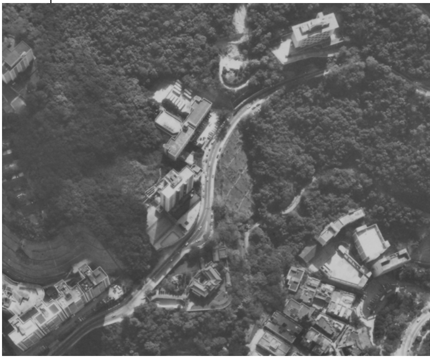
Aerial view of the slope in 1990 kept in Geotechnical Engineering Office
