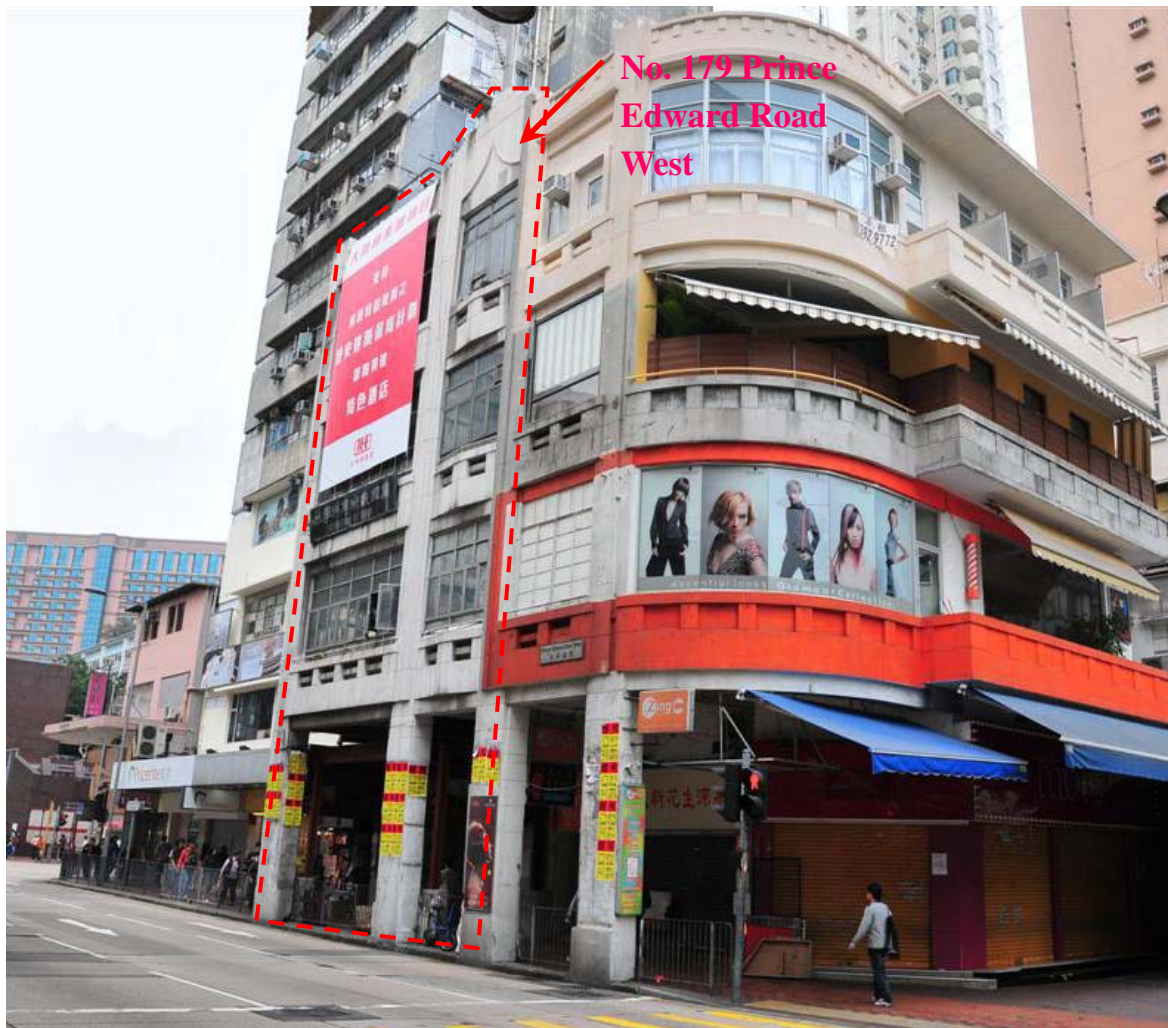
Front view of the existing shophouse
