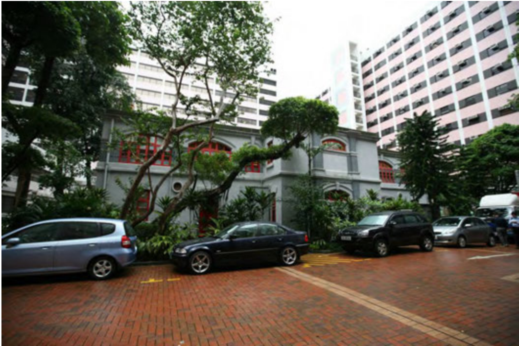
Western-style window openings and wall decorations of the rear elevation
