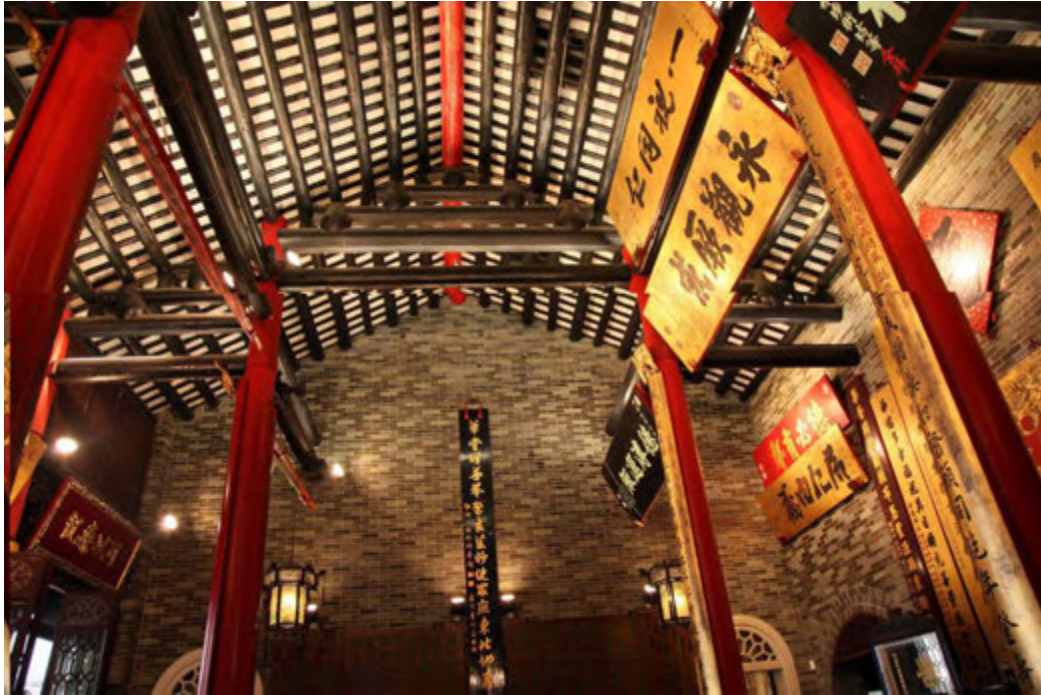
The Chinese truss system inside the main hall
