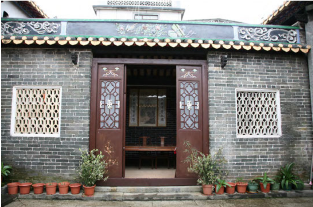
The wooden latticed doors and ceramic window grilles of the side chamber
