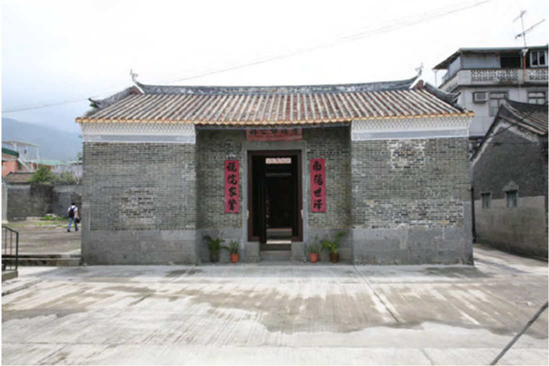
The front elevation of the Tang Kwong U Ancestral Hall
