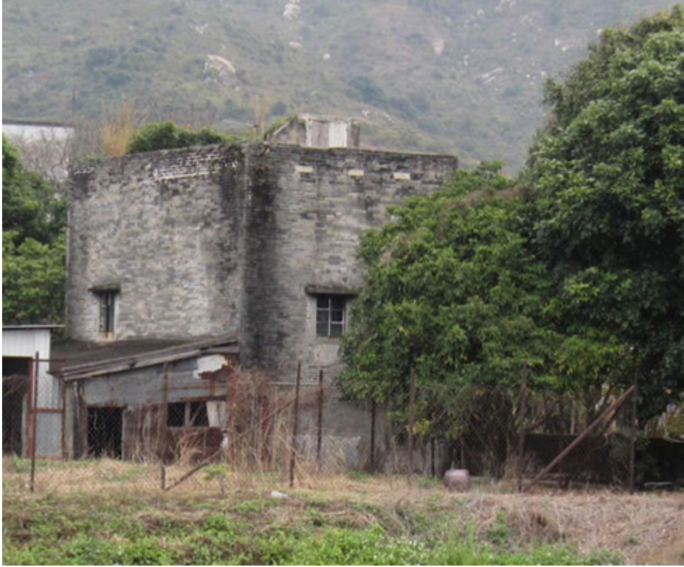
North elevation of the Building
