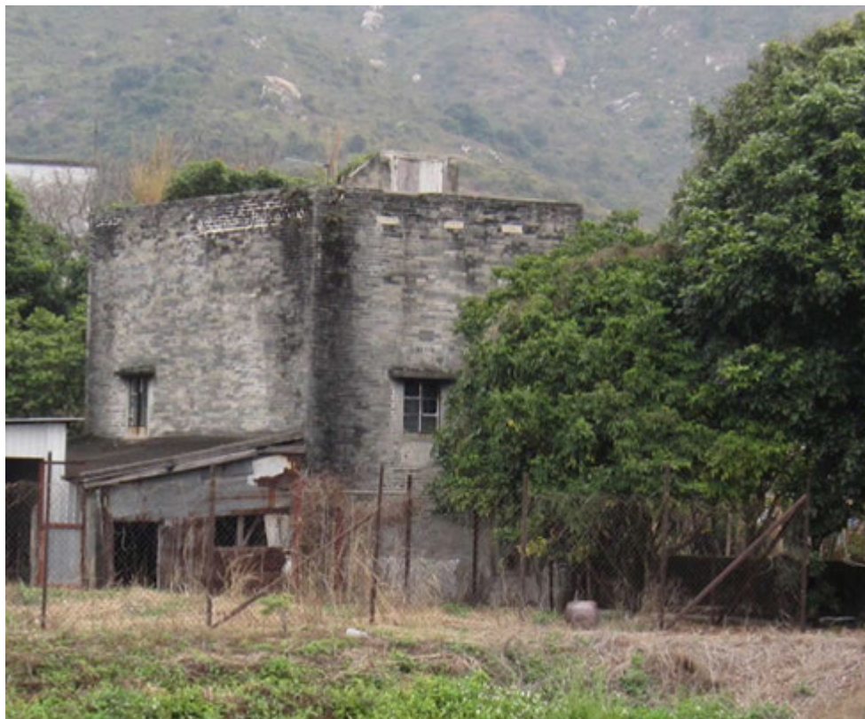
North elevation of the fortified structure
