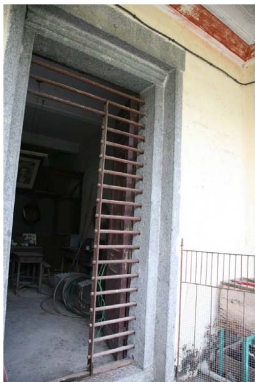
Metal sliding door at the main entrance
