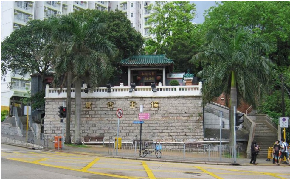
Hau Wong Temple Compound is situated on a terrace with granite steps leading down to Junction Road
