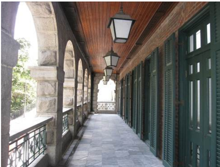
Open verandah, with pendant lights, boarded ceiling and timber shutter doors added during the 2002 renovation.
