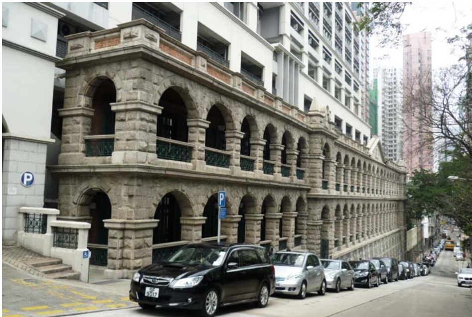
General view of the elevation facing High Street showing the impressive rusticated granite blocks of the façade.
