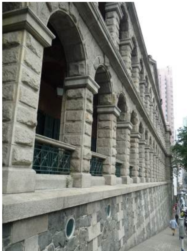
Close up showing random pattern of granite blocks on lowest level and the rusticated treatment of the granite blocks to the two upper storeys.
