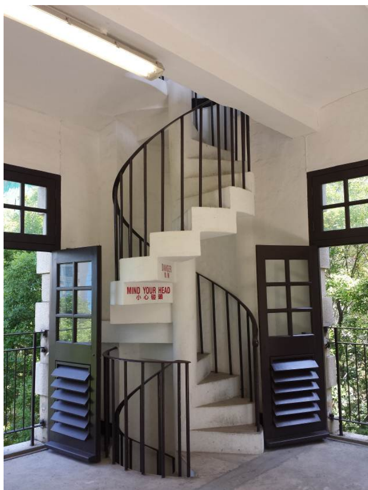
Concrete and steel spiral staircase on 1/F
