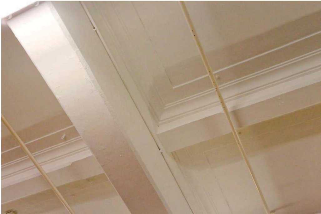
Classical plaster mouldings to the ceiling cornices.
