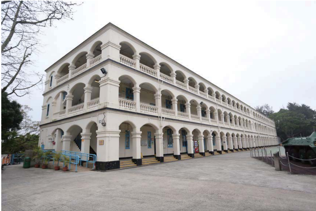
The east facade featuring the long open arched, colonnaded and balustraded verandahs.
