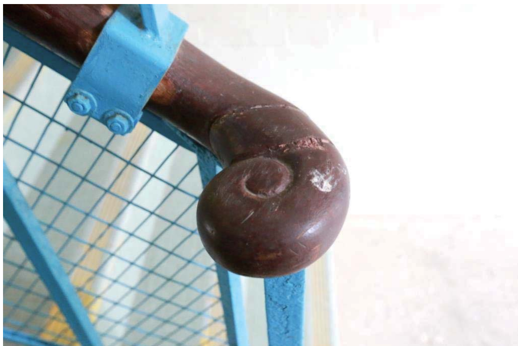
The handrail scroll of an internal staircase.
