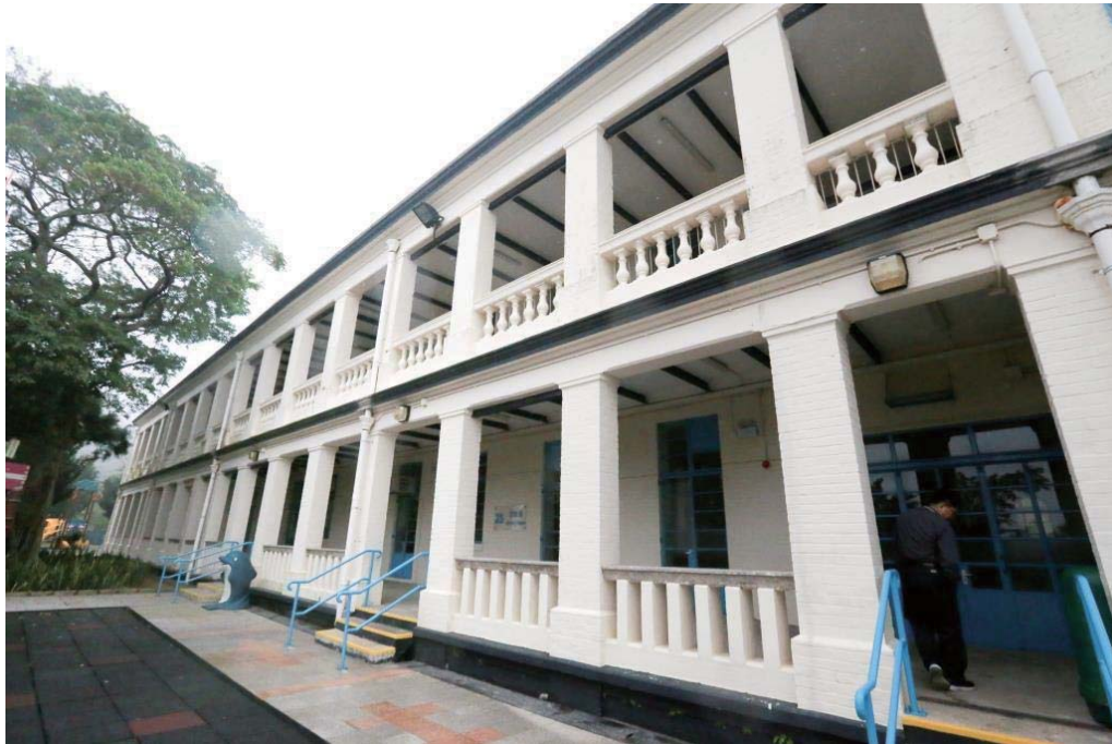
East facade with open colonnaded and balustraded verandahs supported by square brick columns with simple bases and capitals.
