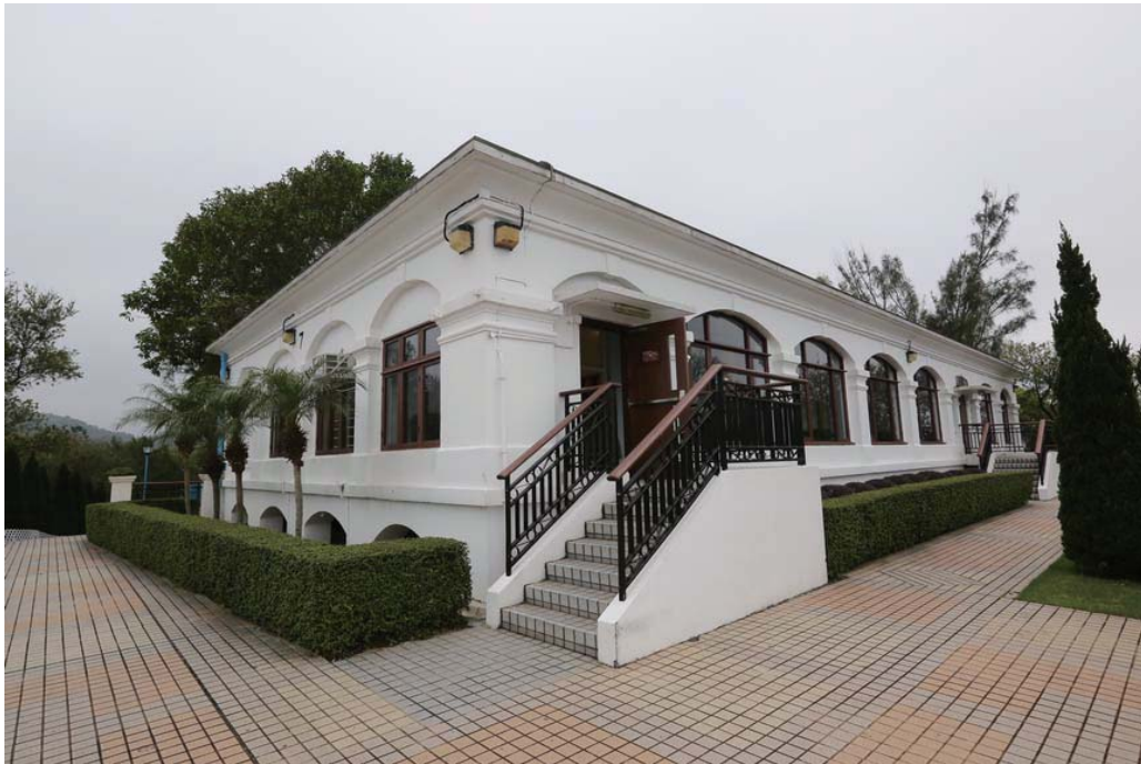
The north and east facades, originally surrounded by wide verandahs set on low segmental arches.
