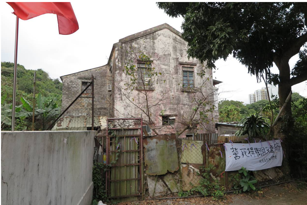
Side elevation of Hung Lau, photo taken on 21 February 2017
