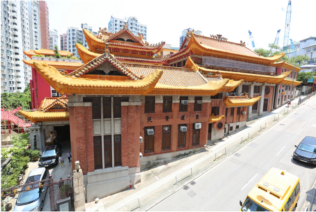
Tung Lin Kok Yuen from Shan Kwong Road. The roof of the Main Hall is in double-eave hip-and-gable style.
