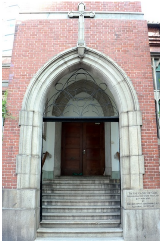
Pointed arch doorway at the main entrance with carved granite cross and foundation stone.
