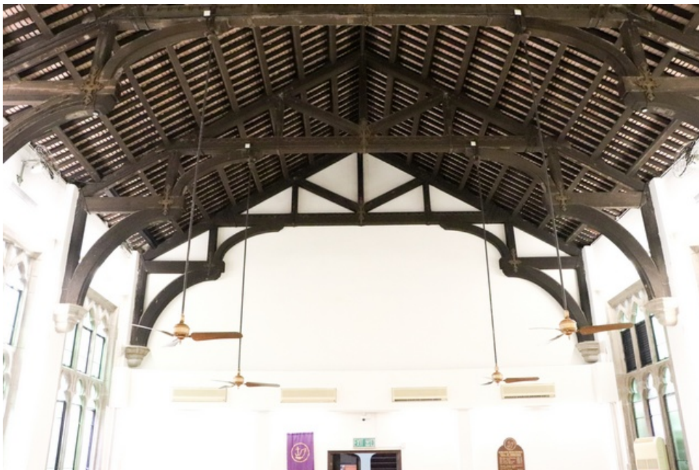
Elegant double hammer-beam timber roof trusses with carved granite corbel supports.
