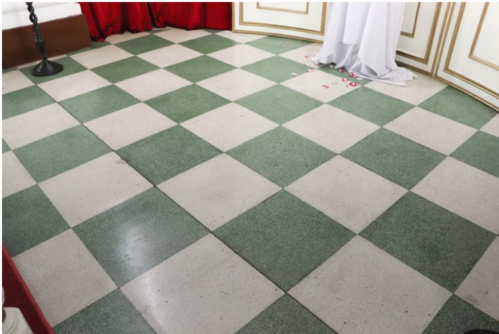
Original green and white terrazzo flooring at the main hall.
