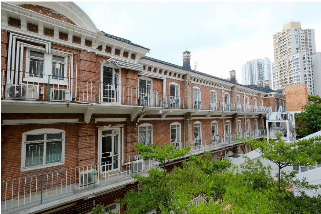
Rear elevation facing May Hall
