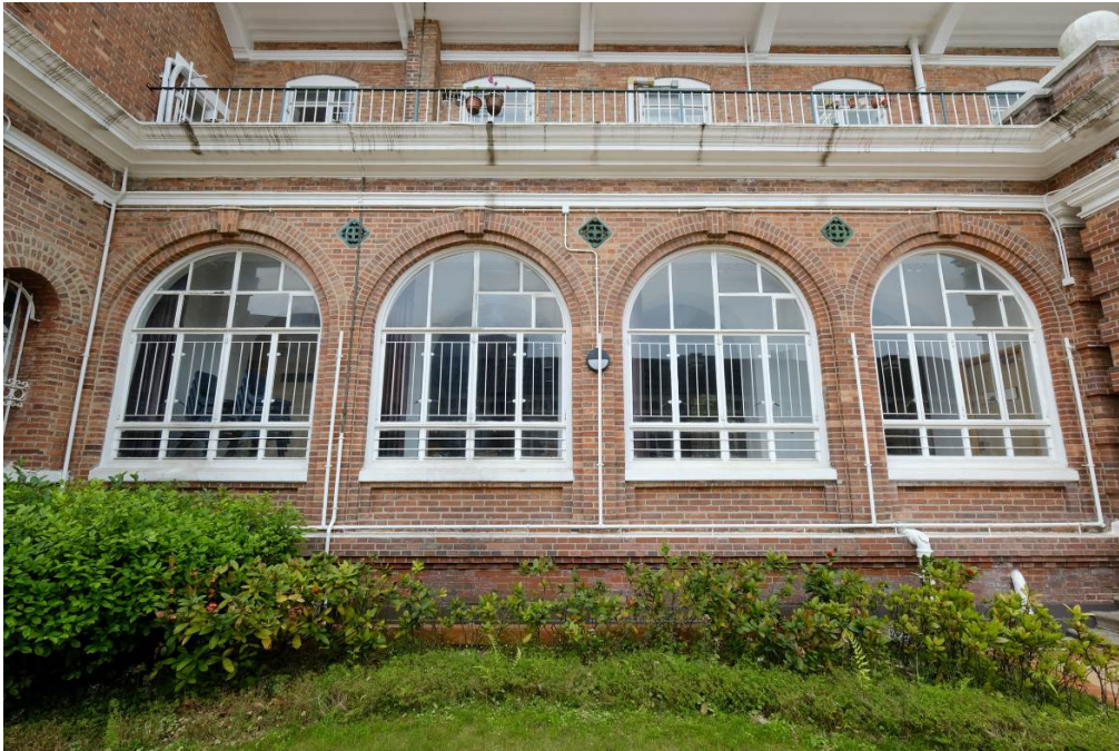
Enclosed verandah (north elevation) on the ground floor
