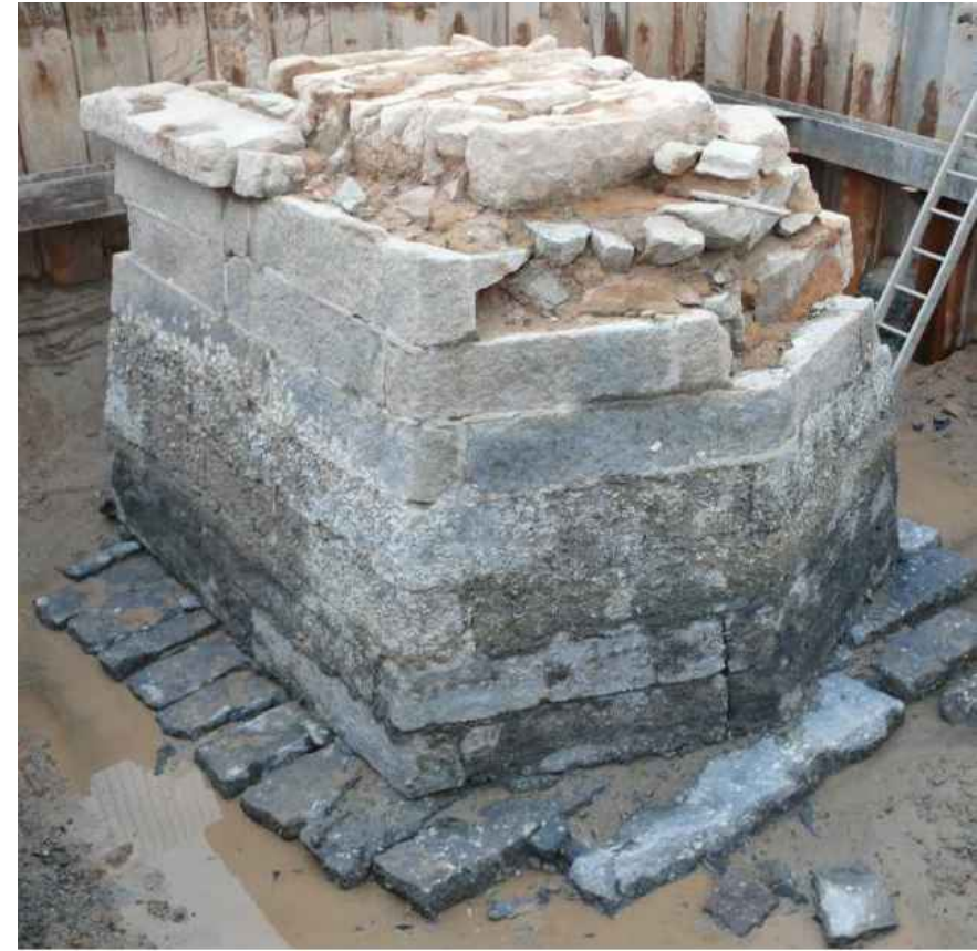
圖B - 橋墩遺跡 (位置見附錄3) FIGURE B - REMNANTS OF STONE SUPPORTING PILLAR (LOCATION OF REMNANTS REFERS TO ENCLOSURE 3)
