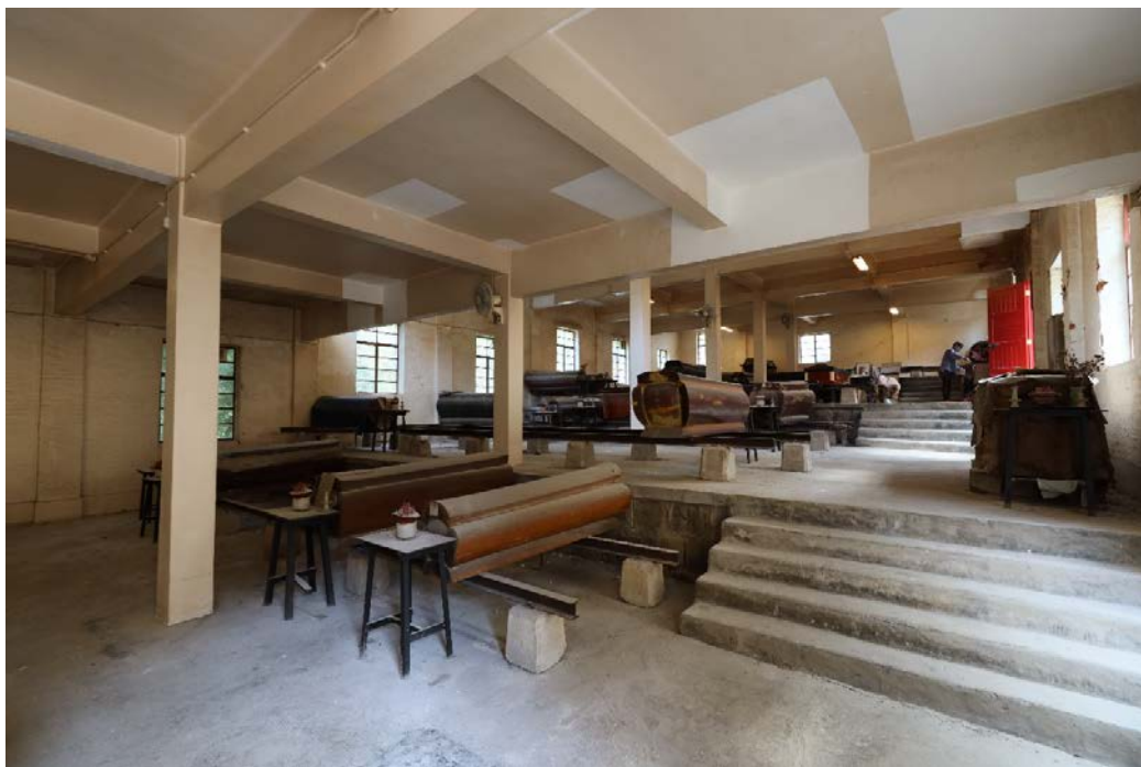
Interior of the New Hall. It is a flat concrete roofed building supported by rectangular columns.
