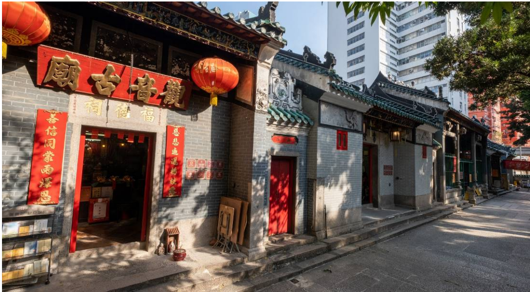
The five temple buildings, i.e. Tin Hau Temple, Kung Sor (公所), Fook Tak Tsz (福德祠) and two Shu Yuen (書院), were built between 1876 and 1920.
