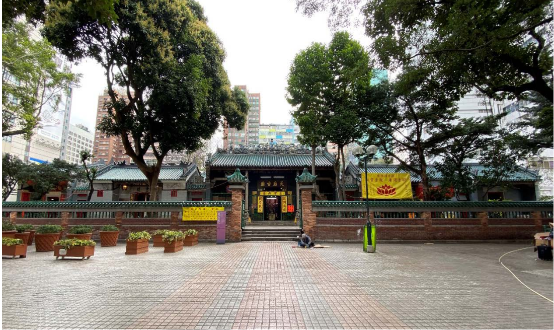
Front elevation of Tin Hau Temple and the adjoining buildings
