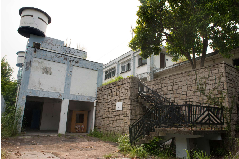
Existing Condition of the Former Lau Fau Shan Police Station 前流浮山警署的現貌
