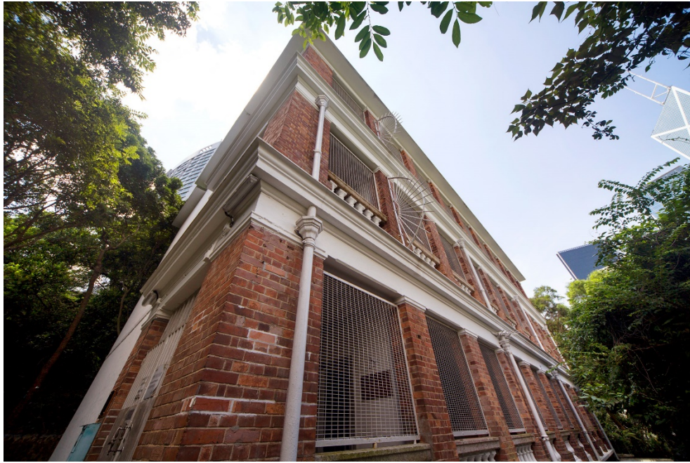
Existing Condition of the Roberts Block, Old Victoria Barracks 舊域多利軍營羅拔時樓的現貌
