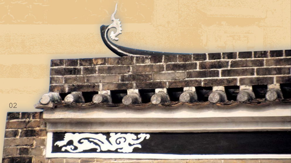
02 門樓屋頂上之龍形翹角正脊 Main ridge with curled up ends in dragon shape at the roof of the Gate Tower
