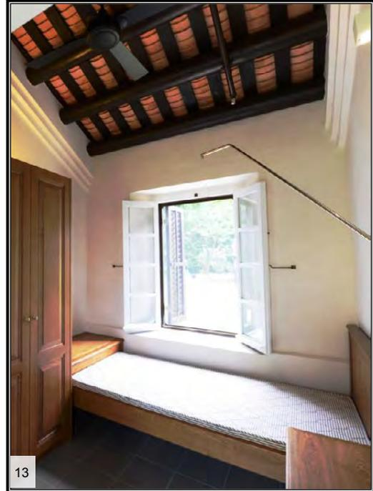
Reconstructed timber purlins and battens are protected with fire retardant paint
