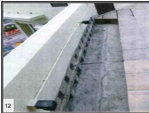
Canton tiles with insulation layer removed along the parapet walls
