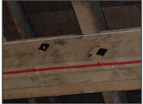
Photos 8 and 9 Three timber joists bolted together
