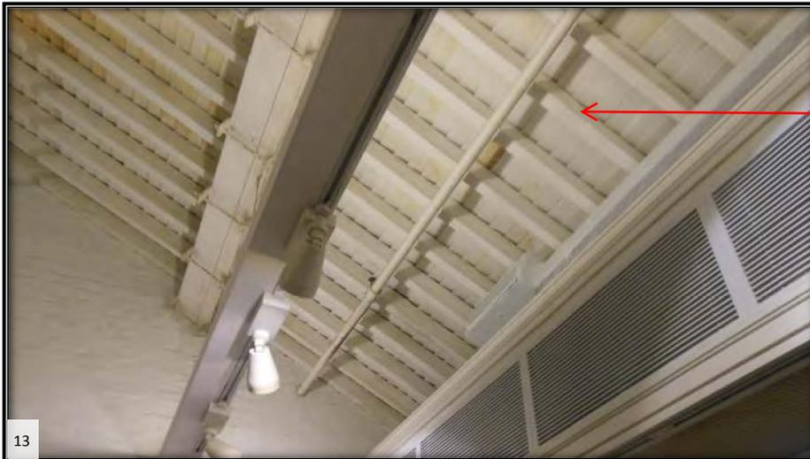
Timber pitched roof protected with fire retardant paint
