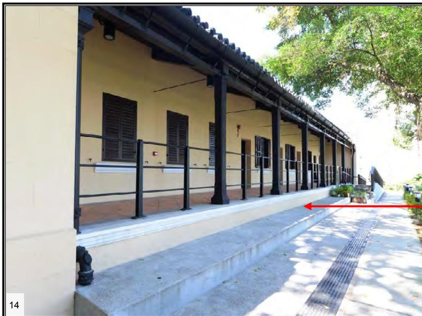
Intermediate platform added to mitigate level difference
