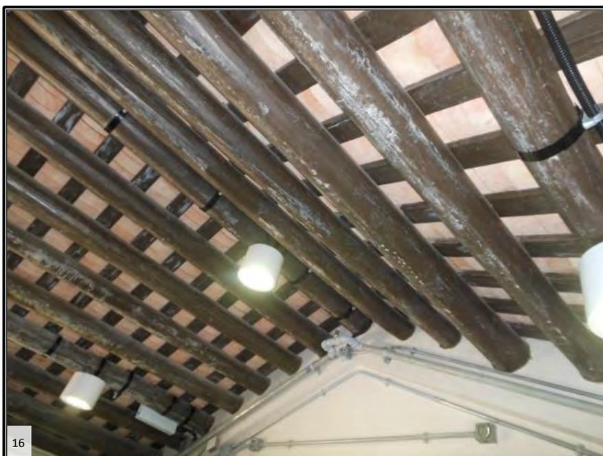
Existing timber pitch roof are retained for appreciation but timber elements are painted with fire retardant paint
