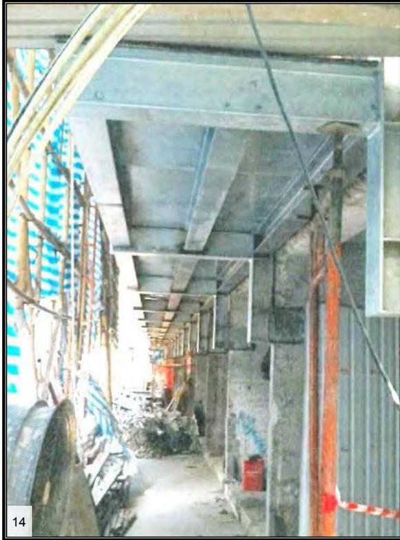
Corridor slabs were demolished and replaced by new structural steel decks
