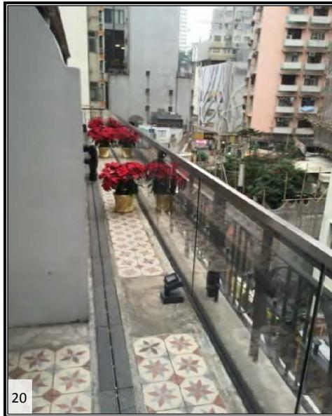
New glass balustrade added behind the existing railing at accessible balconies
