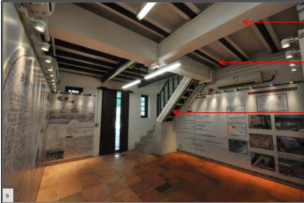
Existing RC beams supporting timber floor & staircase
