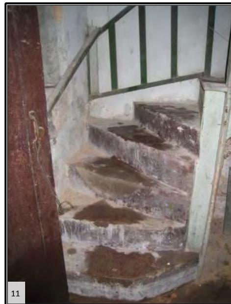
Existing timber staircase with solid winders at the bottom before revitalisation
