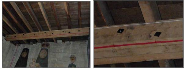
Photos 8 and 9 Three timber joists bolted together
