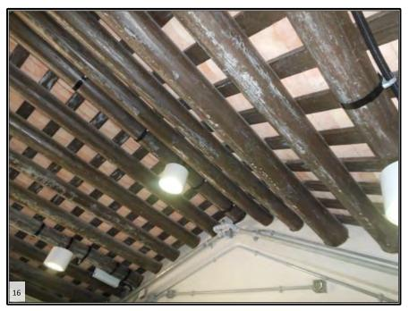
Existing timber pitch roof are retained for appreciation but timber elements are painted with fire retardant paint
