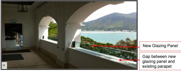
Additional glazing panels to add height to the existing parapet walls in the Main Building
