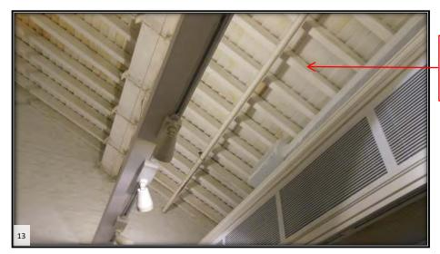
Timber element protected with fire retardant paint
