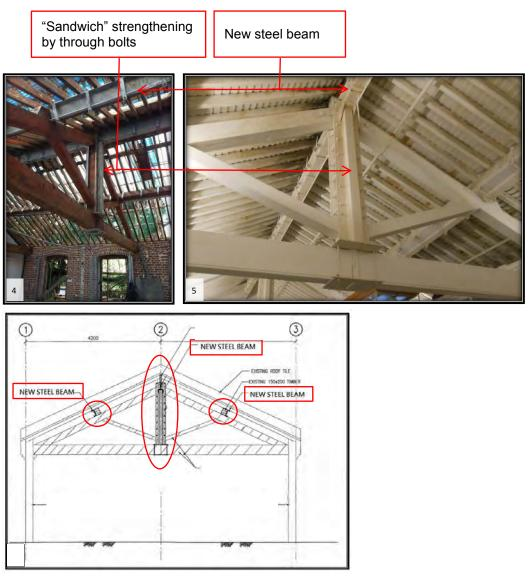
Photo and section showing strengthening to the structural elements and connection joints of roofs of buildings in the Low Zone (Source: P&T Architects and Engineers Ltd.)
