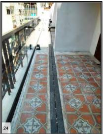
Passageway shall have a clear width of not less than 1050mm in accordance with the Design Manual: Barrier Free Access 2008 (DMBFA).
