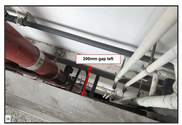
200mm gap was left after partial removal of the existing floor beams
