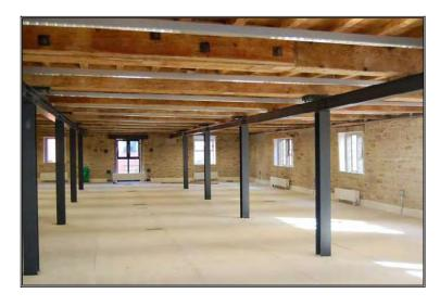
Photo 7 New beams and columns underneath the timber Joists
