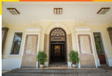
入口拱門上置西式半圓楣窗。 A western-style semi-circular fanlight above the arched doorway.
