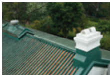
設煙囪的中式金字屋頂。 Chimneys on the Chinese-style pitched roofs.
