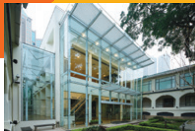
以玻璃幕牆取代展覽大樓外牆，擴闊主樓空間。 A glazed wall replaced the front elevation of the extension building to enhance the foyer space.
