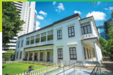
以多立克式（地下）和愛奧尼柱式（一樓）組成的開放式柱廊。 The open colonnaded verandahs feature columns in Doric order on the ground floor and Ionic order on the first floor.
