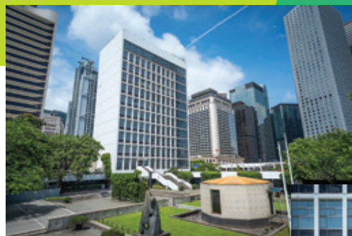
高座正立面以混凝土格網和簡約的組合式窗台設計。 The High Block's façade design features a concrete grid and simple modular window bays.
