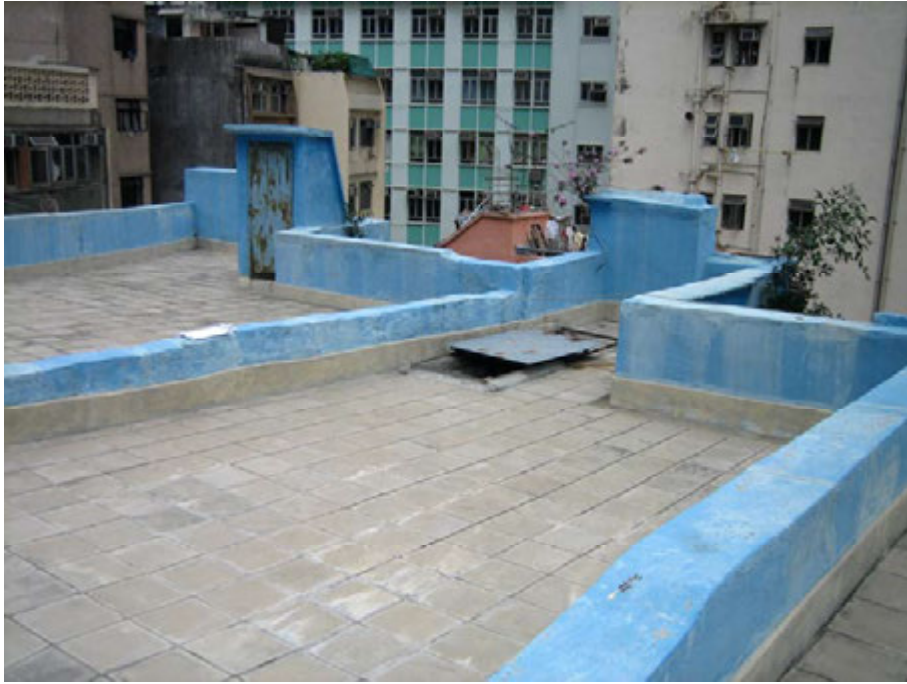
Roofs of 72 and 72A Stone Nullah Lane
