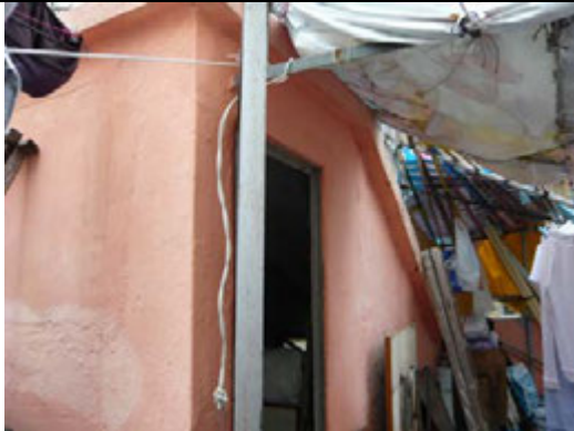
3.3) Roof - The parapet walls and the staircase hood
