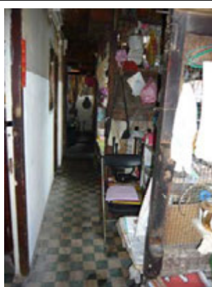
3.4) Flooring - Green and white ceramic tiling in the common areas
