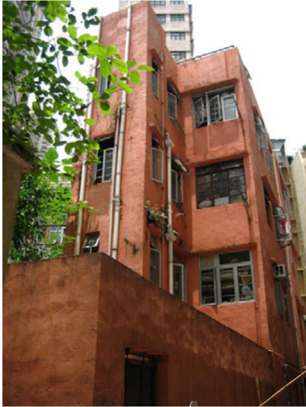
Rear facade of 8 King Sing Street
