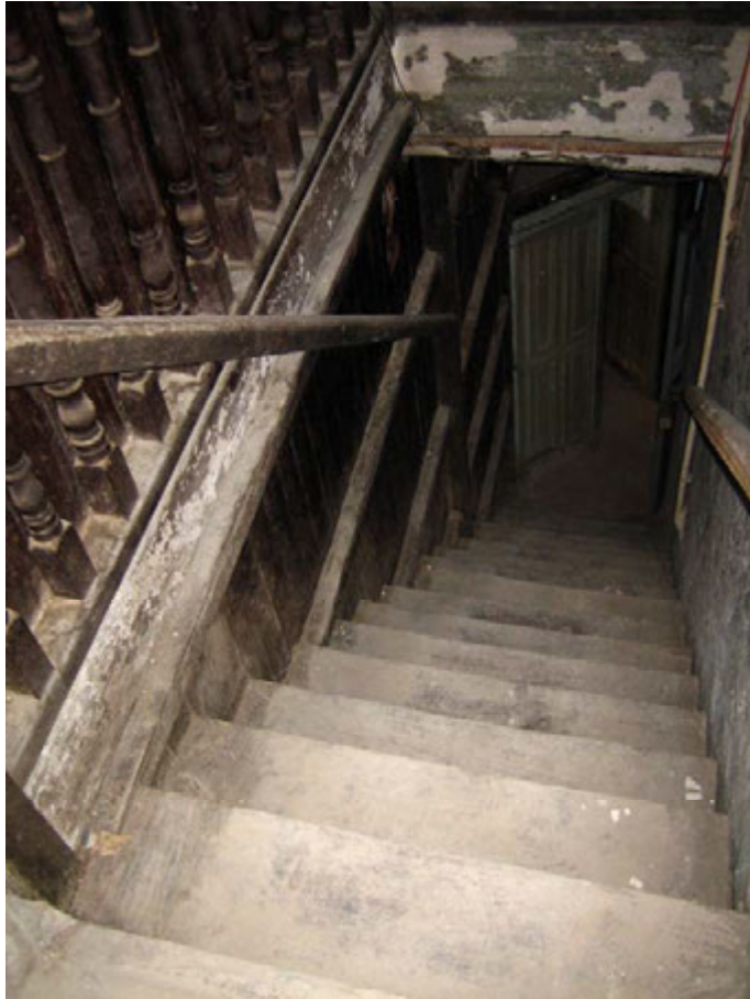
View of one internal timber stair
