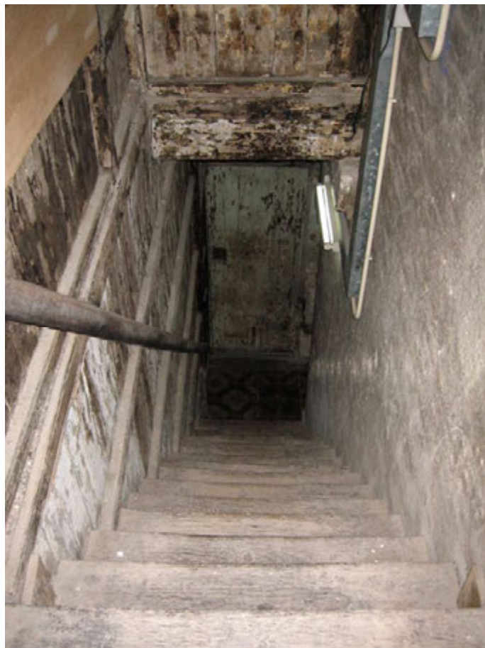
View of one internal timber stair
