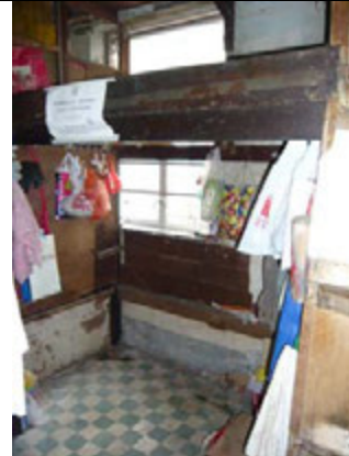
3.4) Flooring - Green and white ceramic tiling in the common areas
