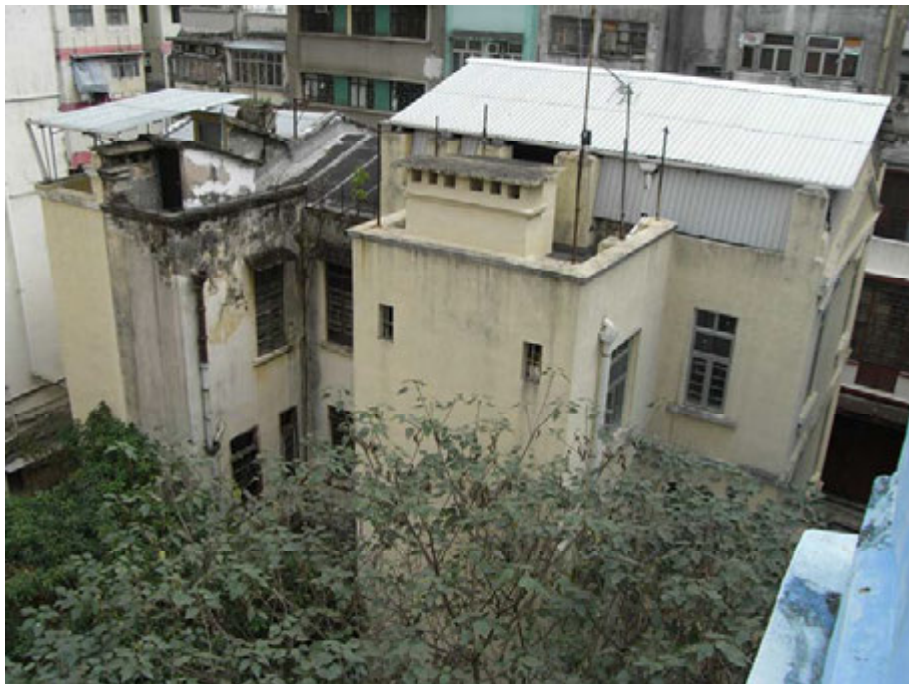
Rear facade of 2-8 Hing Wan Street
