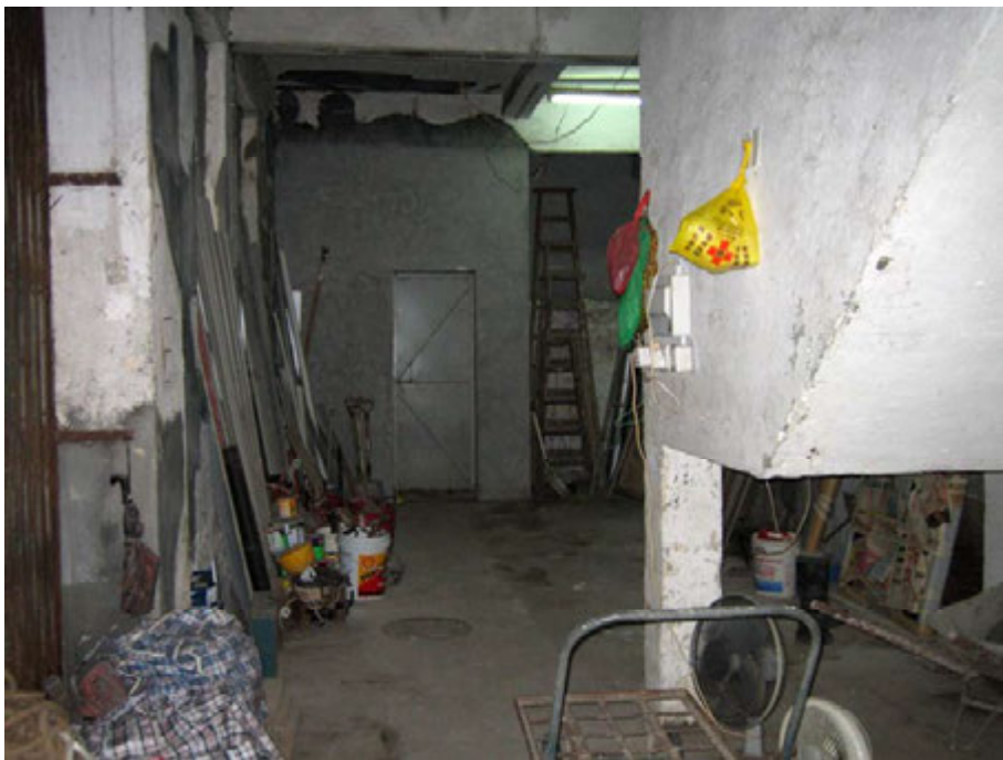
View of the vacant unit on ground floor (view 2)
