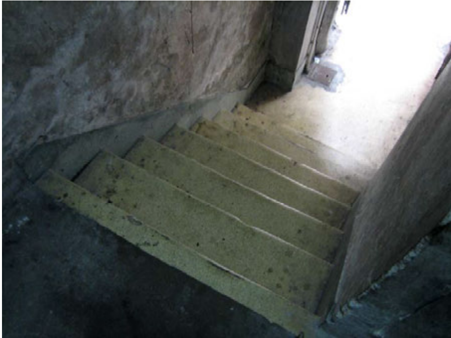
View of one internal reinforced concrete staircase
