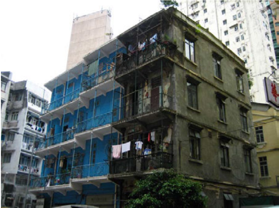
Front and side facades of 72-74A Stone Nullah Lane
