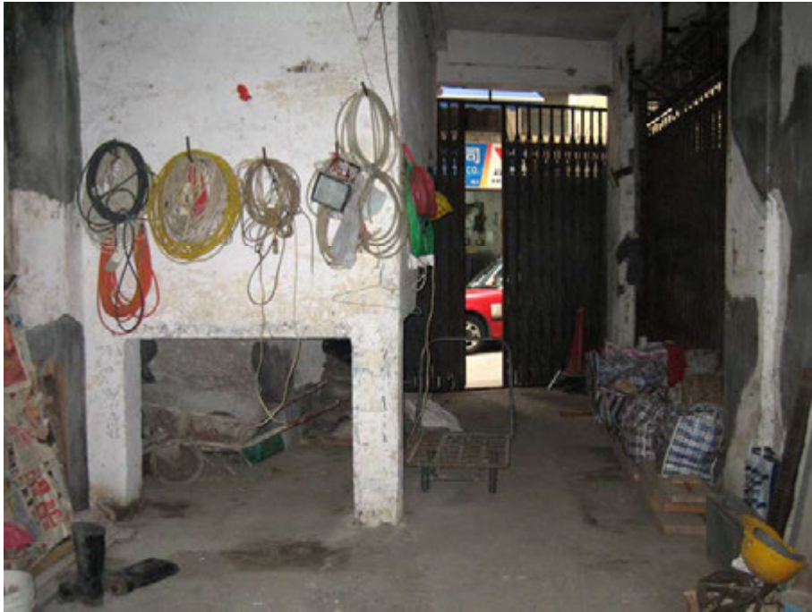
View of the vacant shop on ground floor (view 1)
