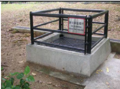
3.3) The water well located next to the House
