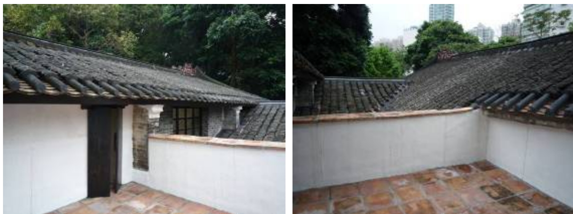
Flat roof of the Old House
