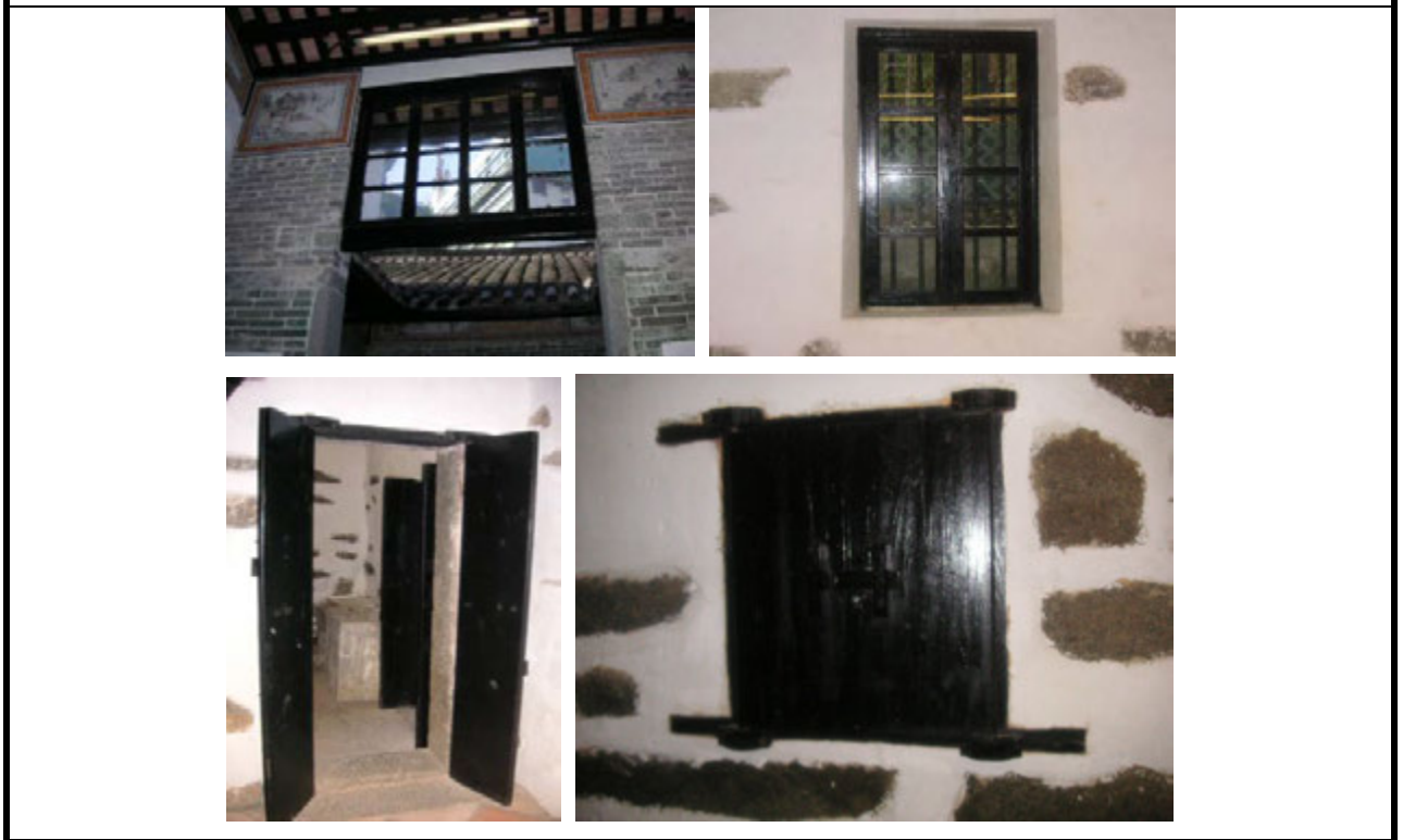
2.8) Timber fan light, shutters, doors and windows and their openings
