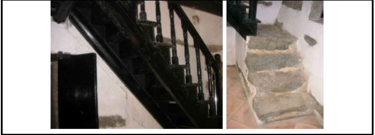
2.10) Timber staircase, granite landings and ornamental balustrades in the four side rooms
