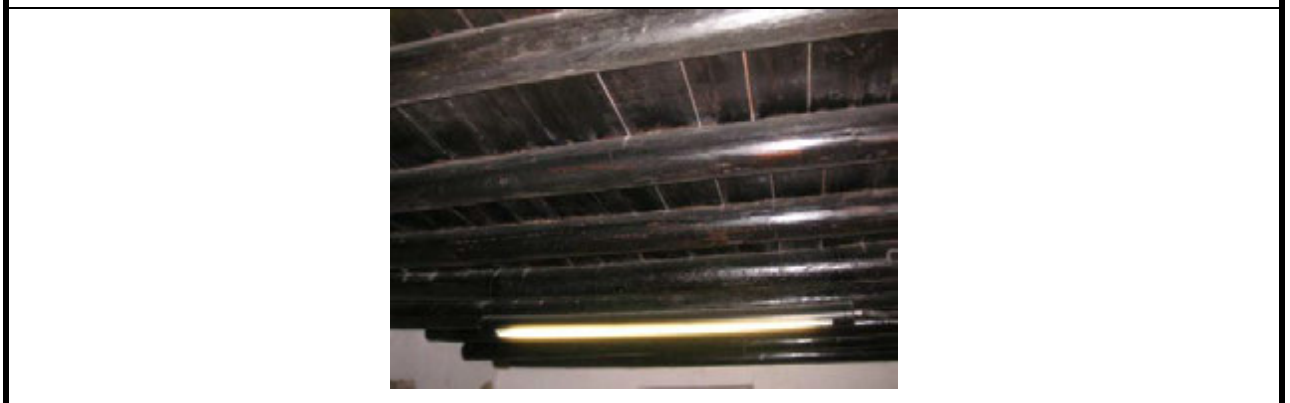
2.9) Timber joists and battens of the cocklofts in the four side rooms
