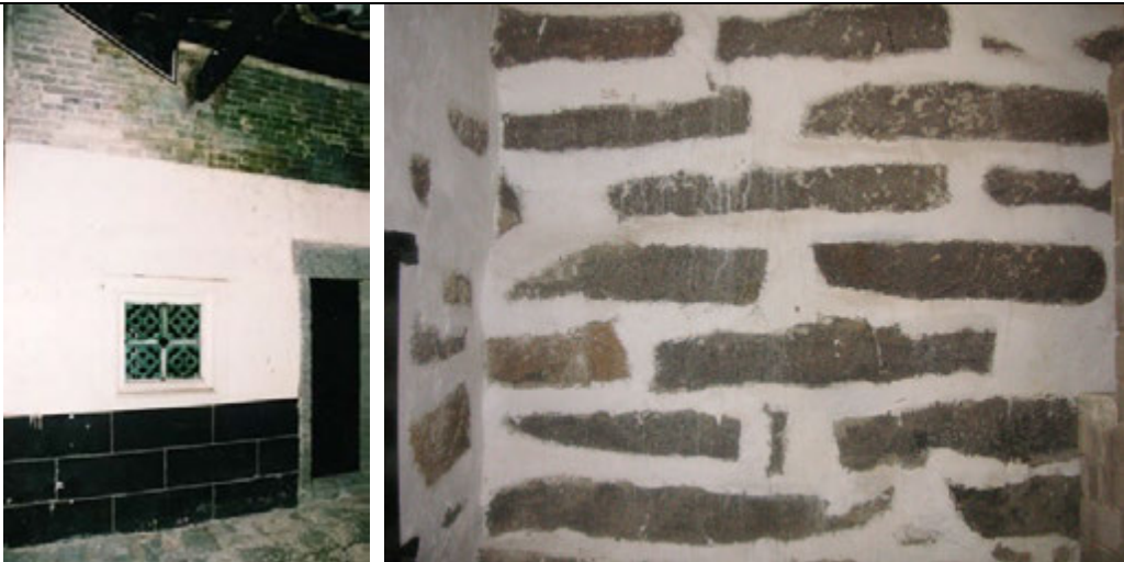
2.2) Wall finishes (some with stonework pattern), exposed granite blocks and brickworks
