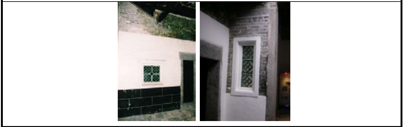
2.7) Ceramic grille-tiles and their surrounds at the open courtyard
