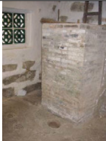
2.13) The partition wall and drain in the bathroom
