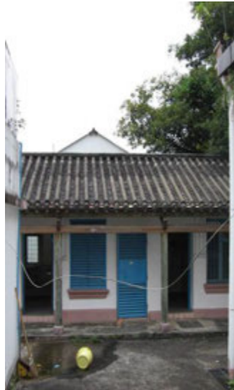
1.7) Verandah to Rear Wing of the Main Building
