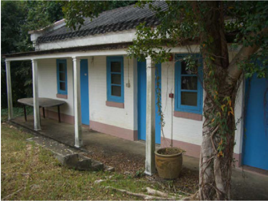
View of Staff Quarters Block
