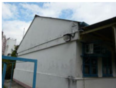
2.2) Painted external walls with brickwork texture
