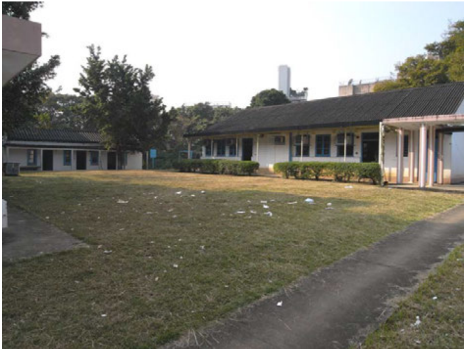
View of Canteen Block and Staff Quarters Block from open lawn
