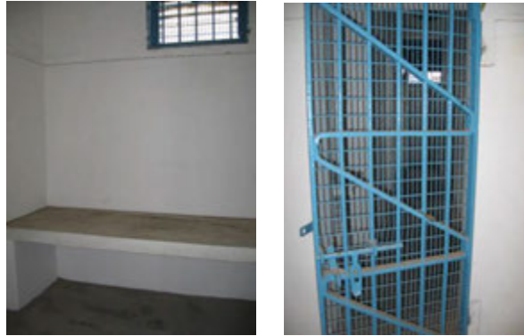
1.4) Cell Unit, which comprises two cells, security doors, toilet and corridor
