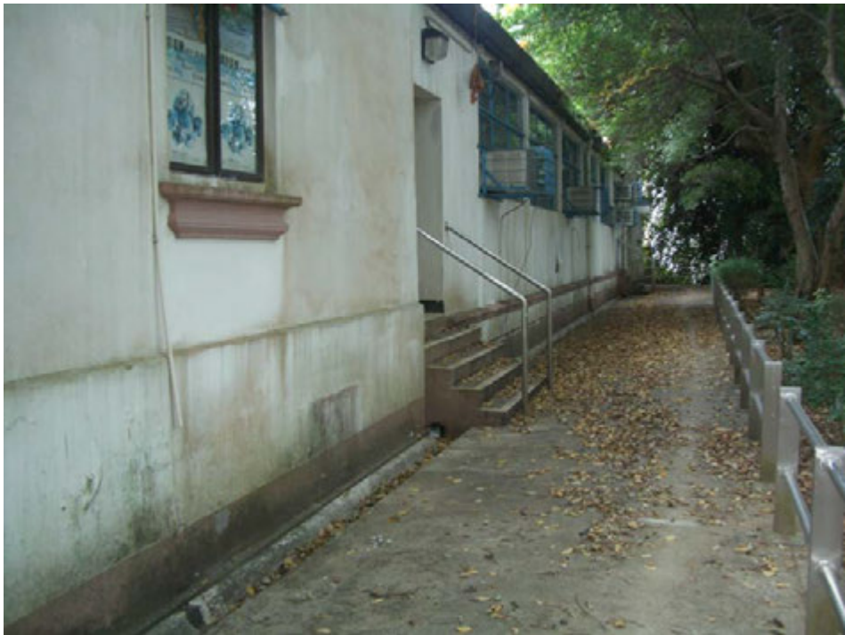
View of footway beside Main Building
