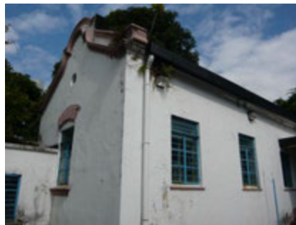
1.9) White coloured external plaster finish
