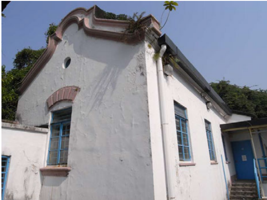
View of cat-arched gable wall at internal courtyard of Main Building
