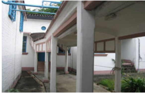
3.1) Covered walkway attached to the Main Building
