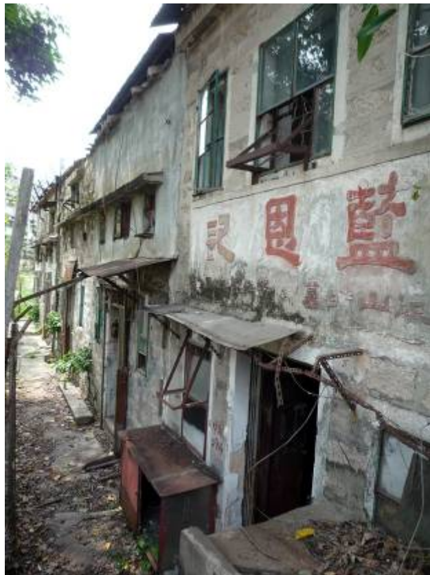
Front elevation of 31-35 Hau Wong Temple New Village
