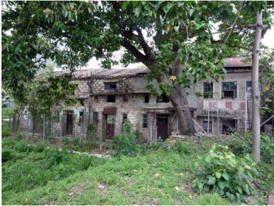
Front elevation of 31-35 Hau Wong Temple New Village
