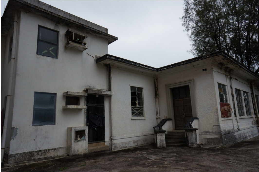
Entrances of the Watervale House
