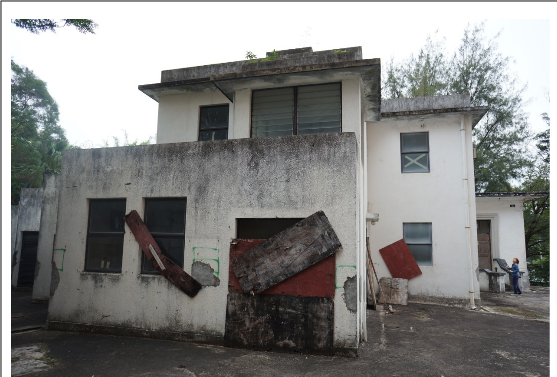
North elevation of the Extension
