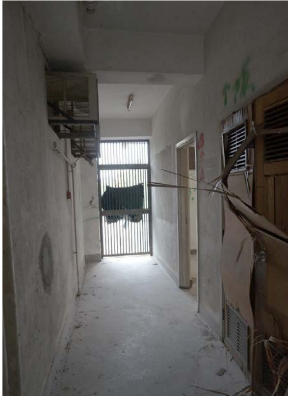
Corridor (Covered Area) between the Main Block and the Extension (G/F)
