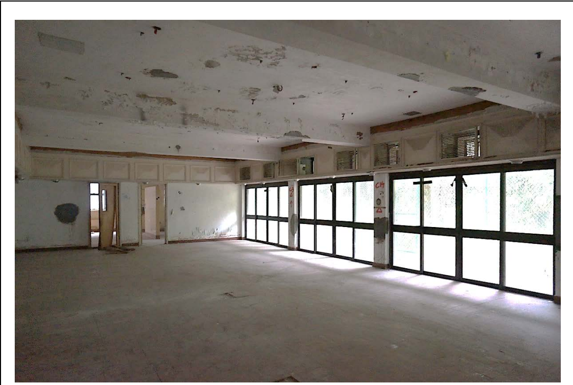
Dining Room of the Extension (G/F)
