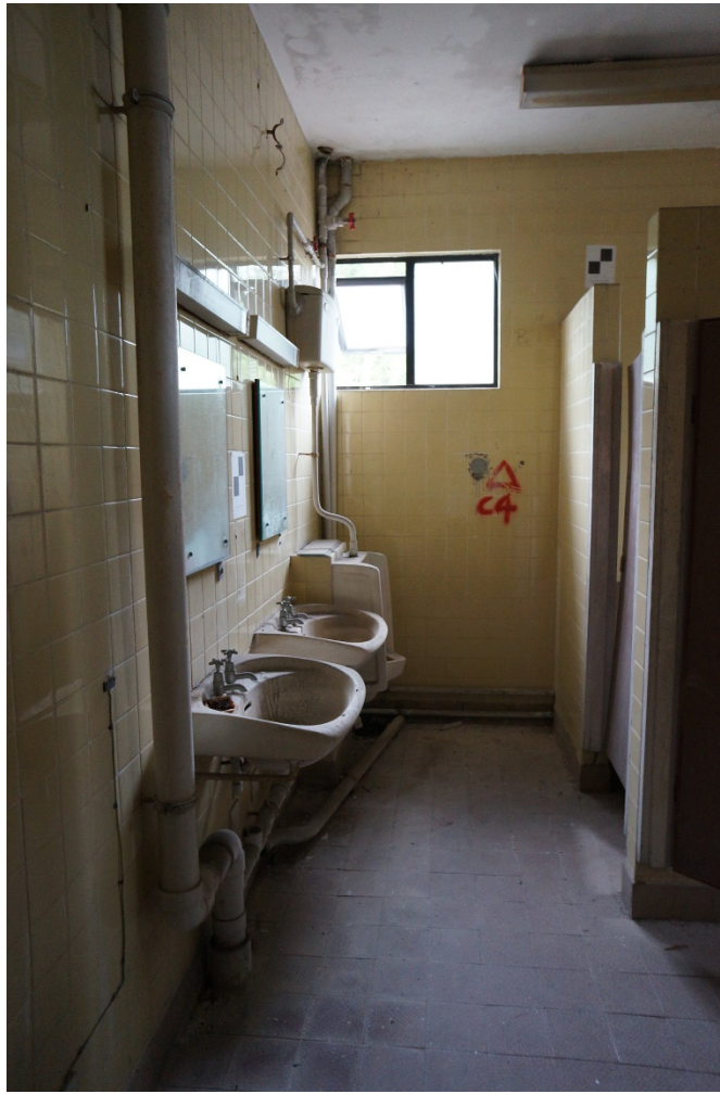
Bathroom of the Extension (1/F)
