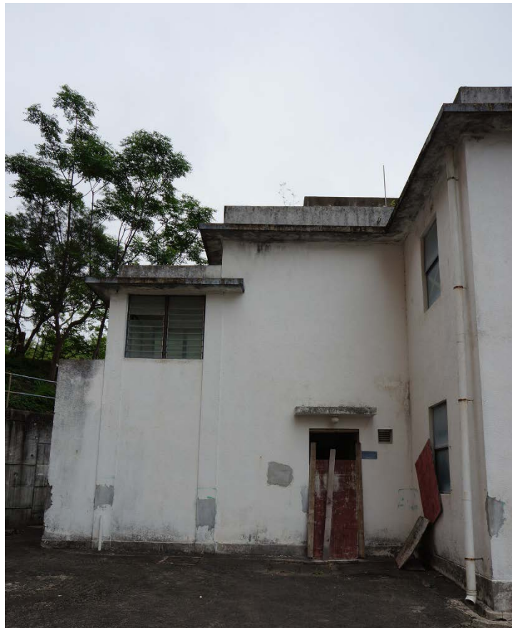
West elevation of the Extension
