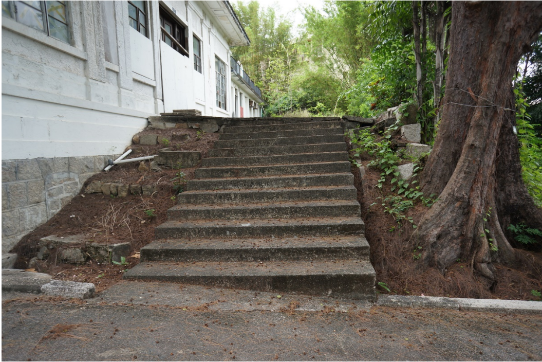
General view of approach staircase of South Entrance
