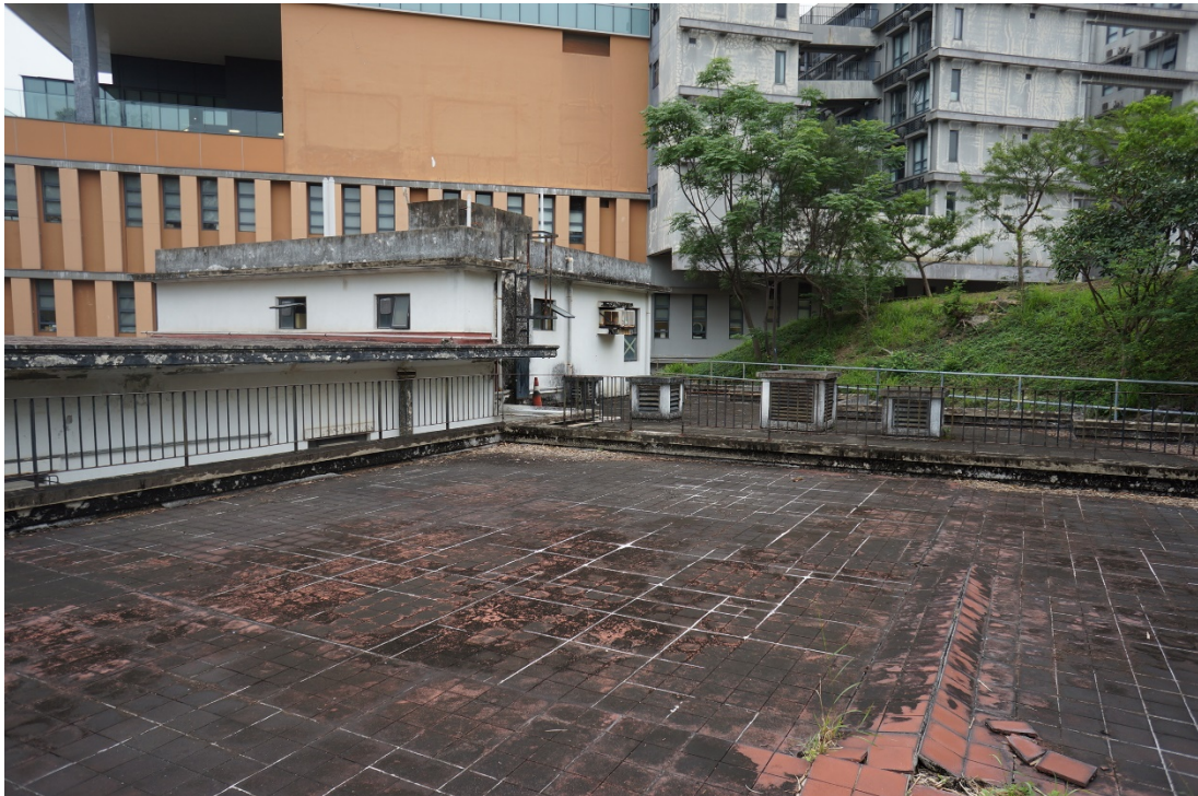
General view of the Roof of the Extension
