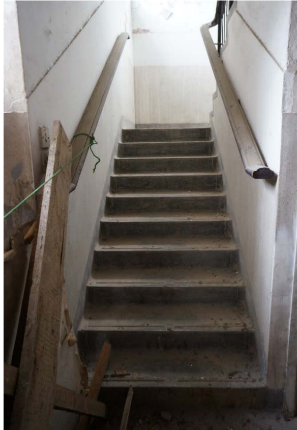
The staircase from G/F to 1/F of the Extension (G/F)
