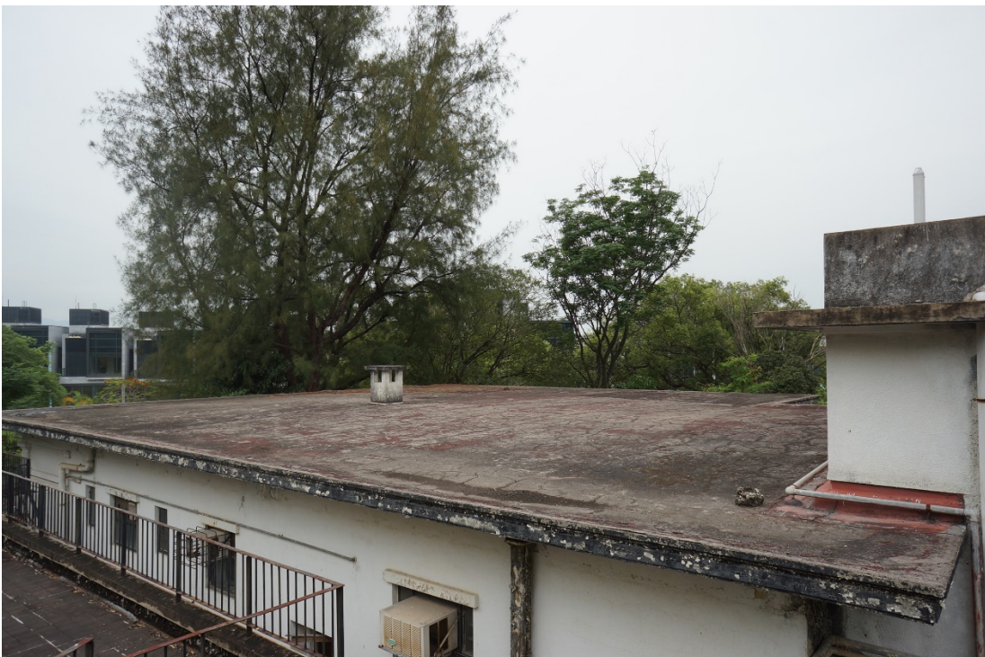
General view of the Roof of the Main Block
