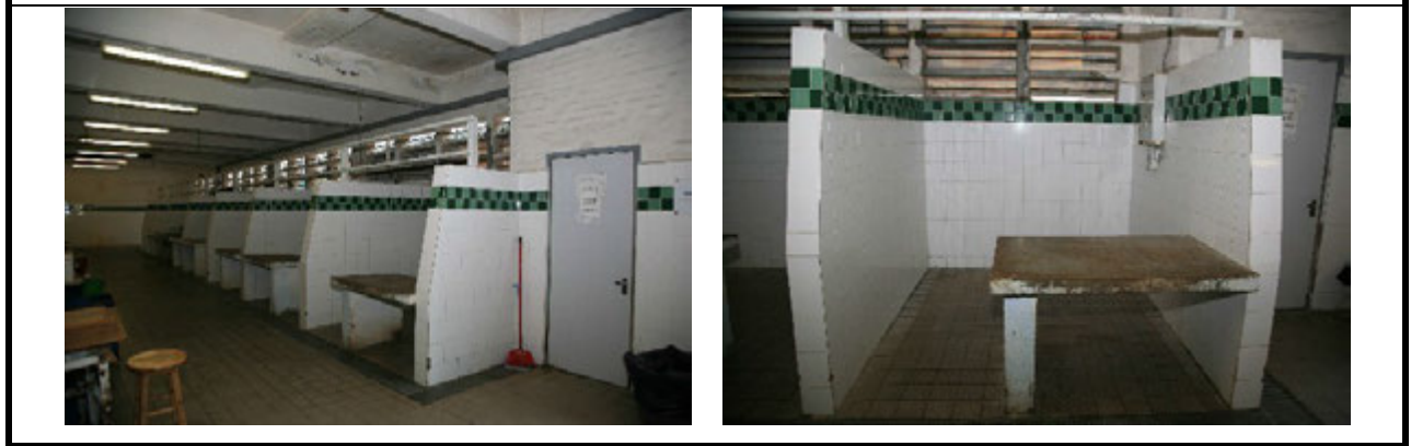
4.1) G/F open stalls cladded by tiles, comprising partition walls, concrete benches and parameter ditches
