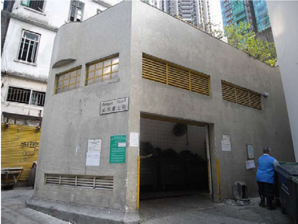
2.12 View of RCP
