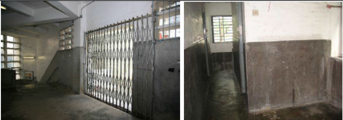
4.5) Shanghai plaster dado on internal walls
