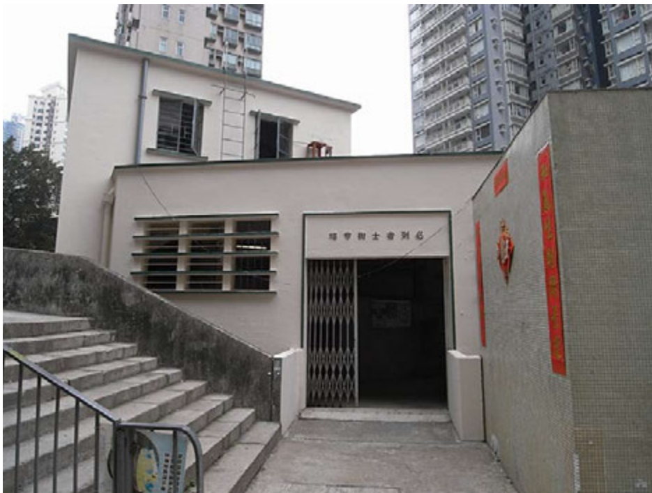
2.3 View of entrance to 1/F of Bridges Street Market from Shing Wong Street
