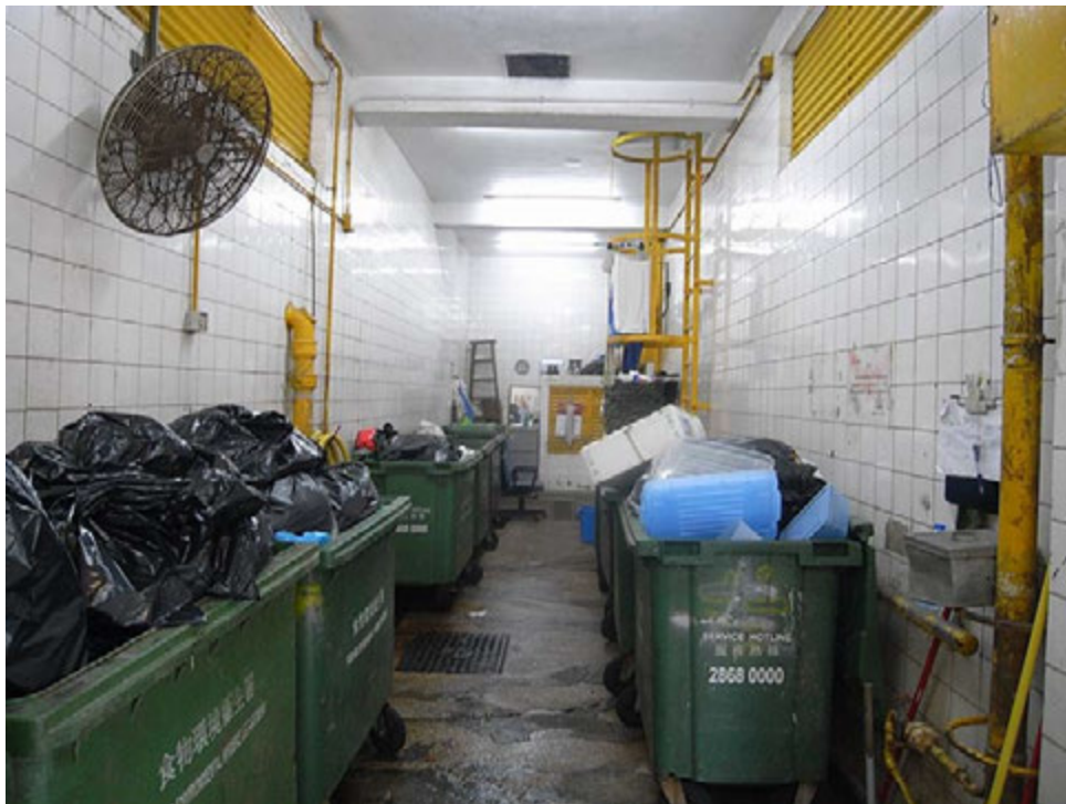
2.13 View of interior of RCP
