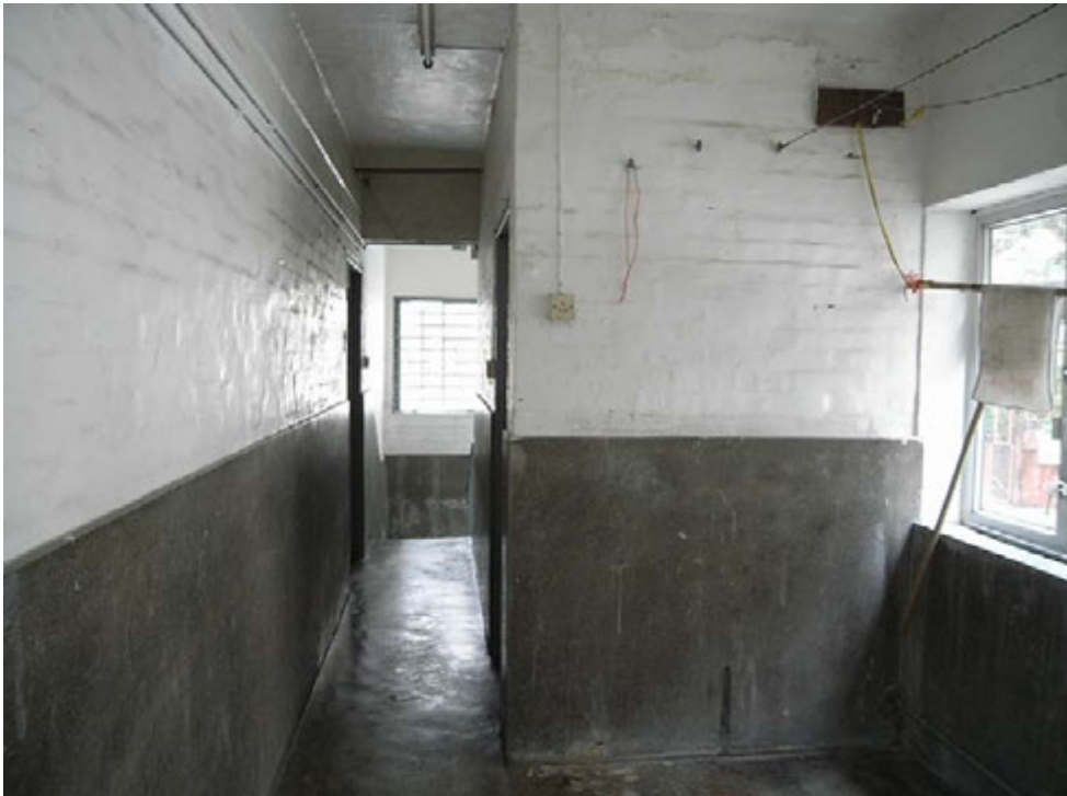
2.11 View of 2/F of Bridges Street Market
