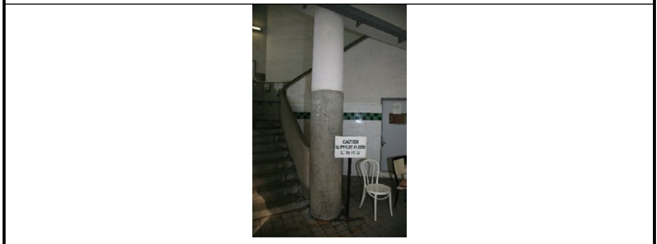
4.3) Round concrete columns with Shanghai plaster dado
