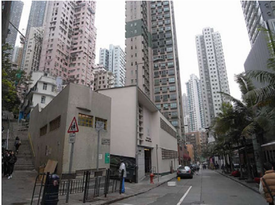
1.1 View of Bridges Street Market and RCP from Bridges Street
