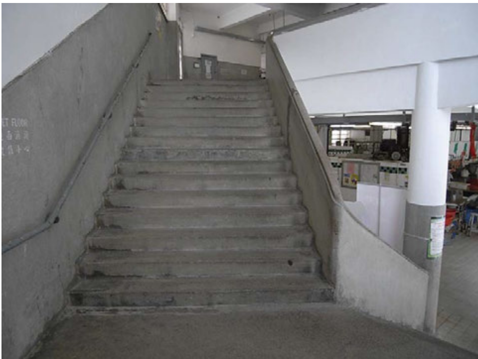
2.7 View of main staircase of Bridges Street Market
