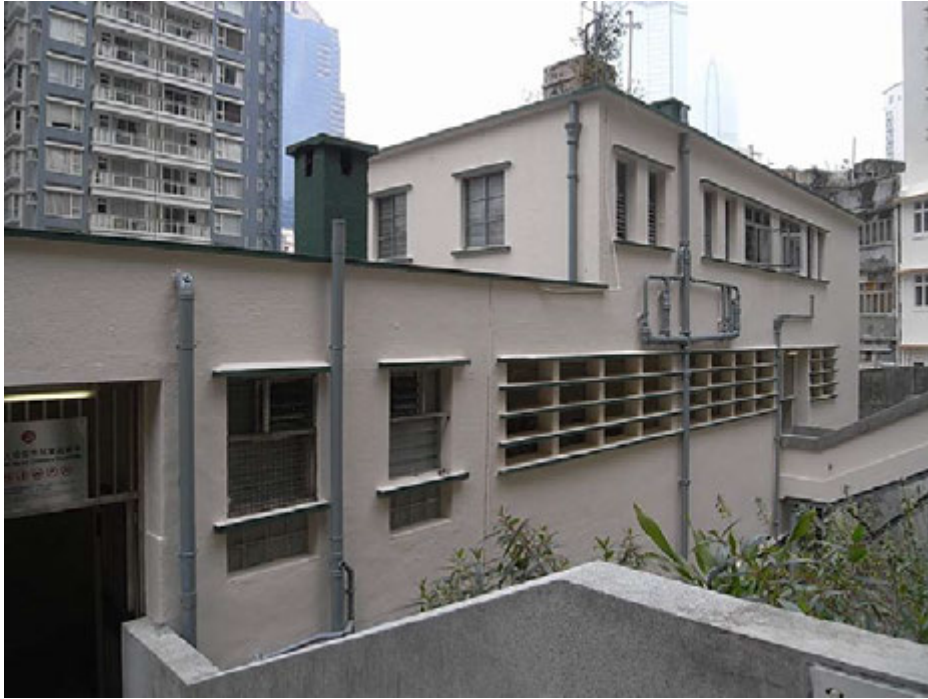
2.4 View of rear façade from Wing Lee Street
