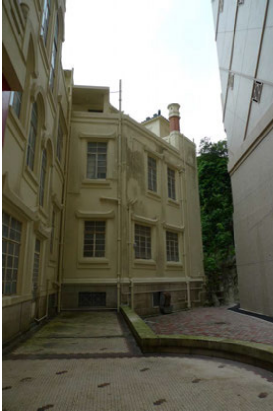
Elevation of the Servants' Quarters (Southeast Facade)
