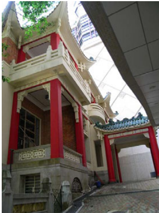
Side Elevation of the Main Block of the Mansion and Entrance Porch (Northwest Facade)
