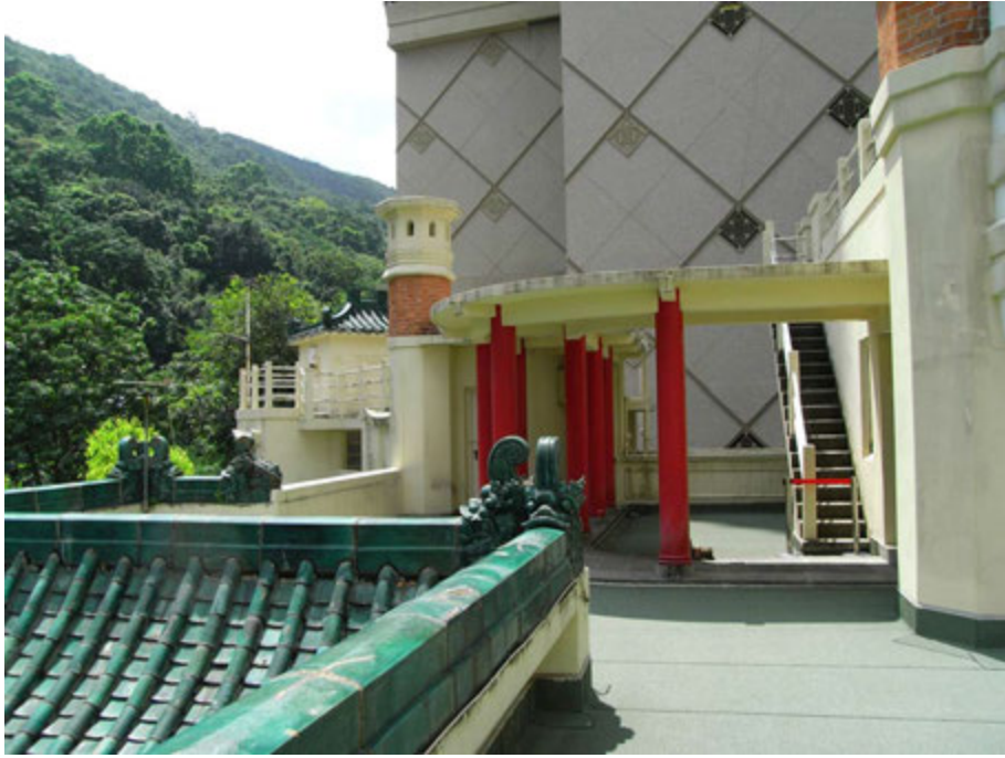
View of the Roof Terrace of the Mansion
