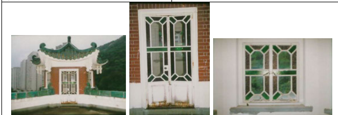
00317 1 glass door and 5 windows (at roof)
