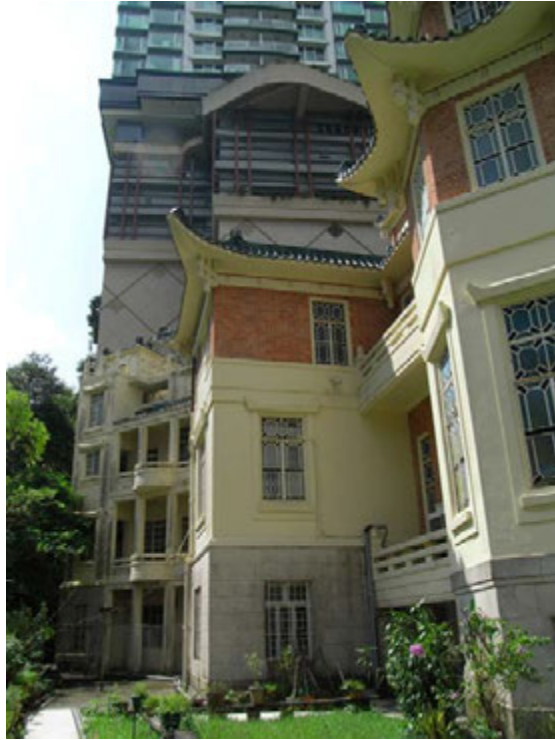
Side Elevation of the Main Block of the Mansion (Northeast Facade)
