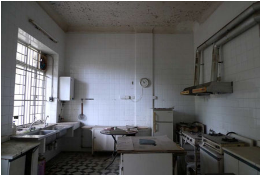
View of the Kitchen at the Lower Ground Floor of the Mansion
