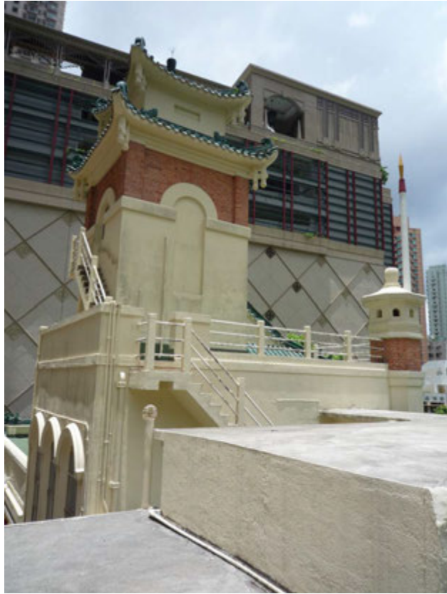
Tower with Water Tank on the Roof of the Mansion
