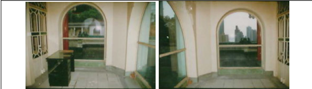
00319A-C Glass with frame (at Room T-3 at roof)
