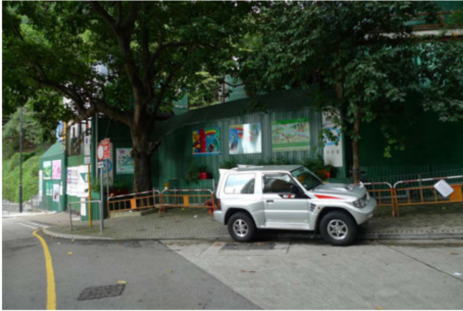
Ancillary Site Enclosed within Hoarding Viewed from Tai Hang Road
