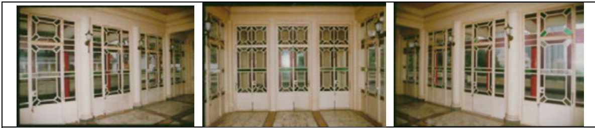
00318 Glass doors and windows (at Room T-2 at roof)
