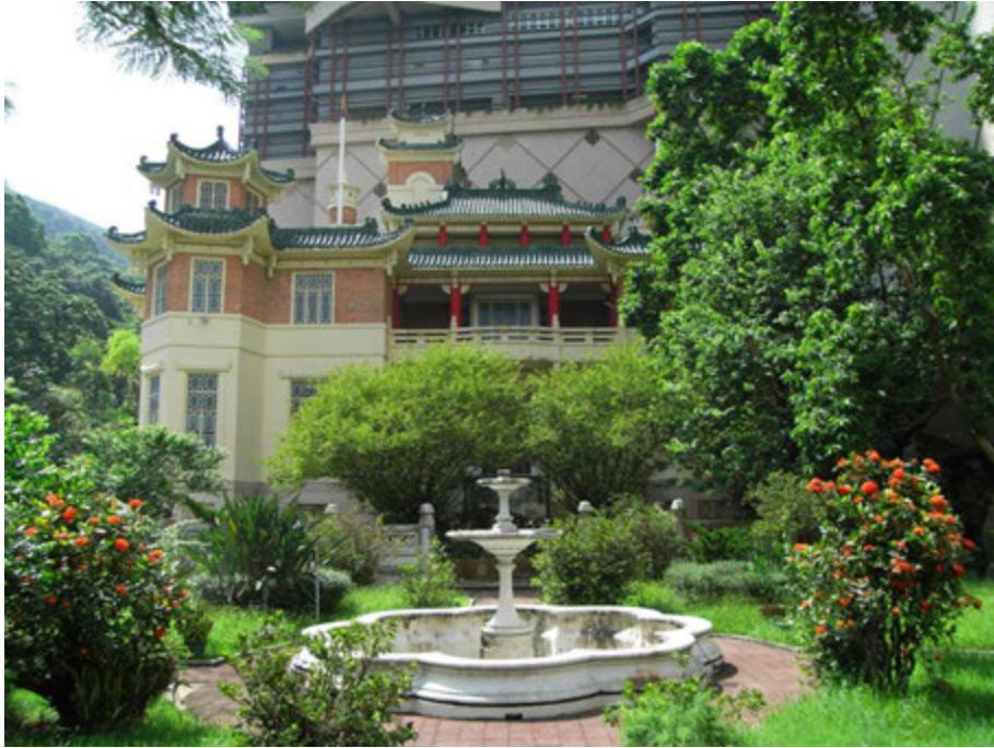
Elevation of the Mansion (Northwest Facade)
