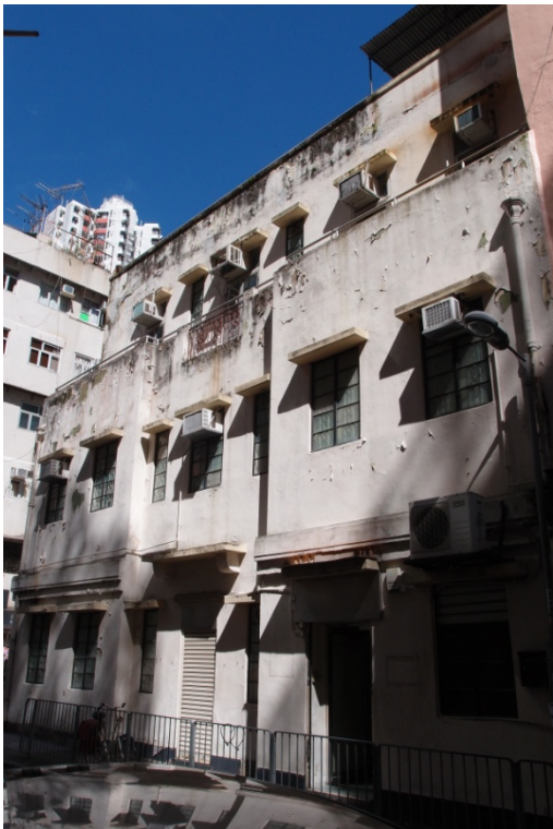
1.2 North west façade (Facing School Street)
