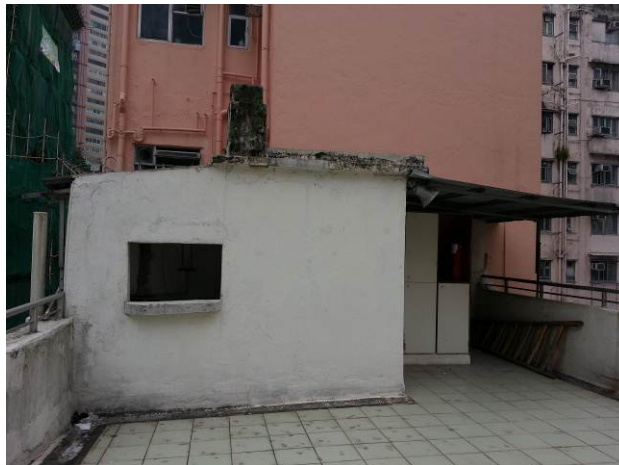
1.12) Staircase hood. (Kitchen and chimney are not original.)
