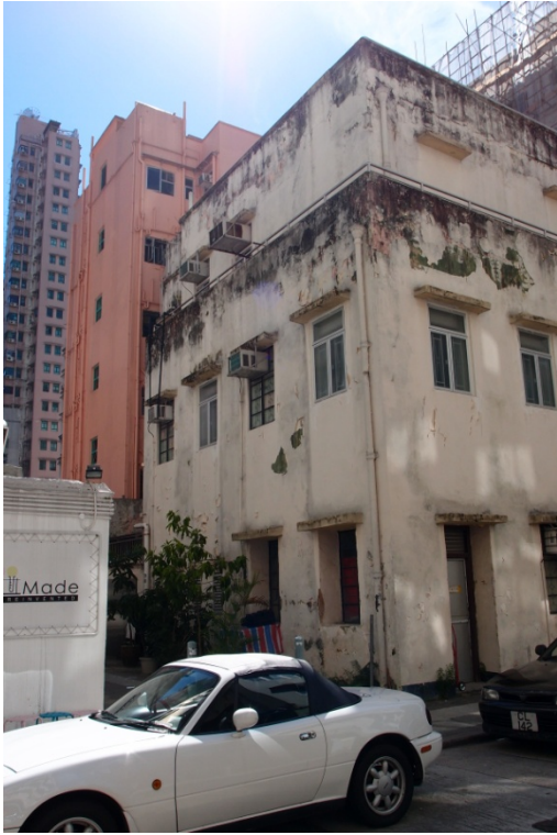
1.4 South east façade (Facing First Lane)
