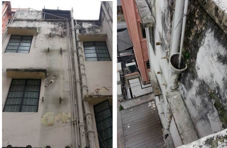
1.11) Ceramic rain water pipe with hopper head.
