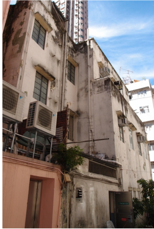
1.5 South east façade (Facing First Lane)
