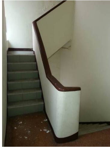
2.1) Staircase and continuous balustrade leading from G/F to R/F.
