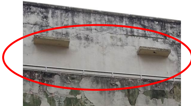
Door openings to open corridor facing Brown Street are being blocked
