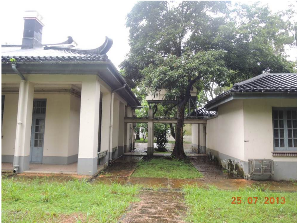
4.1 Covered walkway connecting the Main Block and the Bungalow
