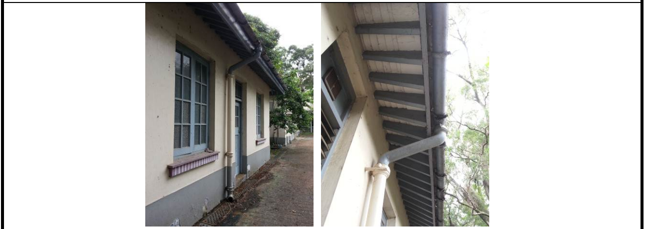
2.12) Cast iron rainwater pipes and eave gutters at the elevations.
