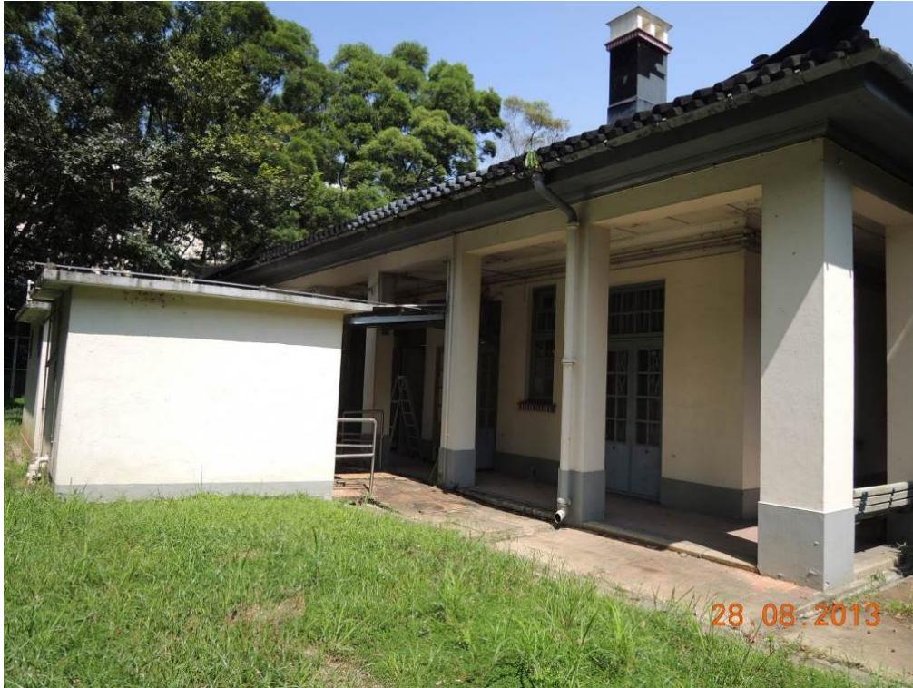
2.4 Rear elevation of Main Block facing Kwu Tung Road
