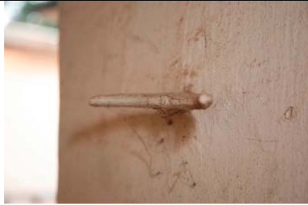
1.19) Cow's horn cleats mounted on the verandah columns.
