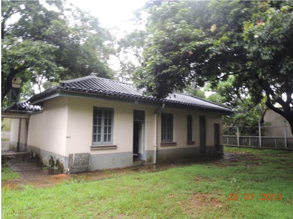
3.4 Rear elevation of Bungalow facing Kwu Tung Road
