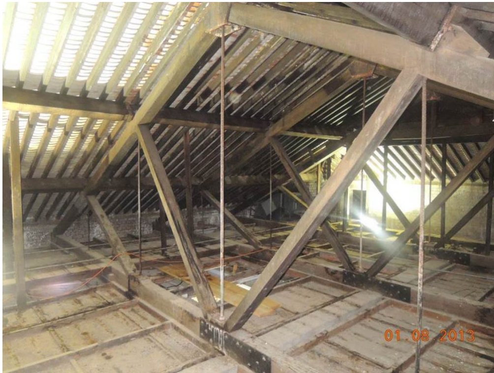
2.6 Roof truss structure at Main Block
