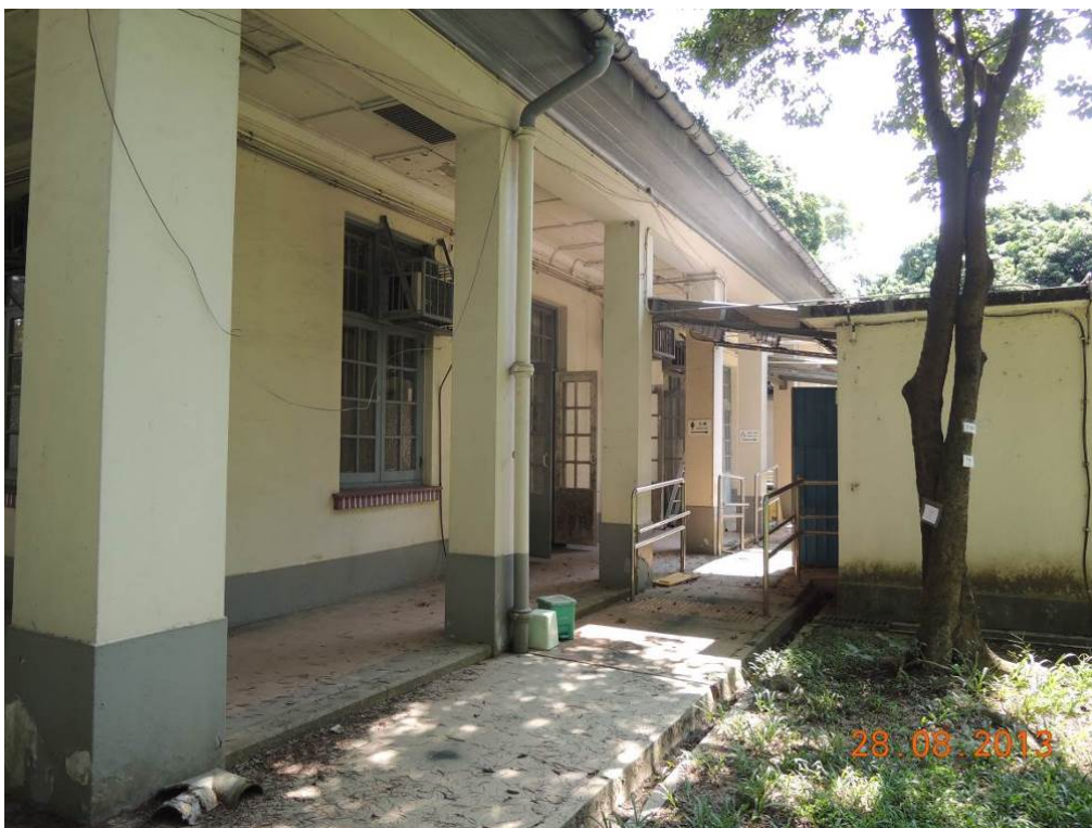
2.3 Rear elevation of Main Block facing Kwu Tung Road
