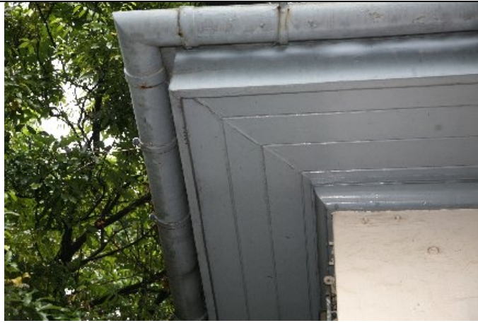
1.8) Over-hanging roof eaves with suspended timber battened ceiling
