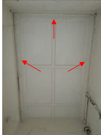
View to ceiling
