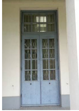
External door to verandah with horizontal pivoted windows
