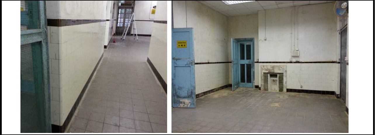
1.11) Original glazed wall tiles in the Waiting Hall and Treatment Room.
