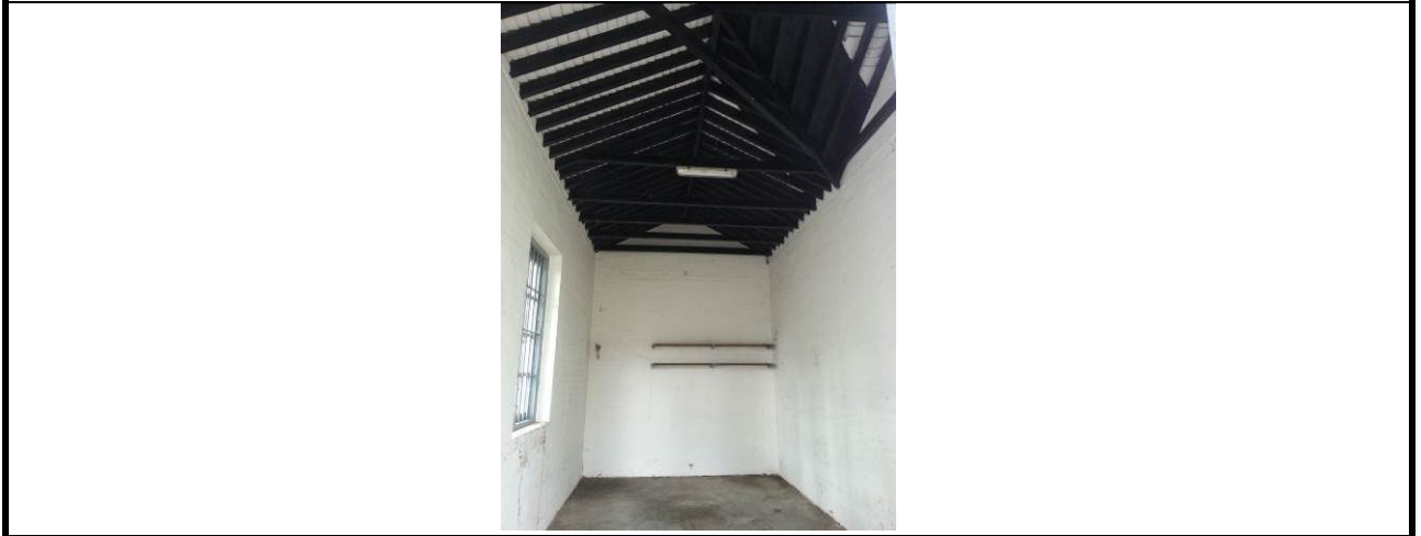
2.11) Internal space of the Garage.
