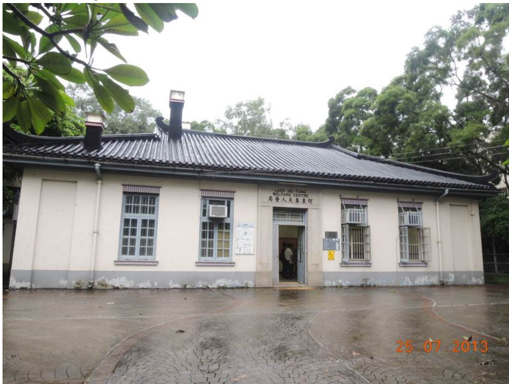
2.1 Front elevation of the Main Block facing main entrance
