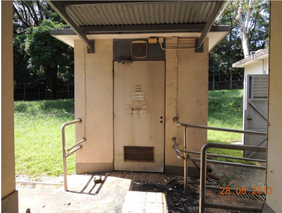
5.2 Disabled toilet facing the Main Block
