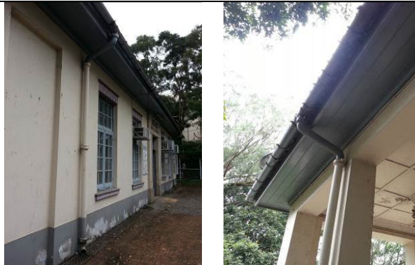
1.20) Cast iron rainwater pipes and eave gutters at the elevations.
