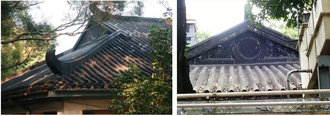
1.7) Chinese style roof with hip and gable roof structure, including curled-up ends of roof ridges and circular decorative moulding on pediment.
