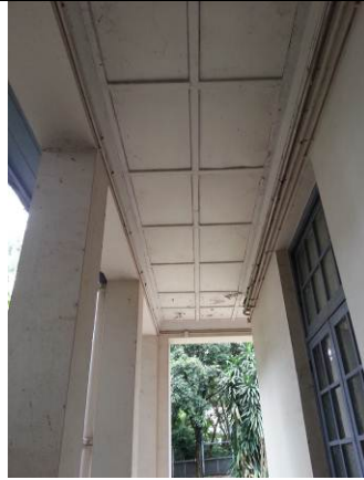
1.18) Timber suspended ceiling along the colonnaded verandah.
