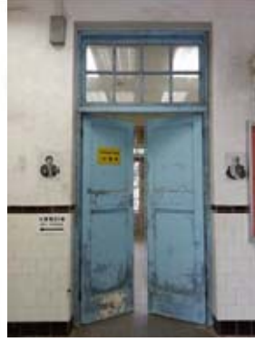
Internal door to Treatment Room
