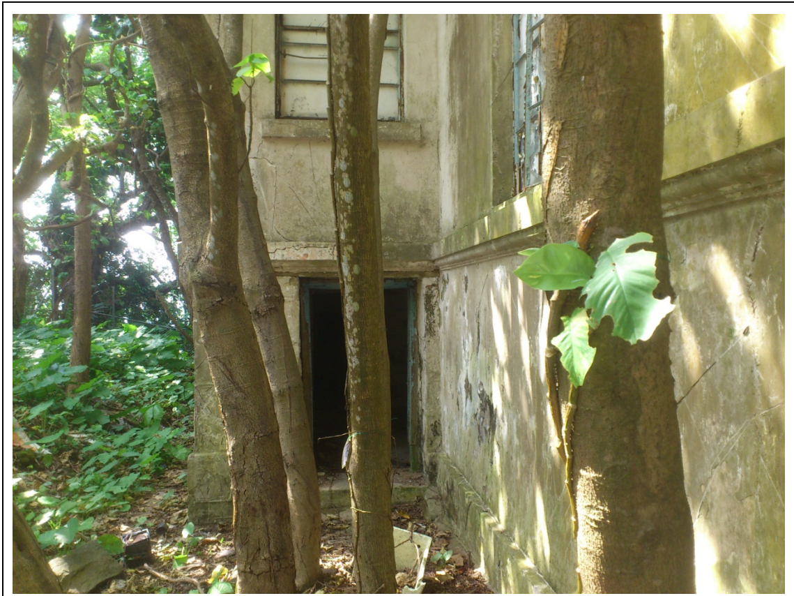
Entrance to G/F of the Main Building
