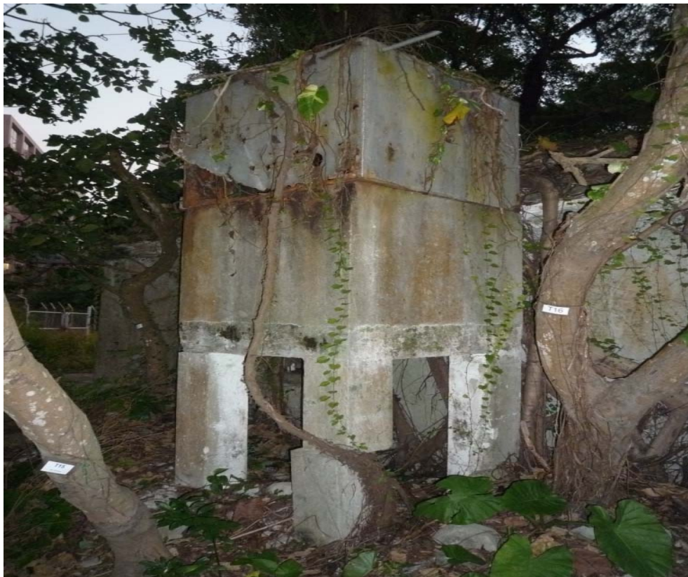
View of the water tank
