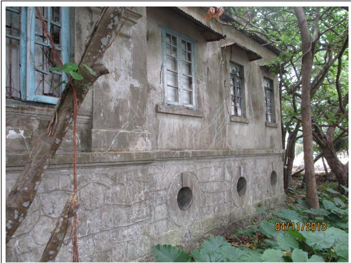
Side elevation of the Main Building
