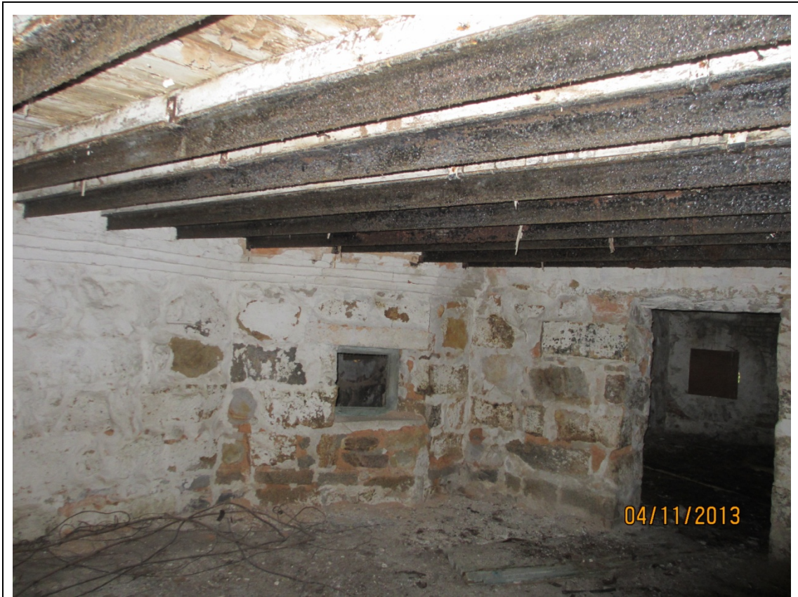
View of the G/F of the Main Building
