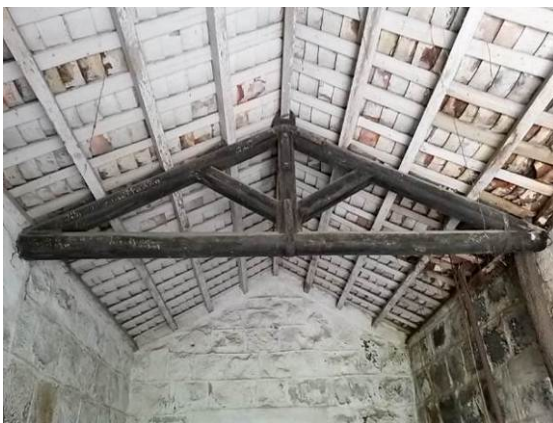
Roof of the Garage Block
