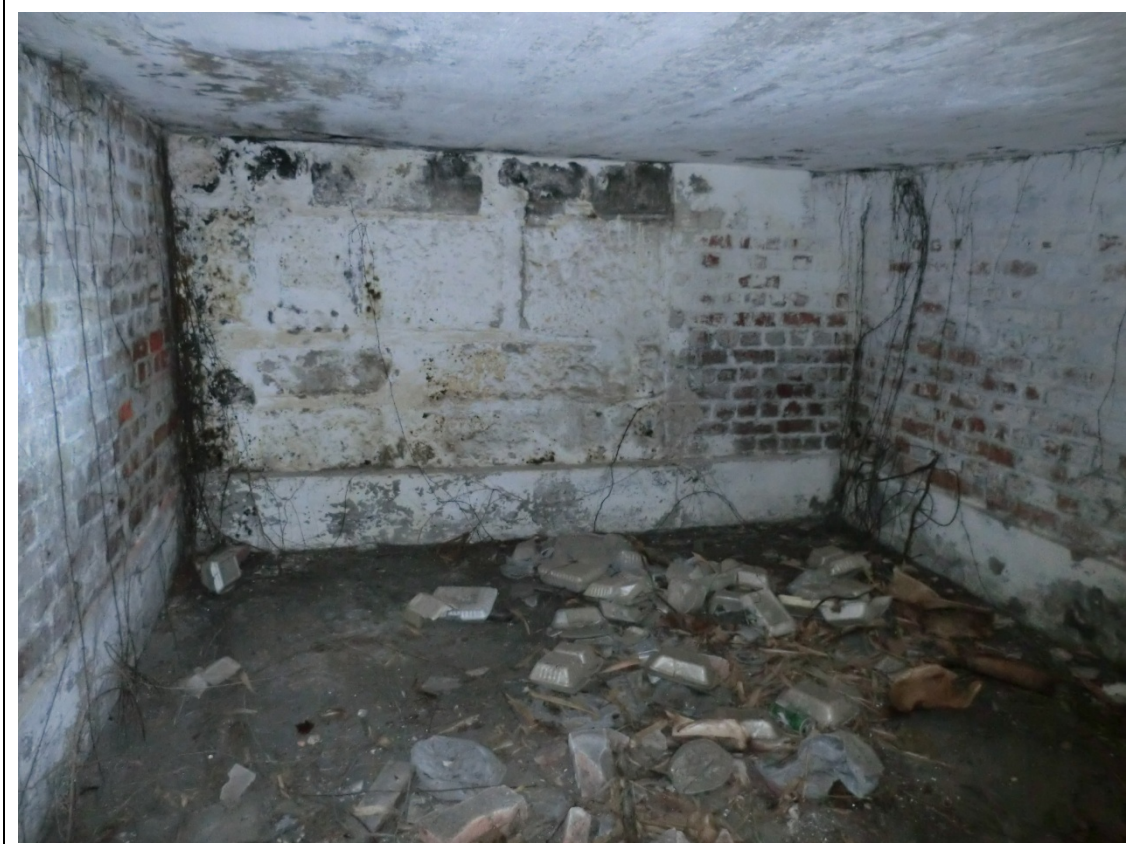
View of the usable space of the Main Building
