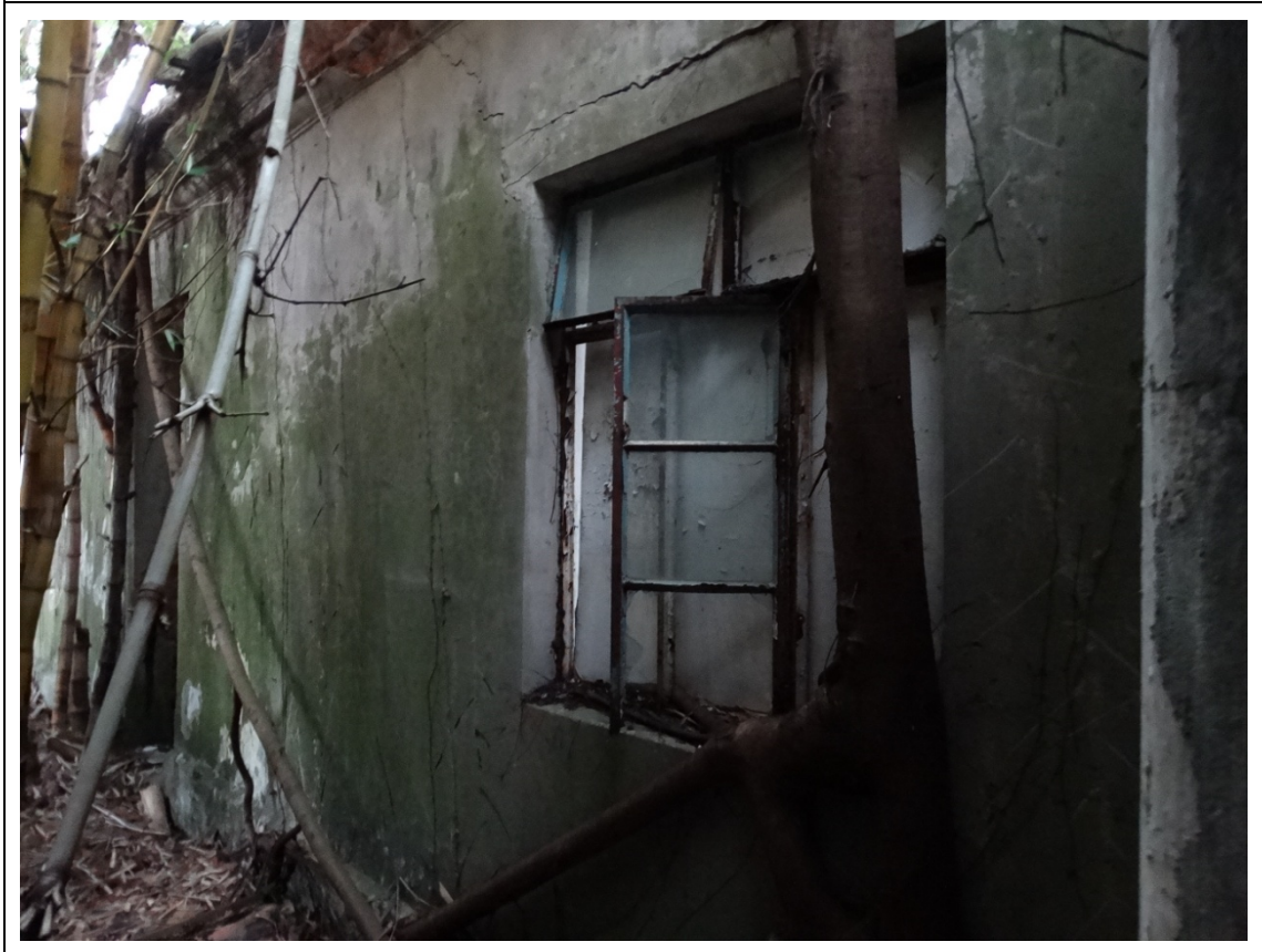
Elevation of the Servants' Quarters
