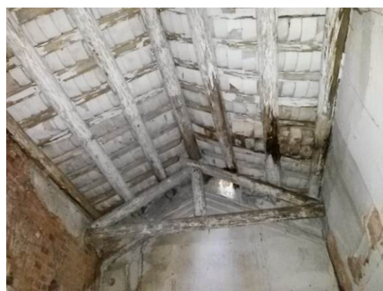
Roof of the Servants' Quarters
