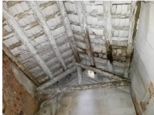
Roof of the Servants' Quarters
