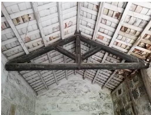
Roof of the Garage Block
