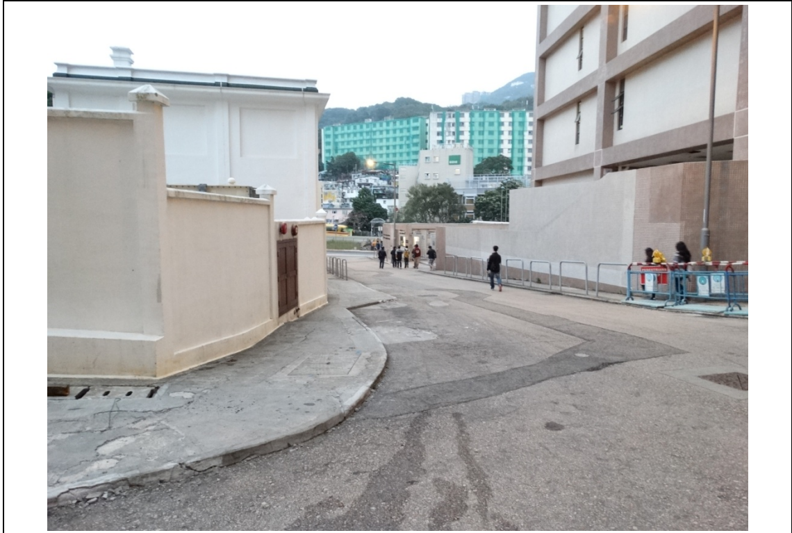
An access road connecting the Site to Pok Fu Lam Road (currently managed by the VTC)
