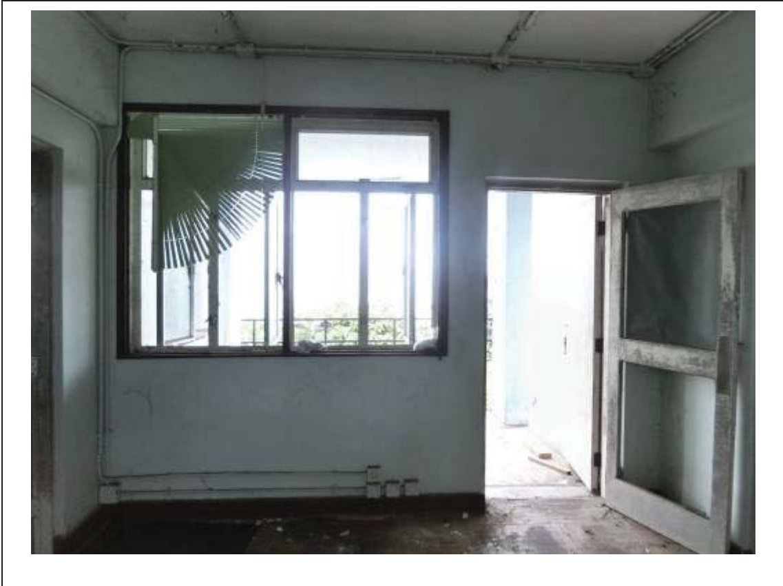
General view of the General Office
