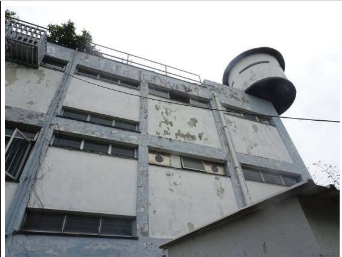
Rear elevation of Main Block
