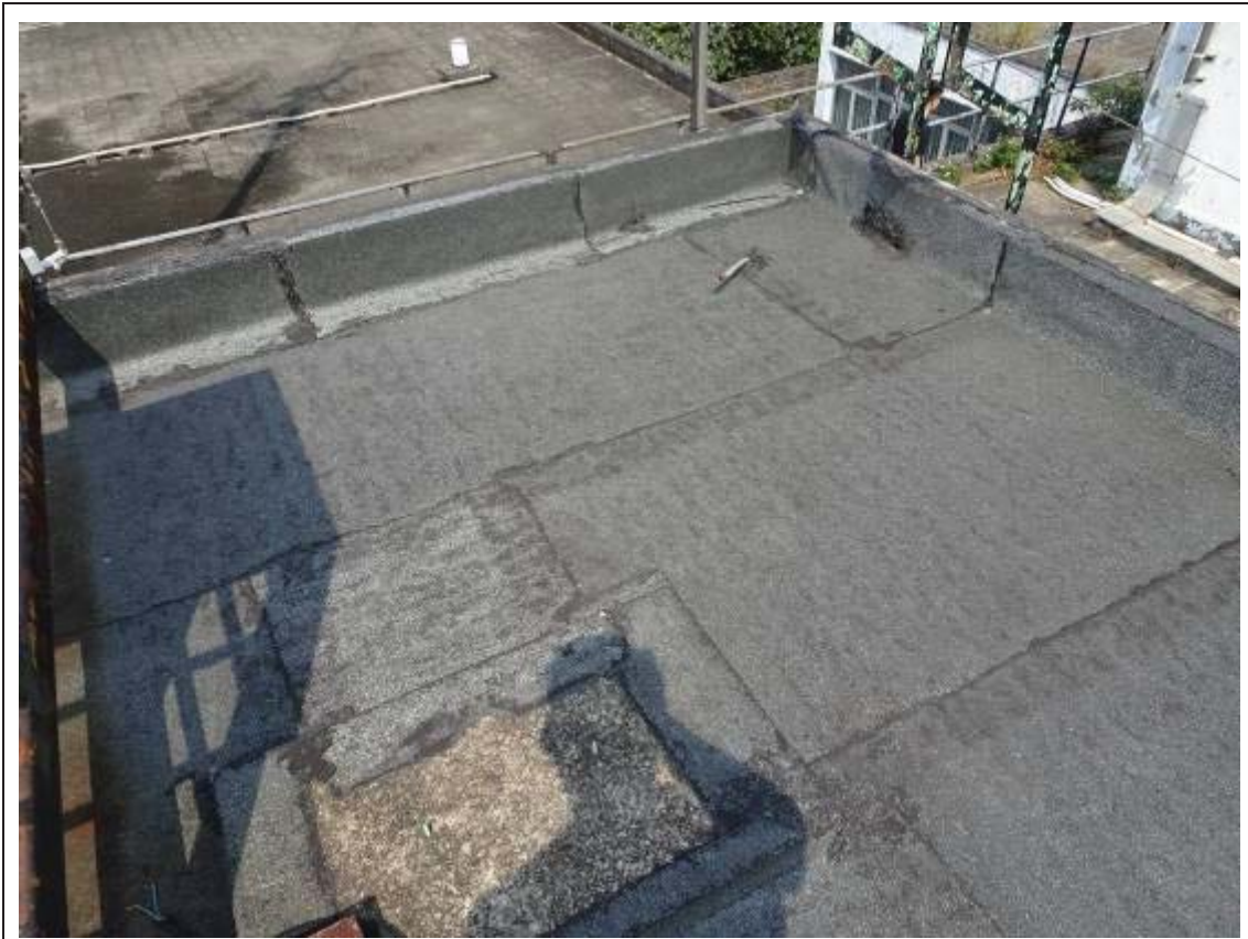
General view of the Upper Roof
