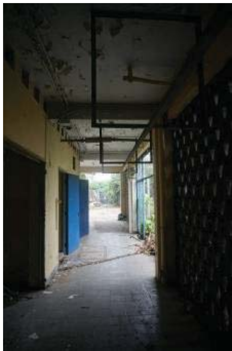
General view of the corridor at LG/F
