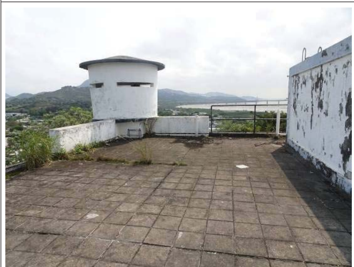
General view of the Main Roof
