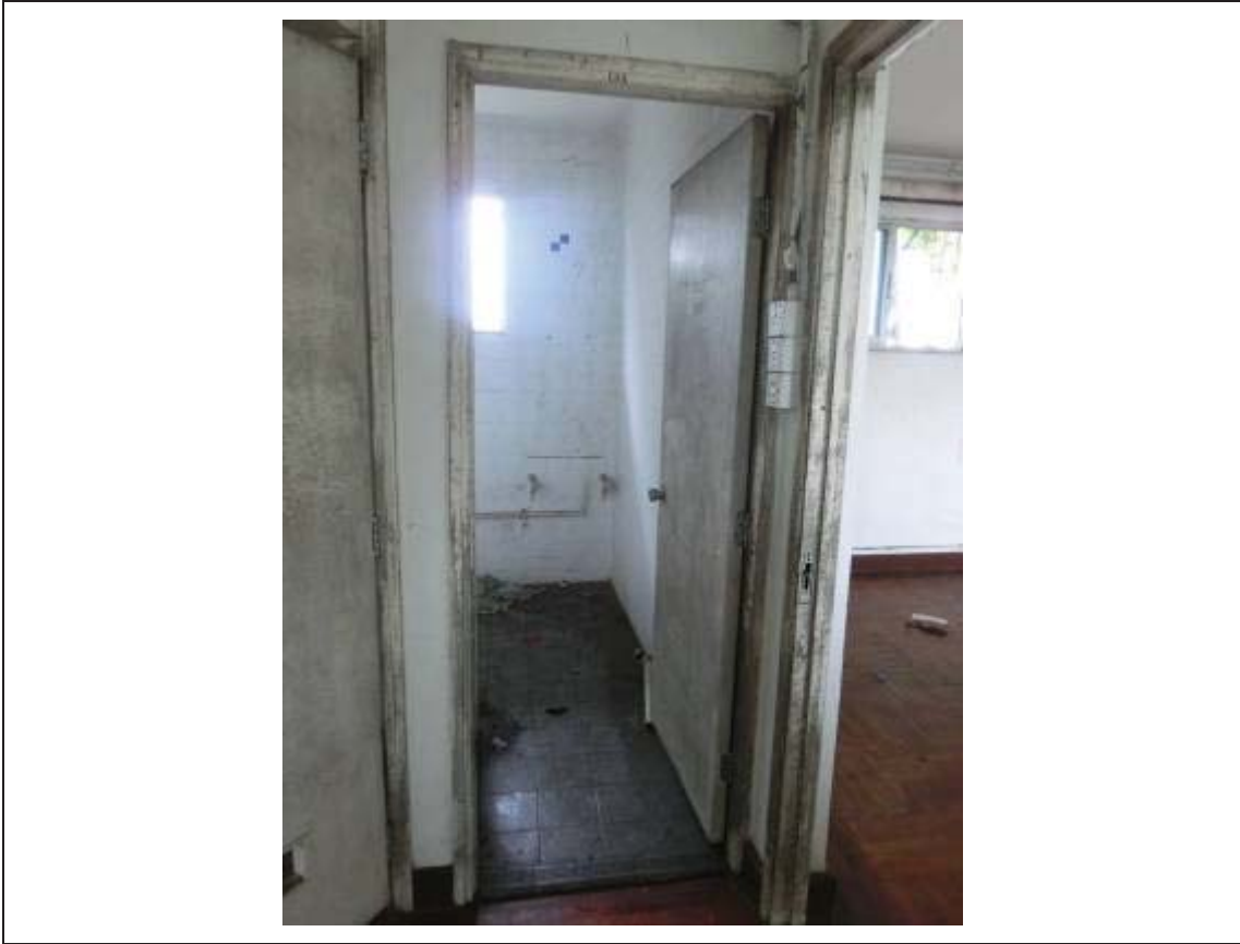
General view of the Toilet 2
