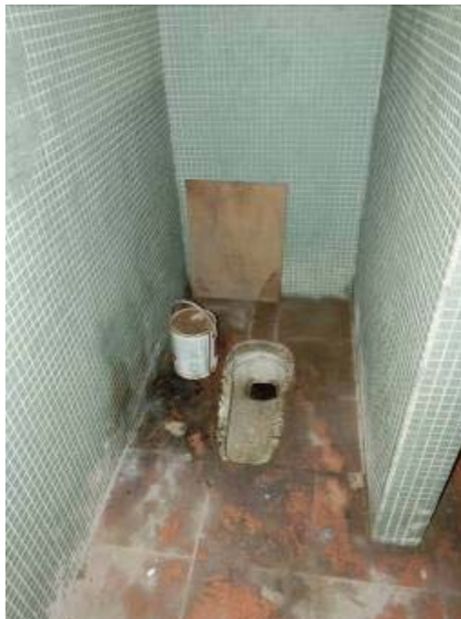
General view of the Cell Room
