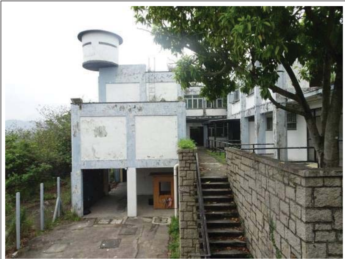
Front elevation of Main Block
