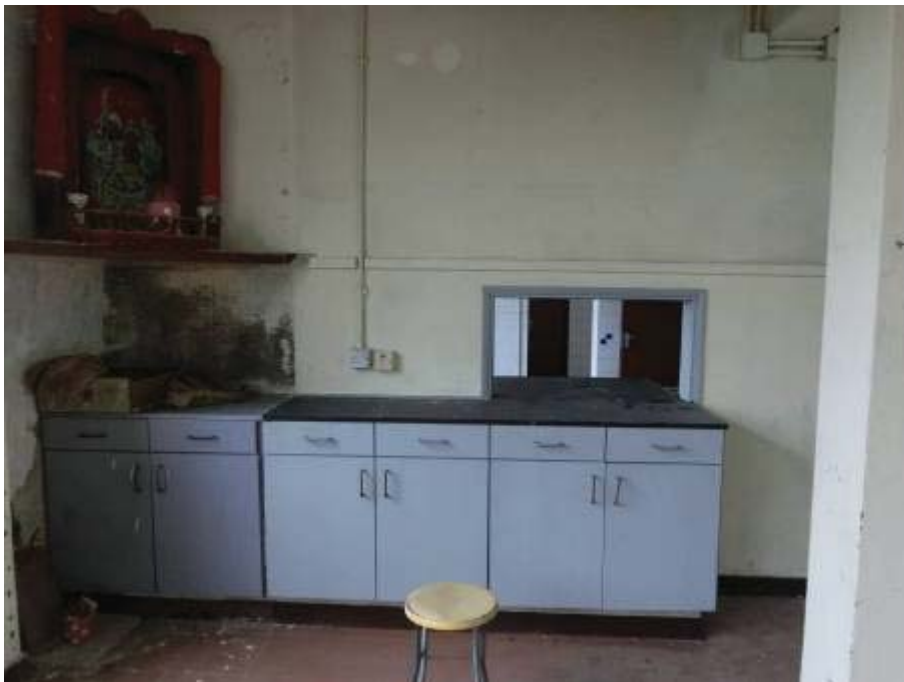
General view of the Mess Room and Recreation Room
