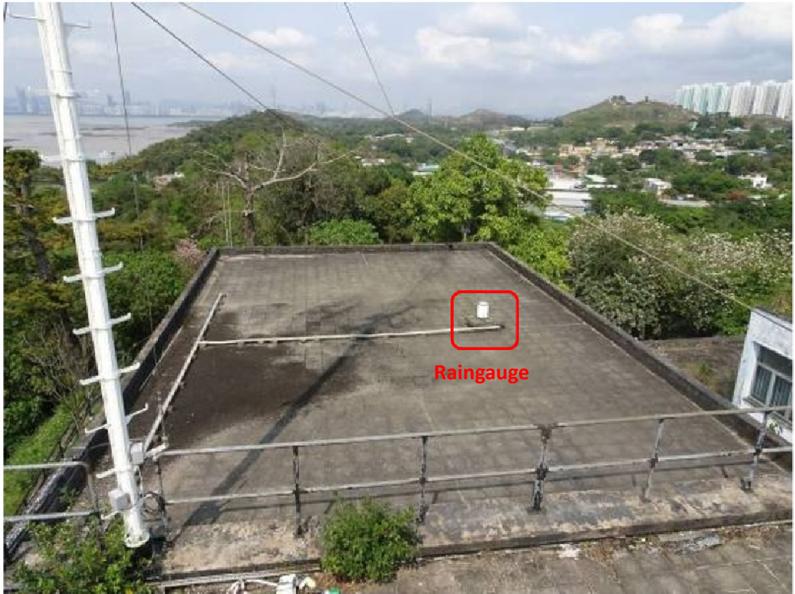
General view of the Main Roof and location of HKO's raingauge
