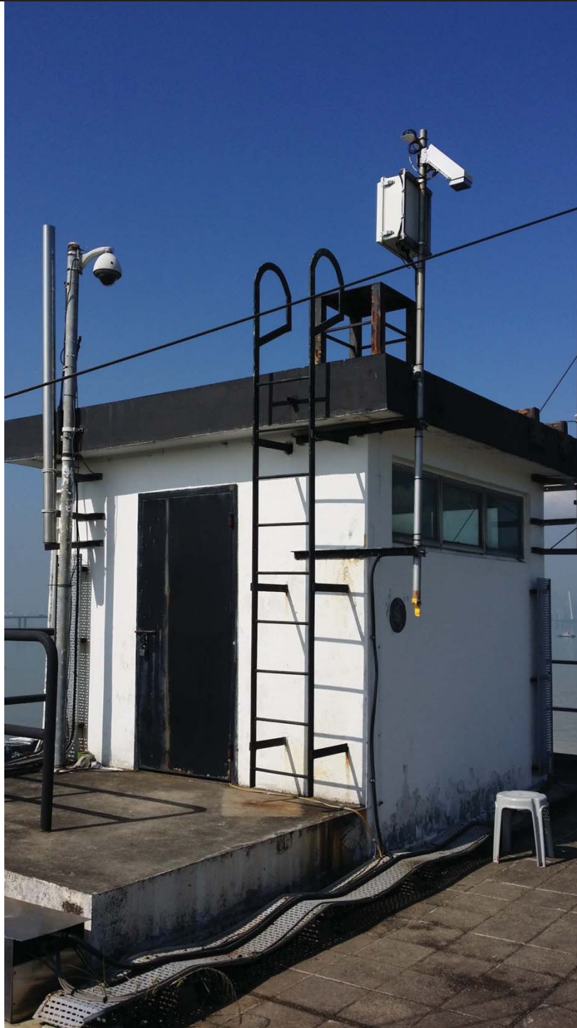
Existing HKO's instrument (lightning sensor) on Roof
