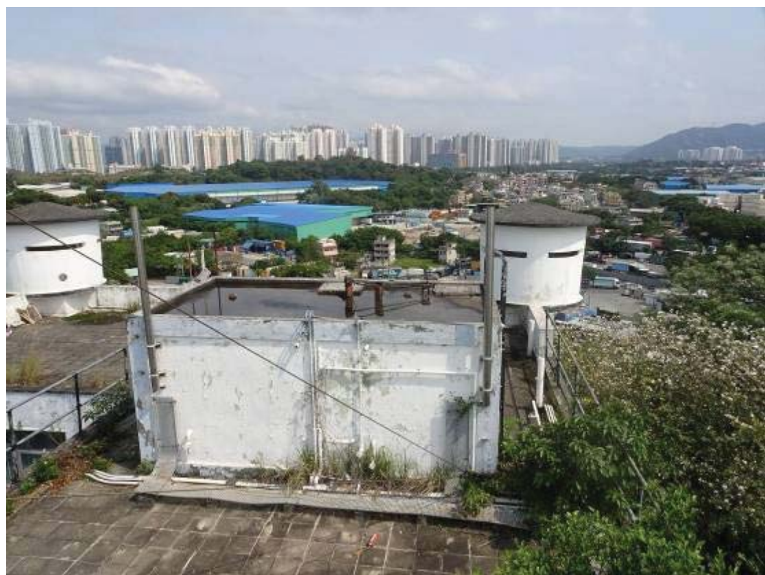
General view of the roof of Water Tank and Scout Towers
