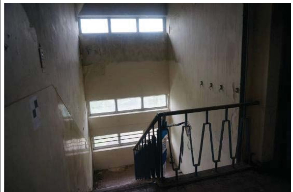
General View of staircase at 1/F
