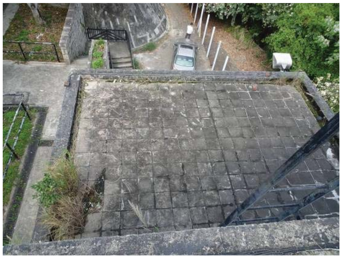
General view of the Flat Roof at 1/F of Main Block
