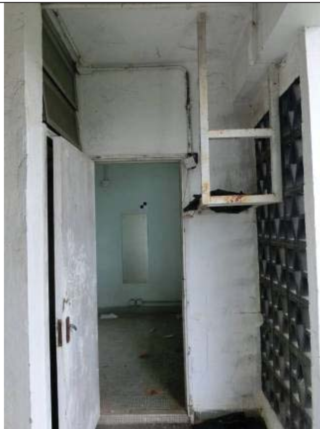
General view of the Female Barrack Room main door
