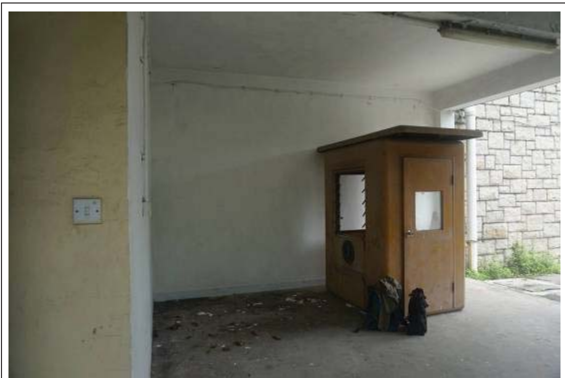
General view of Covered Parking Space at LG/F
