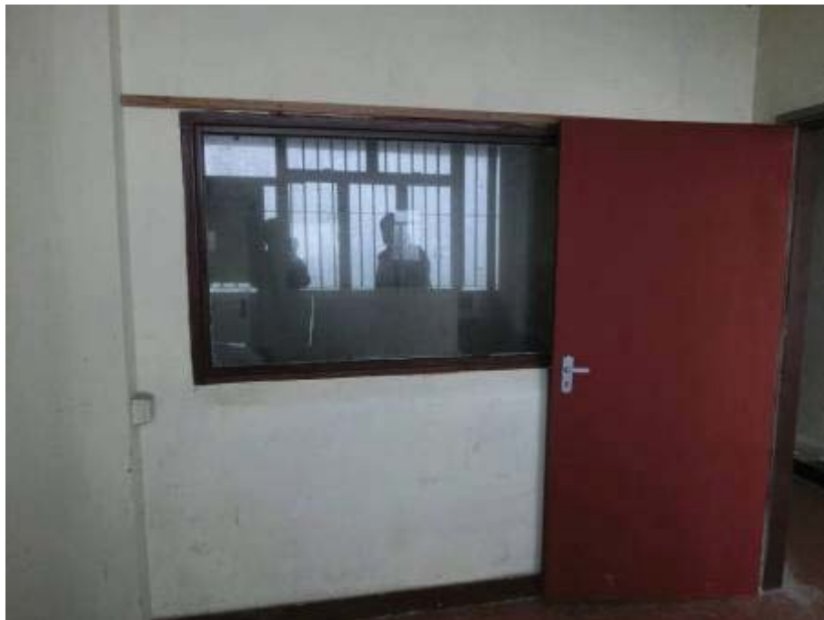
General view of the corridor
