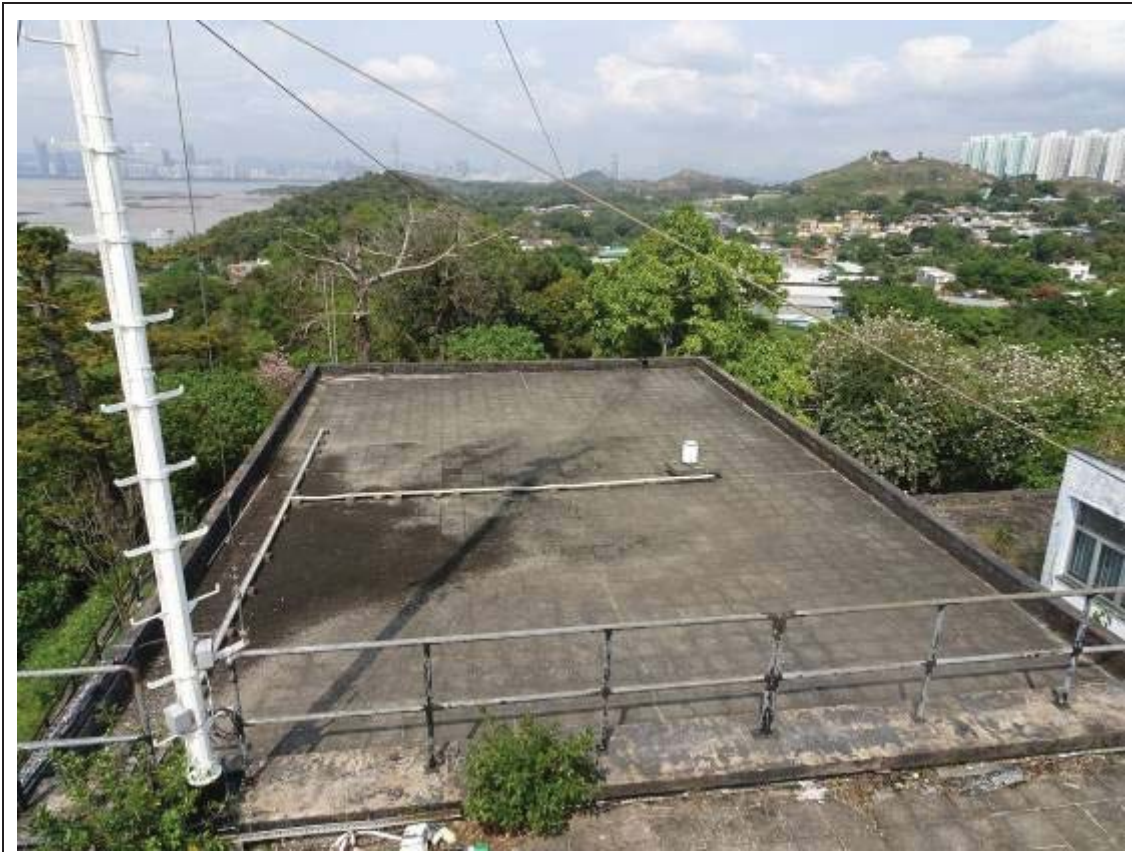
General view of the Main Roof
