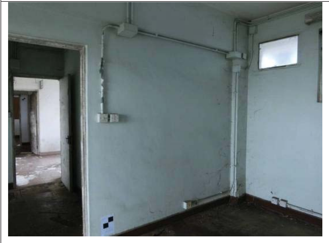
General view of the General Office
