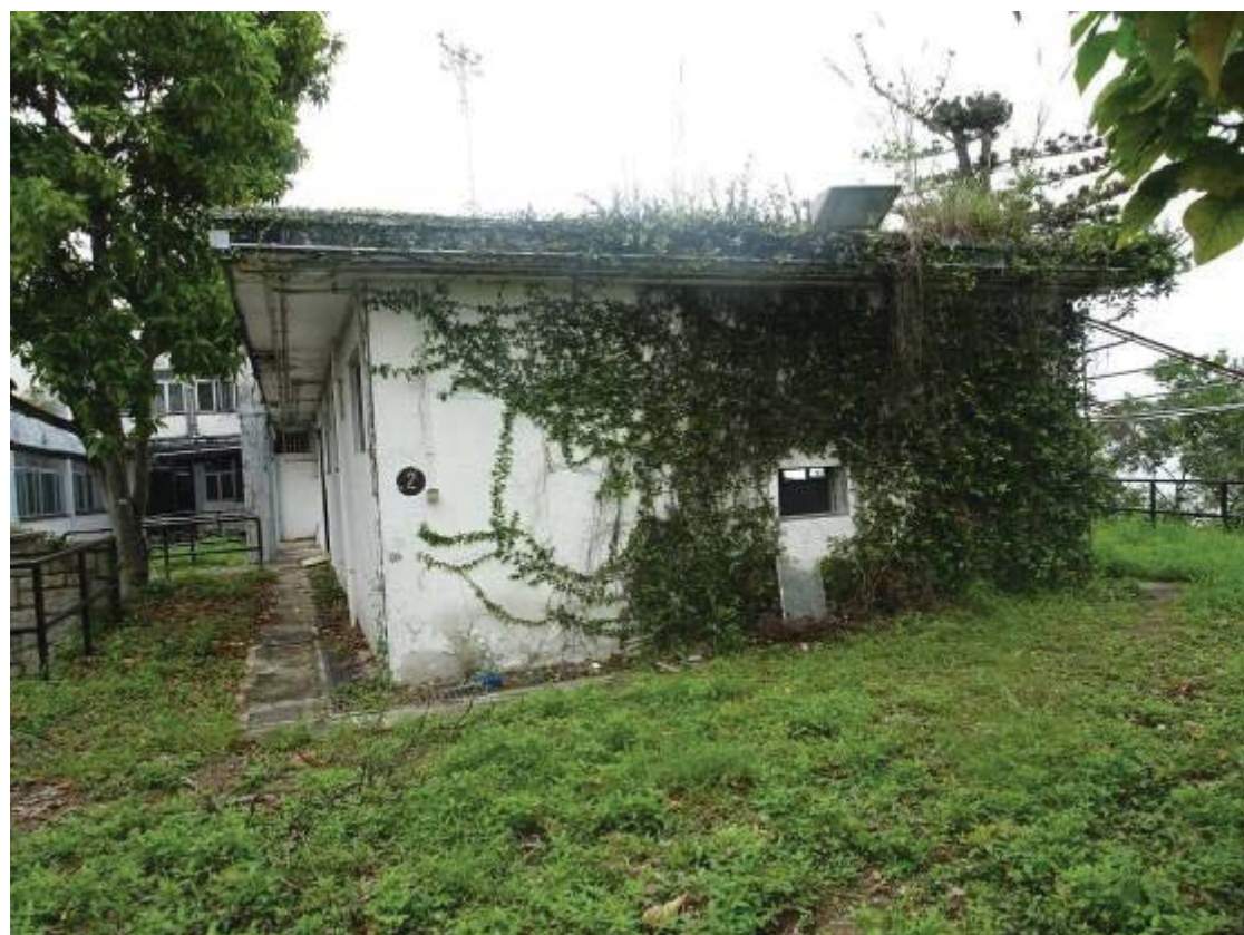
Front elevation of Main Block
