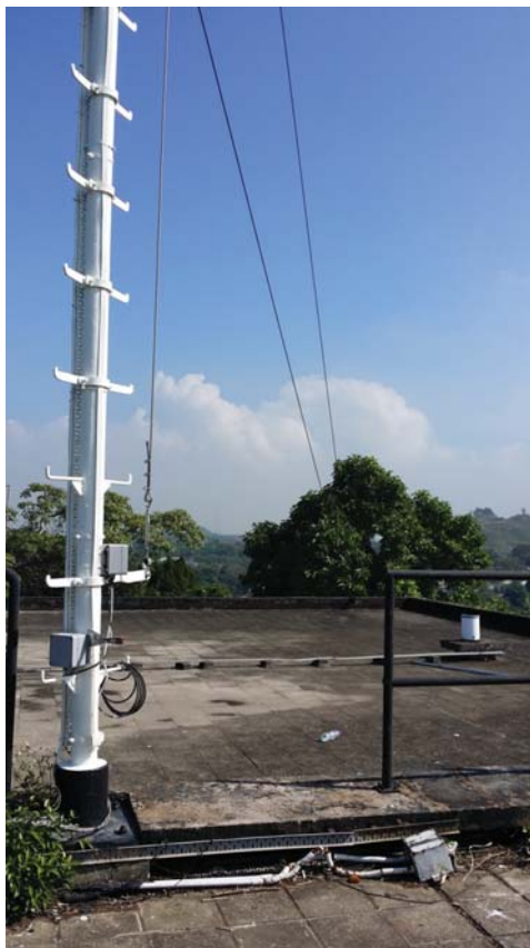
Base of the anemometer mast with guy wires
