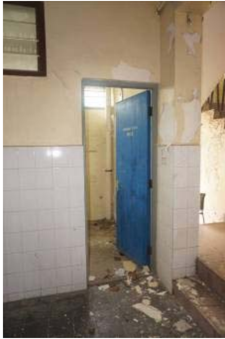
General view of the Workman Room
