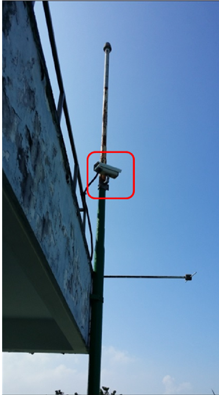
Existing HKO's instrument (weather camera) on Building Elevation facing North
