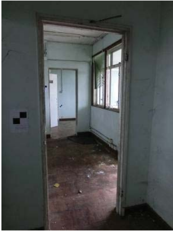
General view of the General Office
