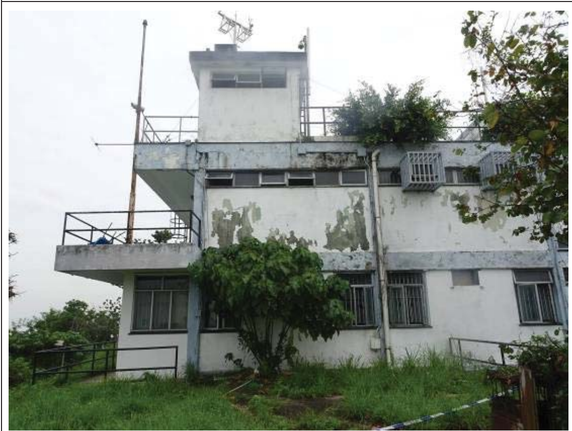
Rear elevation of Main Block
