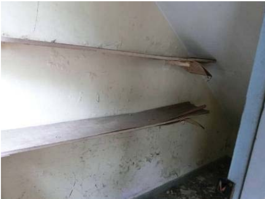
General view of the staircase at LG/F
