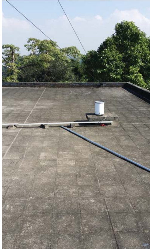
General view of the Main Roof and location of HKO's raingauge
