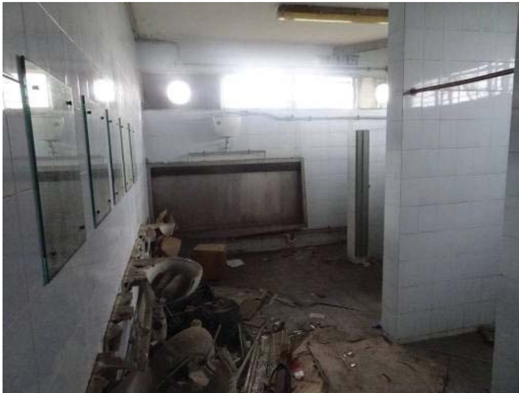
General View of Male Bathroom and Toilet at 1/F
