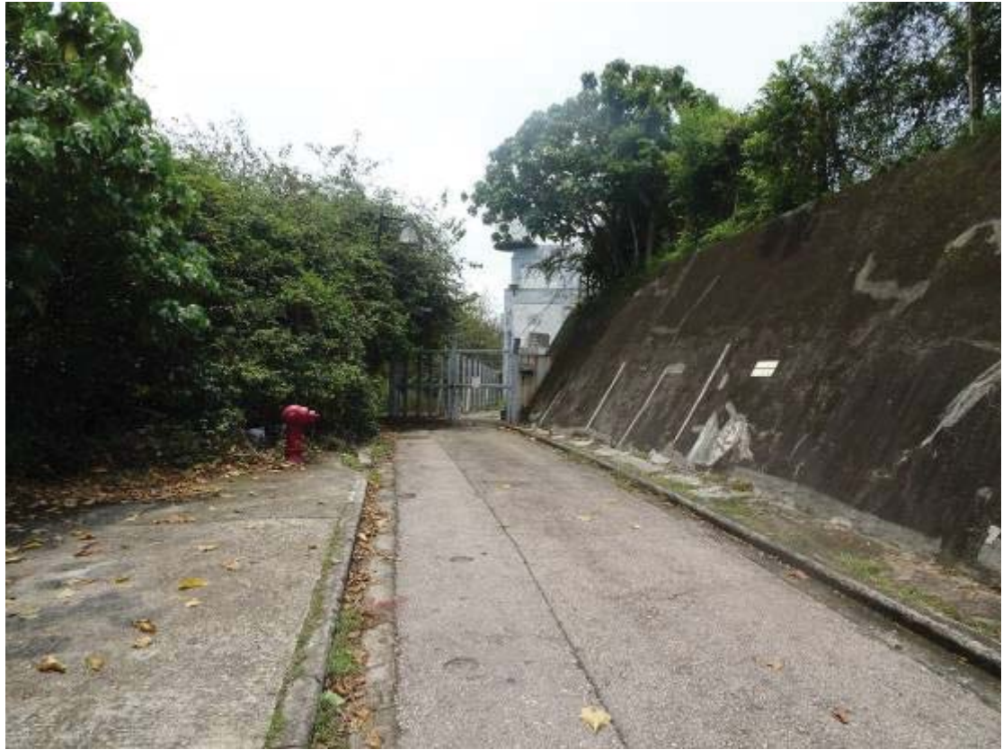
An access road connecting the Site to Lau Fau Shan Roundabout
