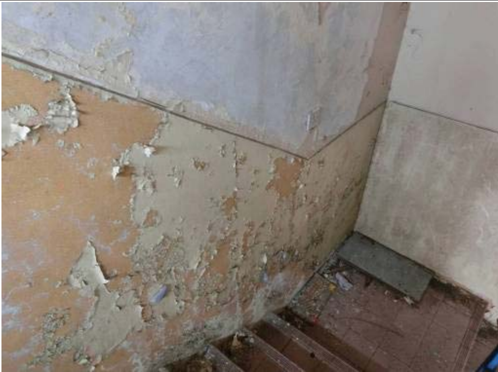
General view of the staircase between G/F and LG/F
