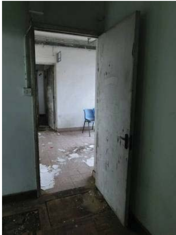
General view of Lobby 1
