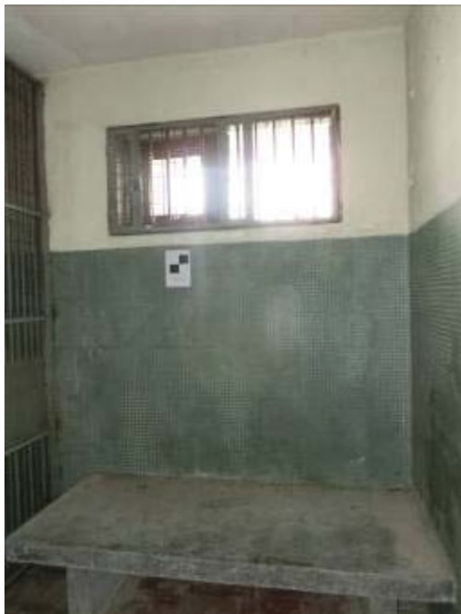
General view of the Cell Room
