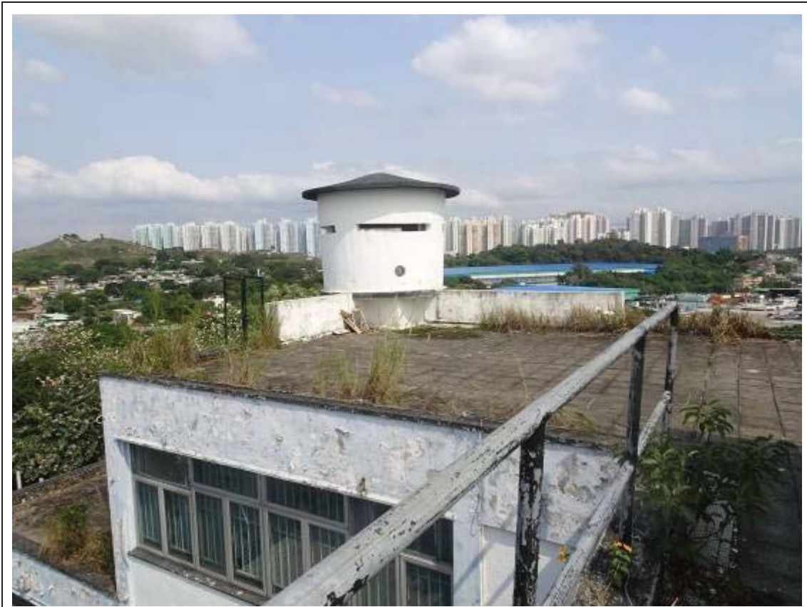
General view of the Main Roof
