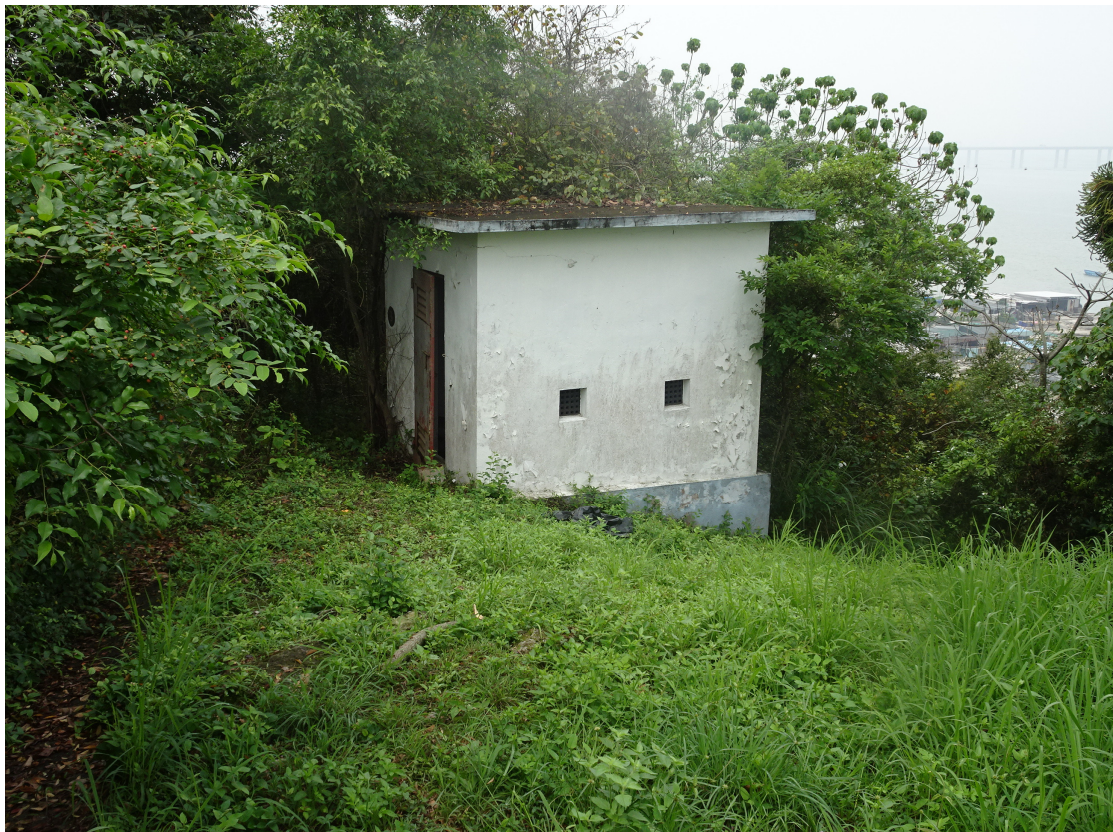
General view of Storage Shelter No.2
