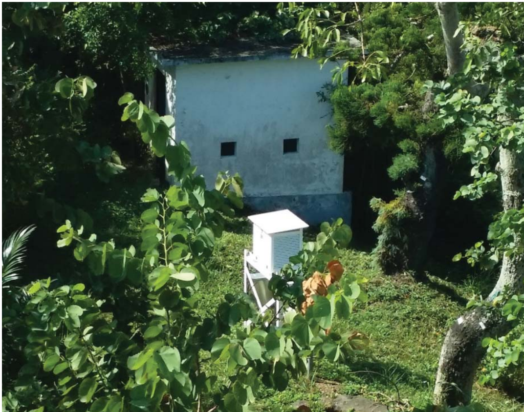
External weather monitoring instrument (HKO's Stevenson Screen for temperature and humidity measurement) and Storage Shelter No.2
