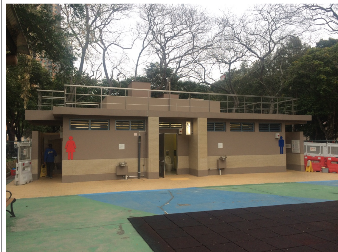
Photo 10 View of the Public Toilet in Luen Wo Hui Playground
