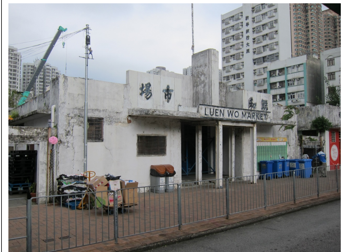
Photo 24 The strengthening work at the main entrance
