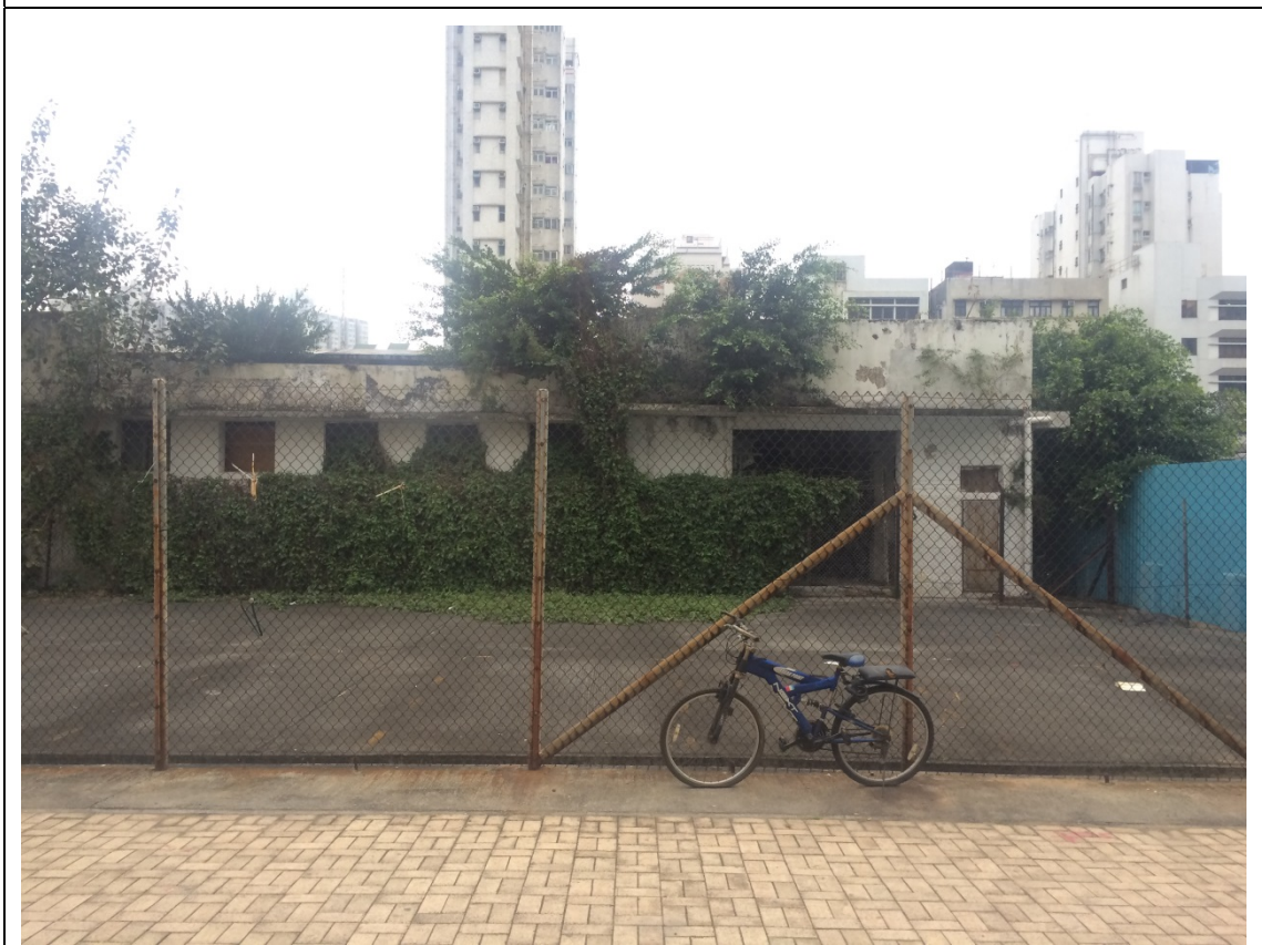
Photo 8 View of the Open Space abuts Luen Shing Street
