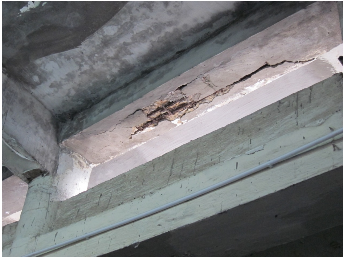
Photo 19 Example of the concrete spall on the bottom of beam
