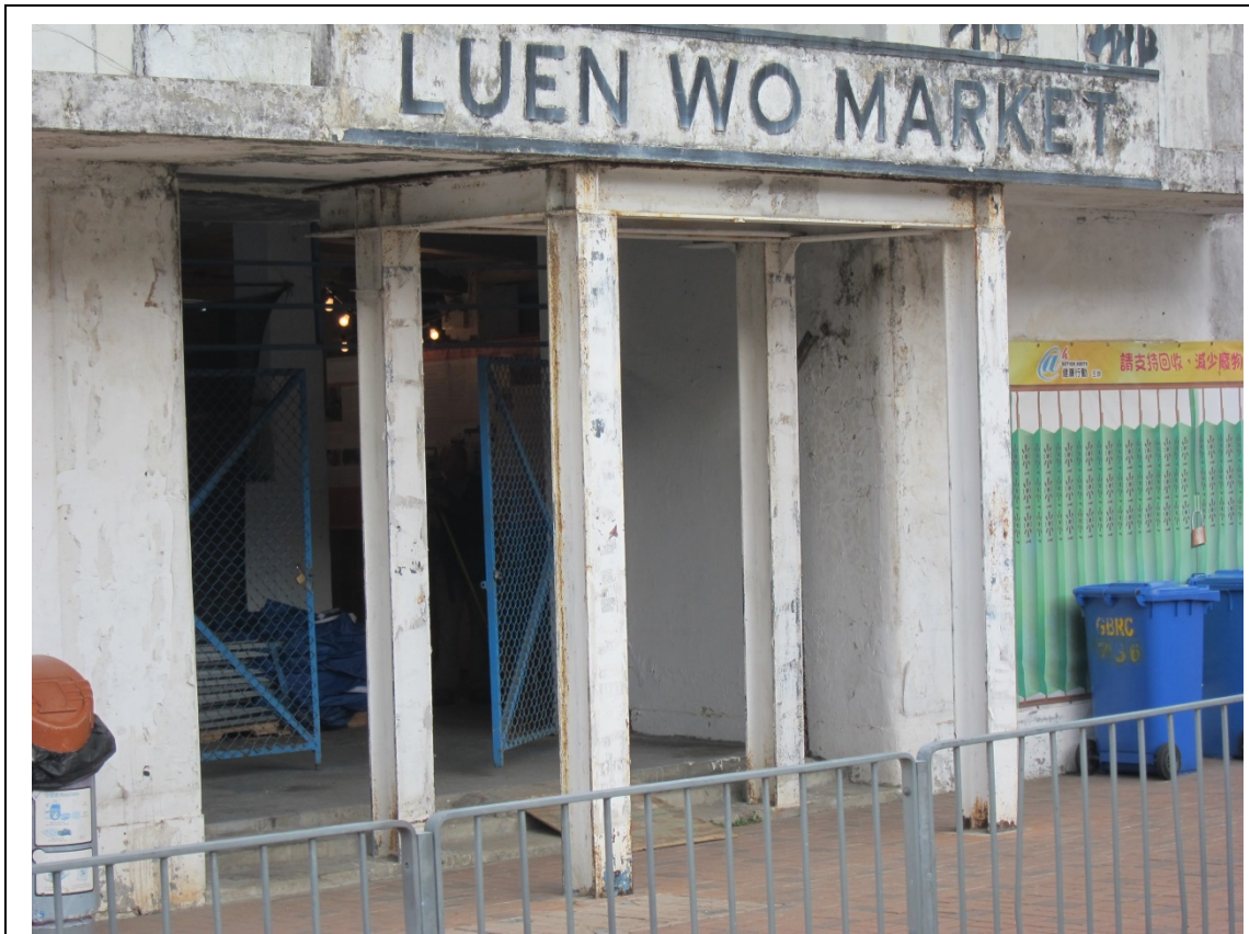
Photo 23 The strengthening work at the main entrance
