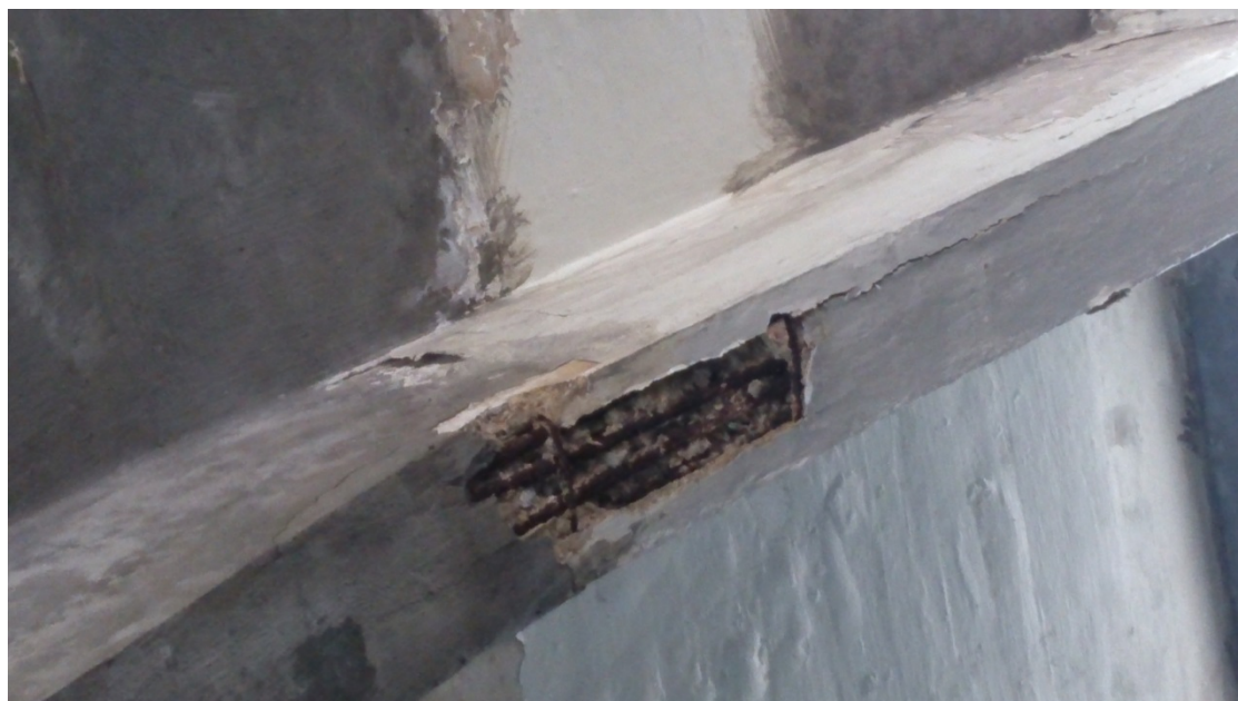
Photo 19 Example of the concrete spall on the bottom of beam
