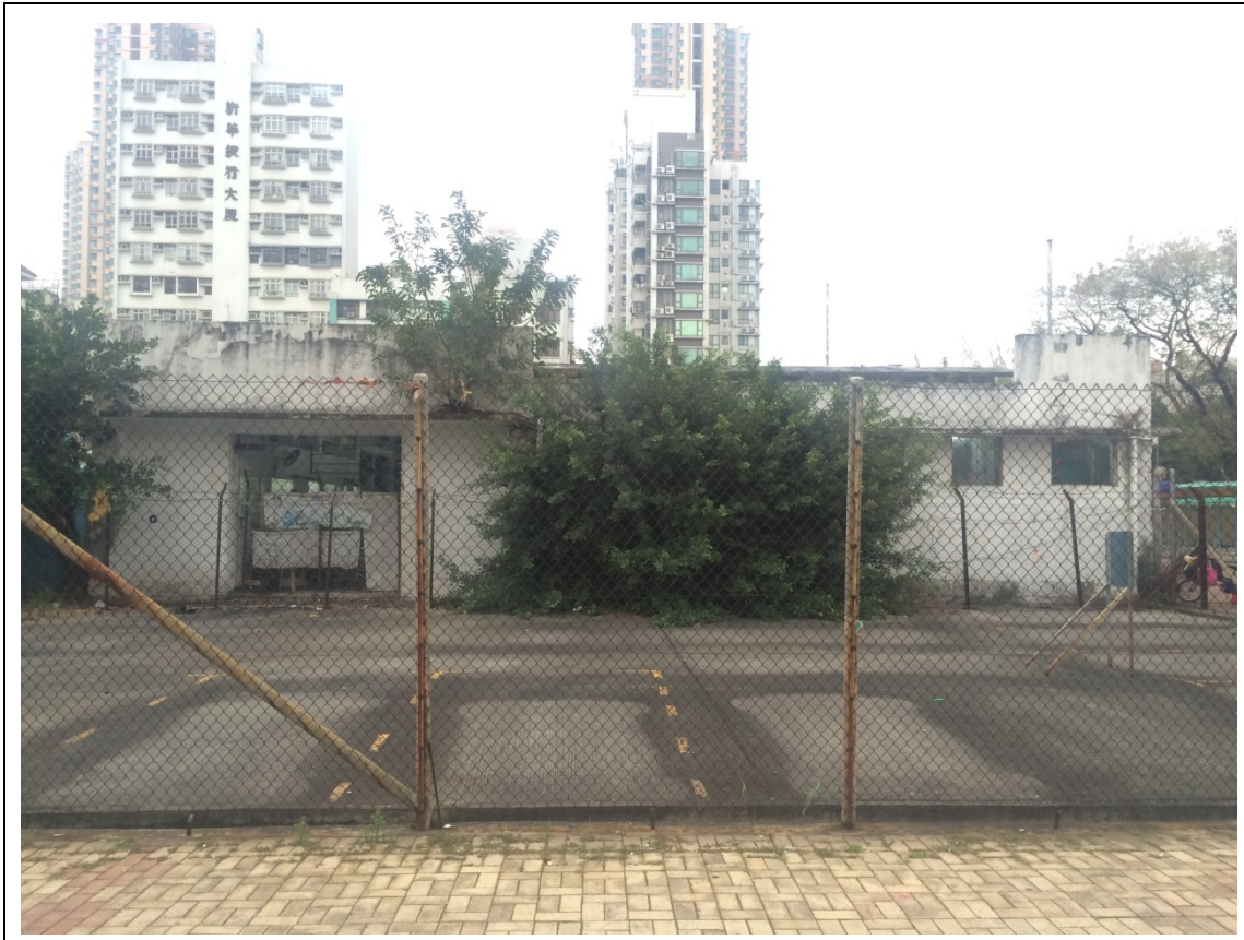
Photo 7 View of the Open Space abuts Luen Hing Street
