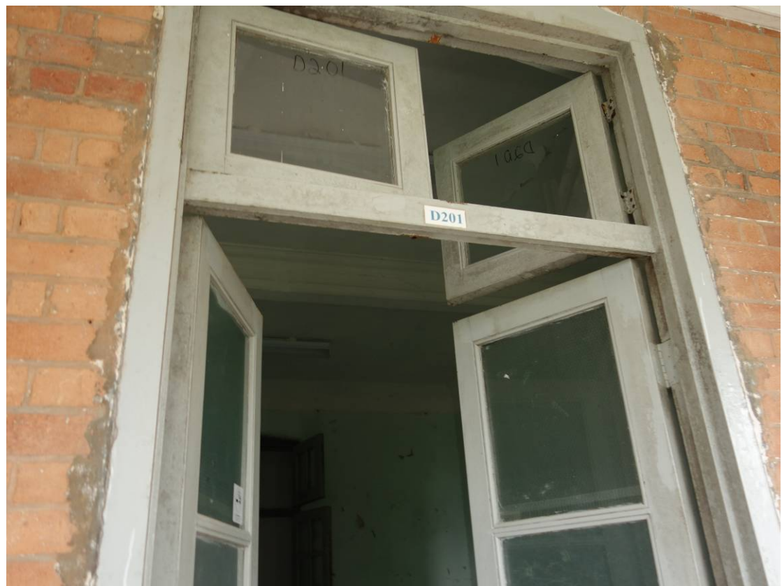
General view of the door at room D201
