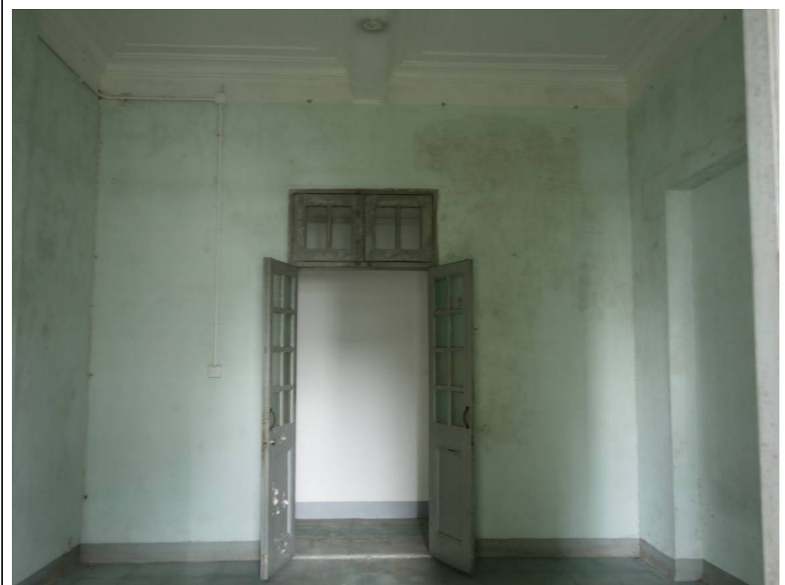
General view of room D301 at 2F
