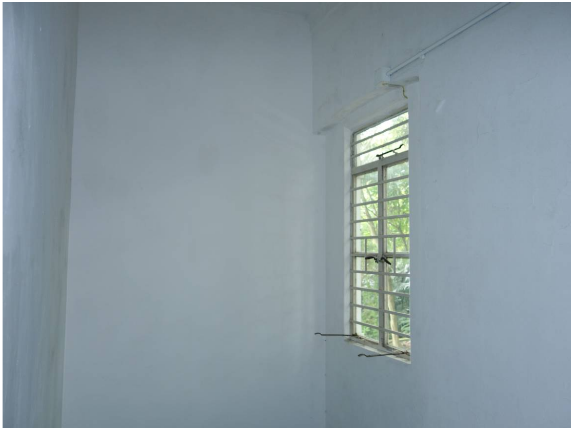
General view of room S212 at 1/F
