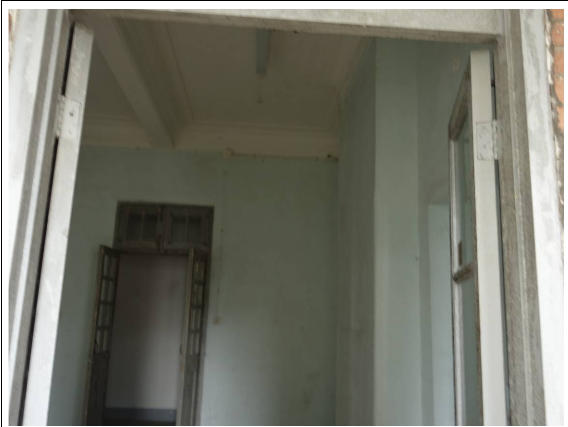
General view of room D302 at 2/F
