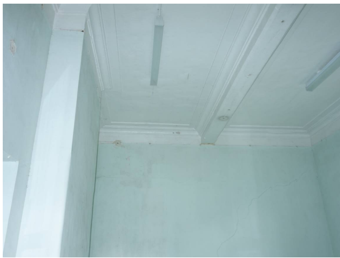
General view of room D303 at 2/F
