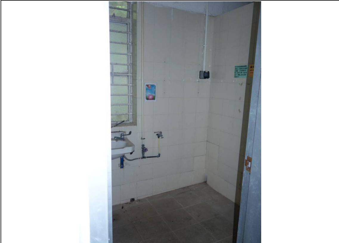
General view of Lavatory at 2/F
