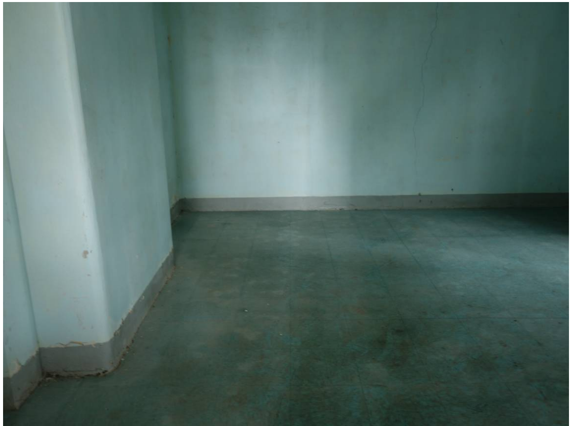
General view of room D203 at 1/F
