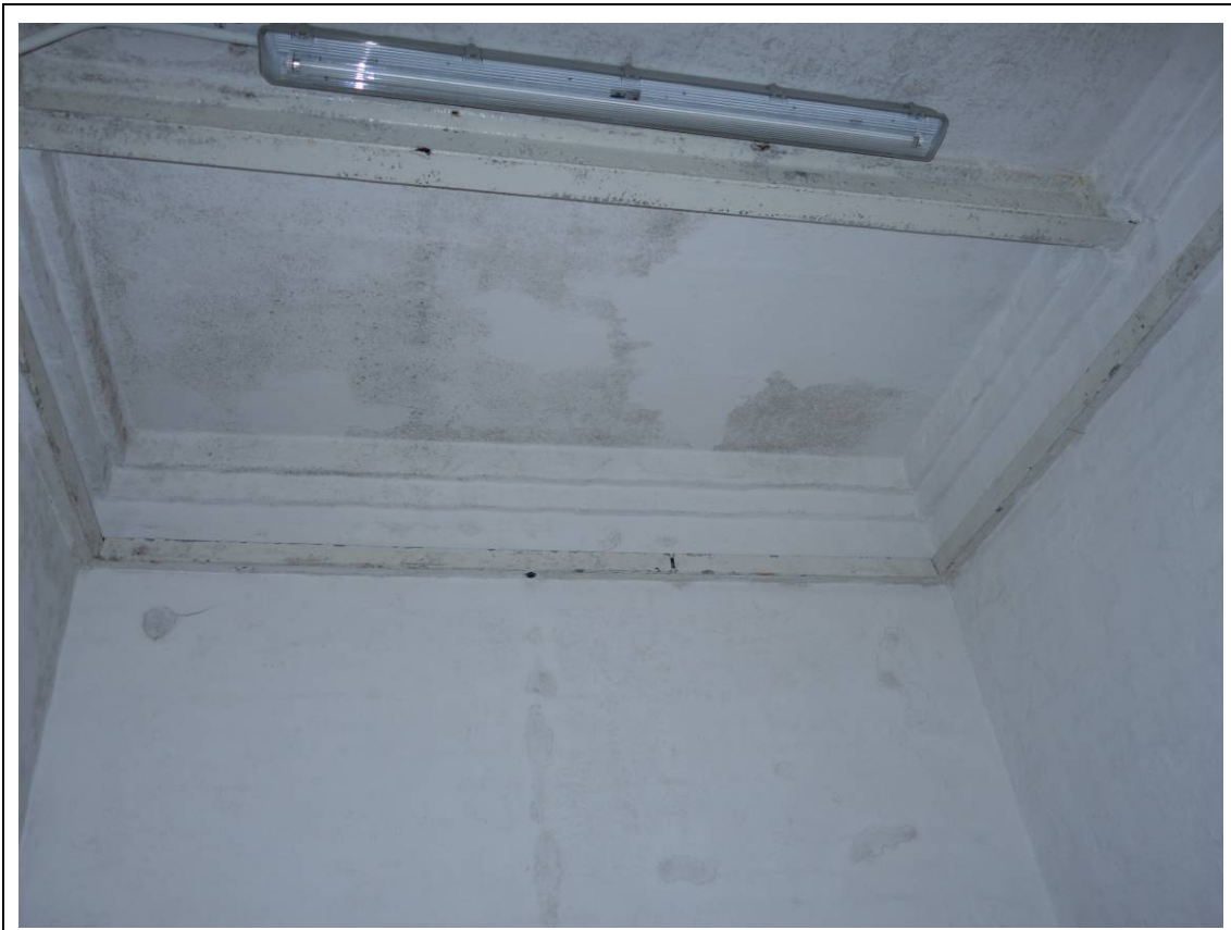
General view of ceiling of kitchen 1/F
