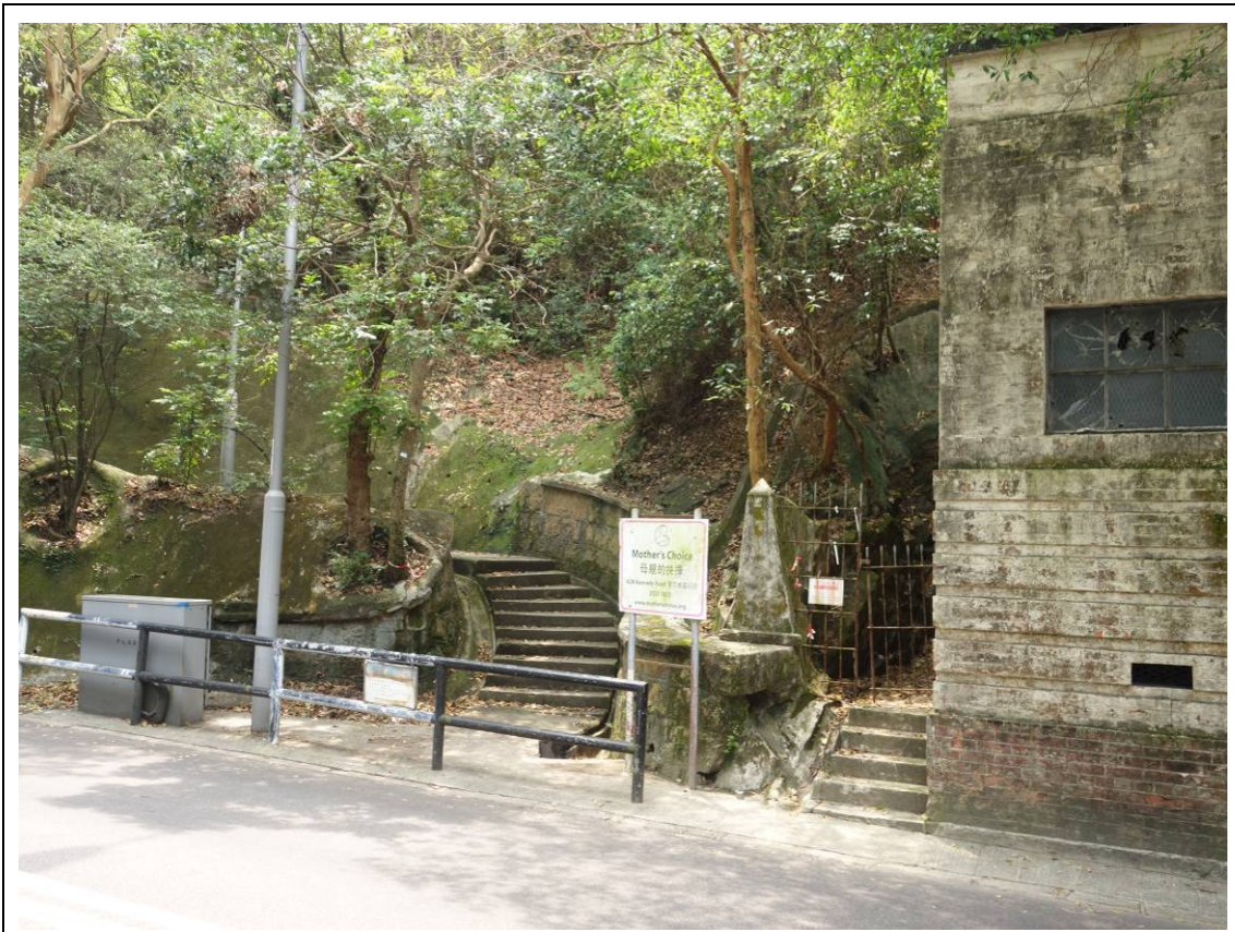
An access staircase connecting the Site to Kennedy Road
