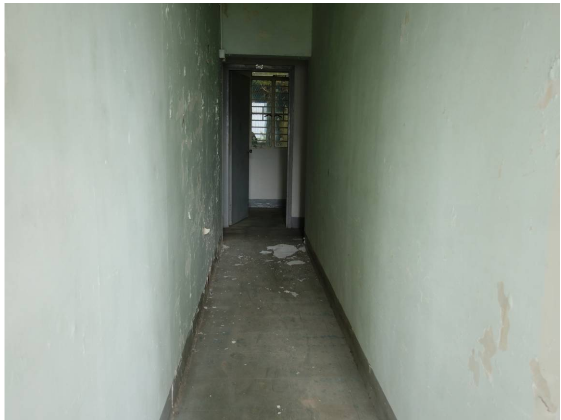
General view of indoor corridor at 1/F
