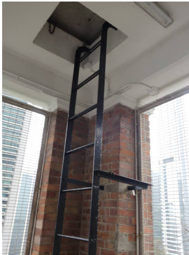
Cat ladder accessing to the roof
