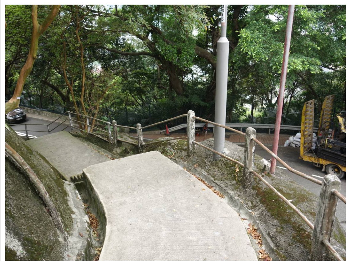
General view of access staircase connecting the Site to Kennedy Road
