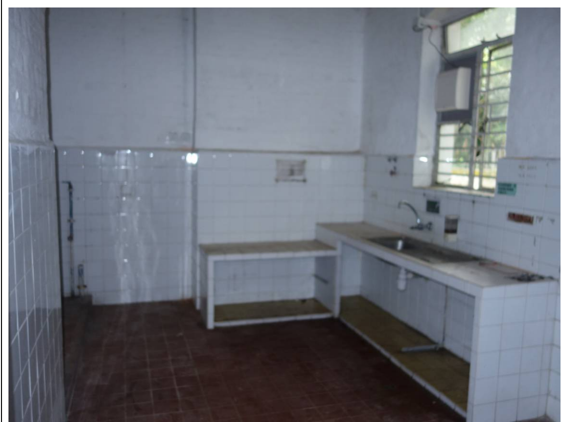
General view of Kitchen at G/F
