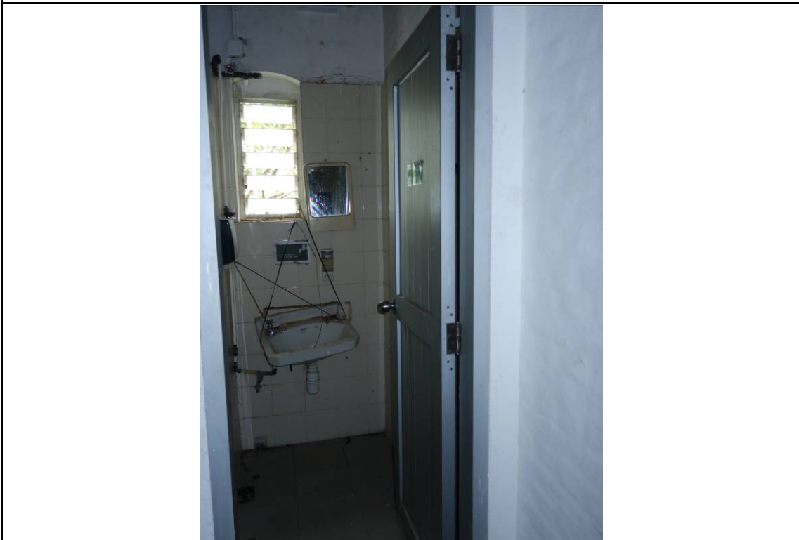
General view of Bathroom at 2/F
