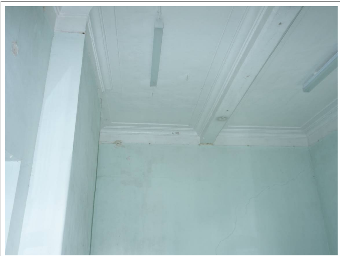
General view of room D303 at 2/F
