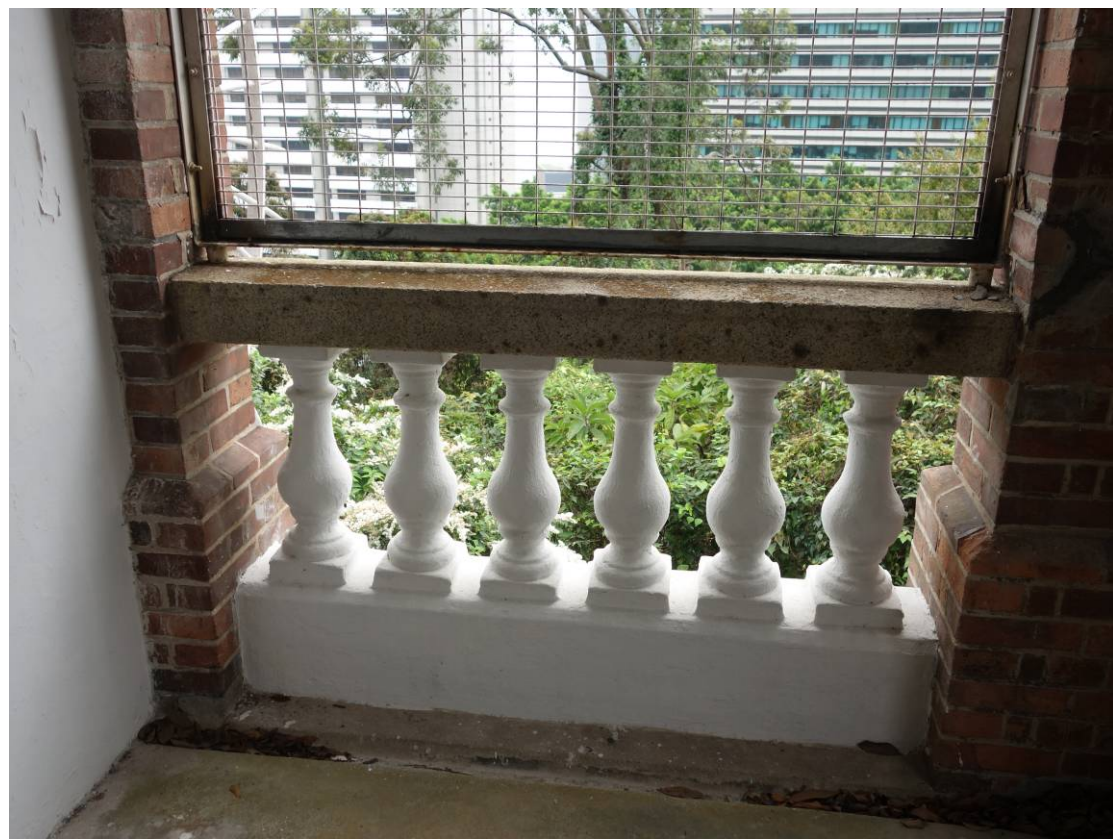
General view architectural feature at 1/F
