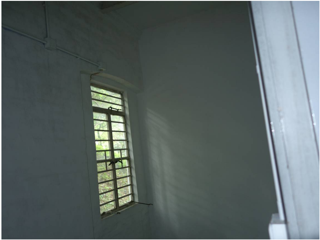
General view of room S213 at 1/F
