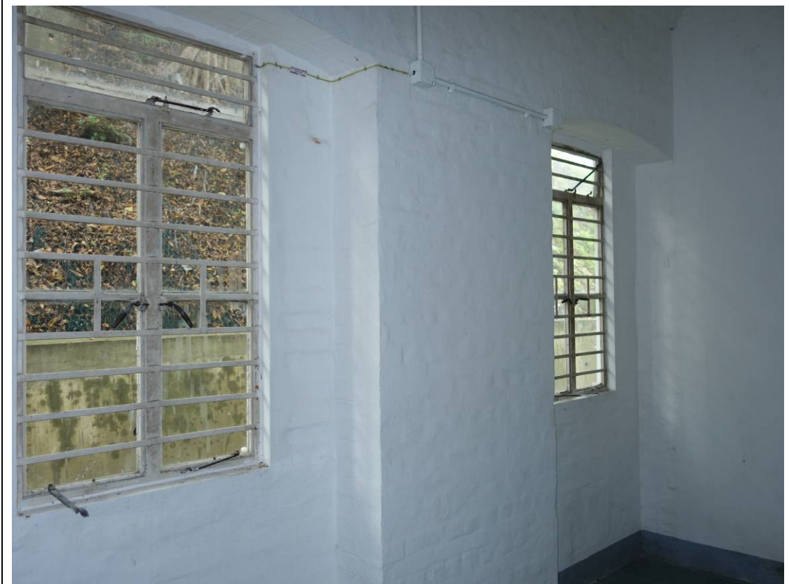
General view of room S112 at G/F
