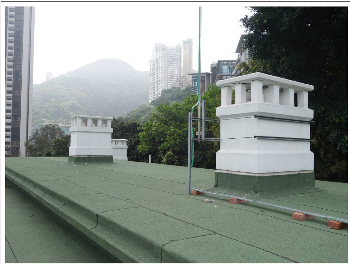
General view of the roof of the Roberts Block
