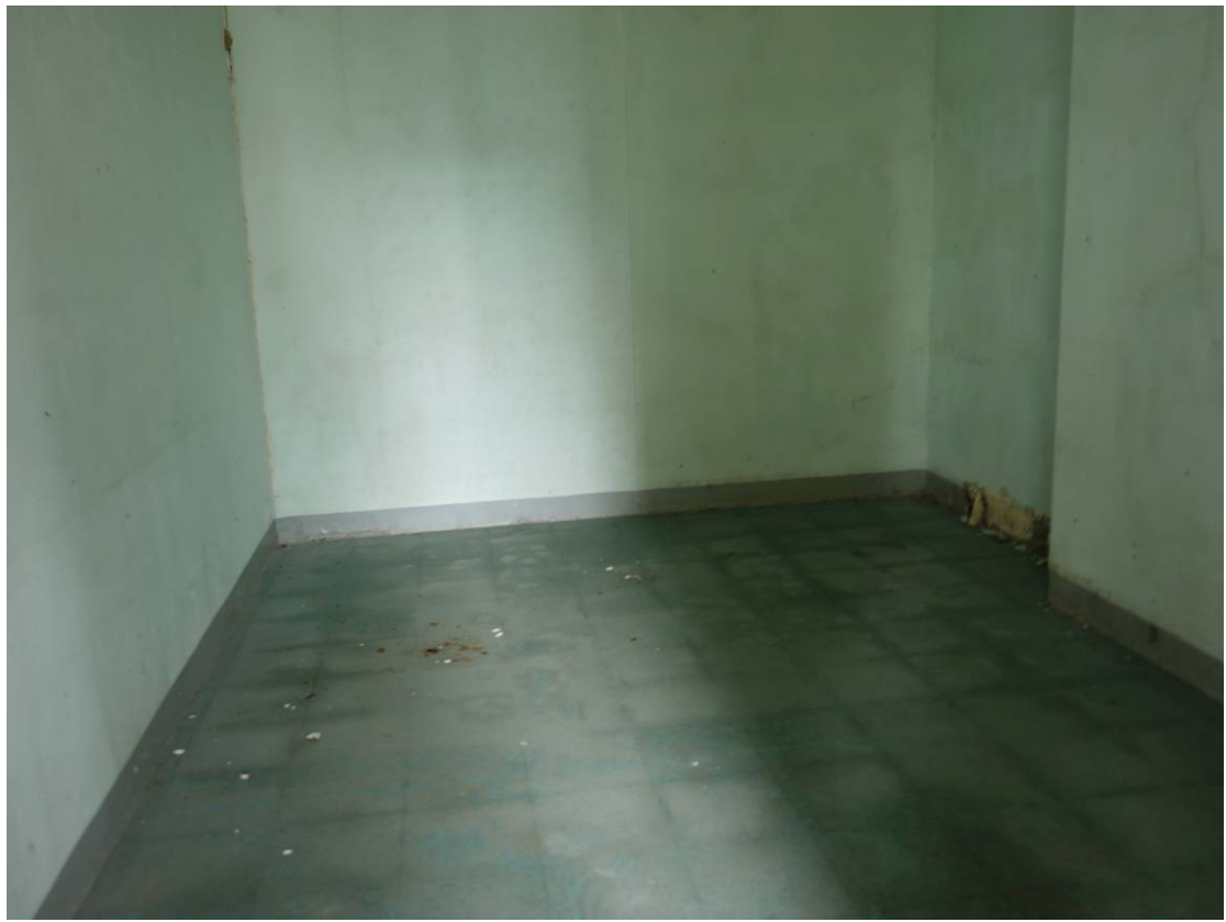
General view of room D202 at 1/F
