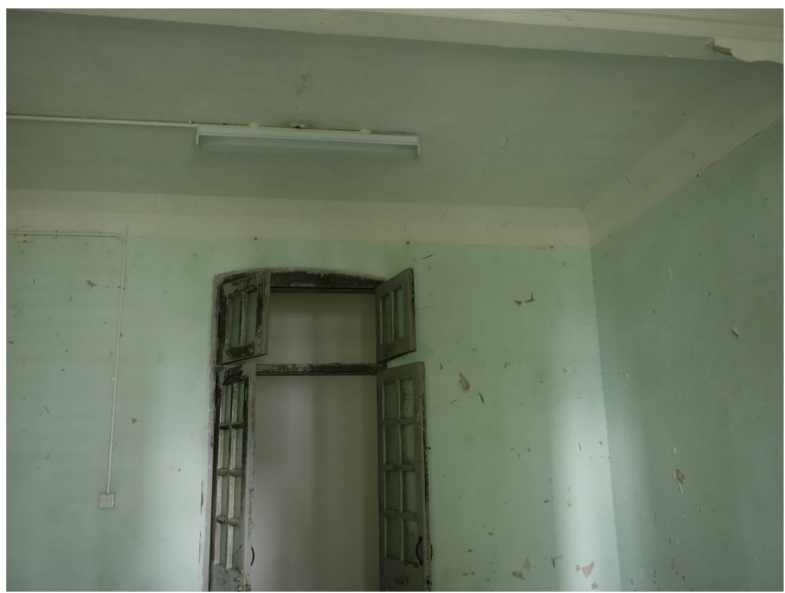
General view of room D201 at 1/F
