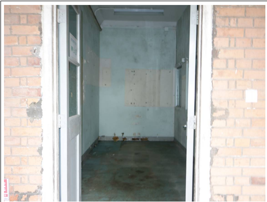
General view of Office at G/F
