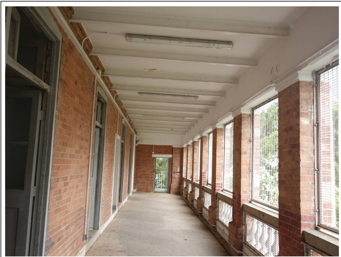
General view of Veranda at 1/F
