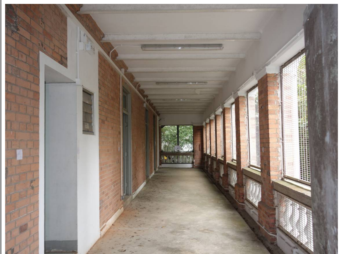
General view of Veranda at G/F
