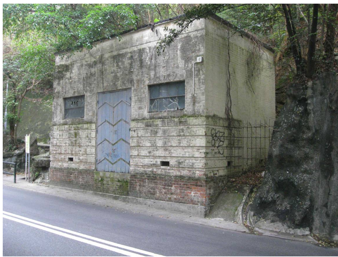
General view of substation facing Kennedy Road
