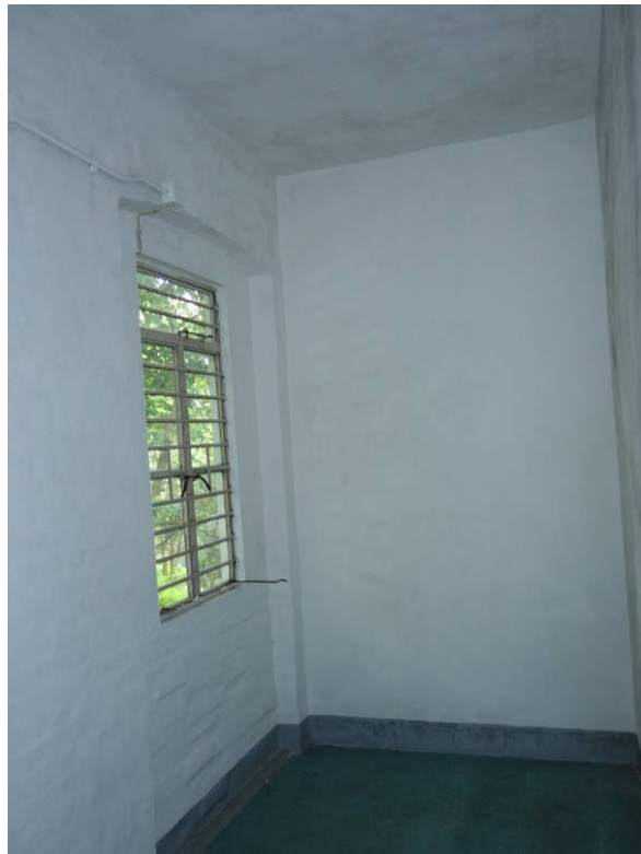
General view of room S313 at 2/F
