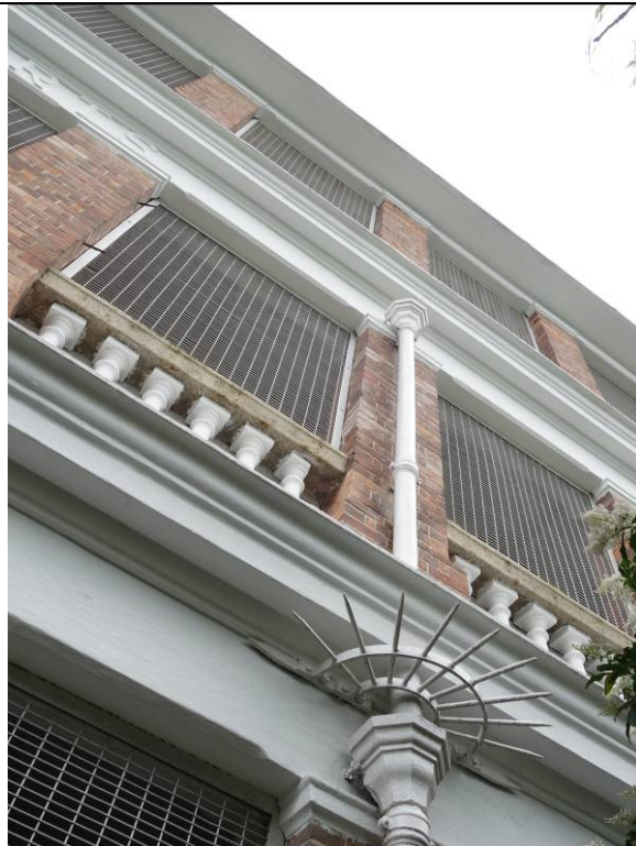
Front elevation of the Roberts Block
