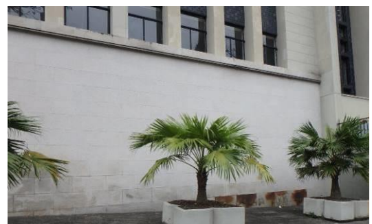
Plain ashlar-faced retaining wall along north side of LG/F
