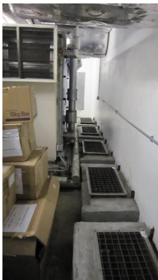
Ducts Room (Grid A-C)
