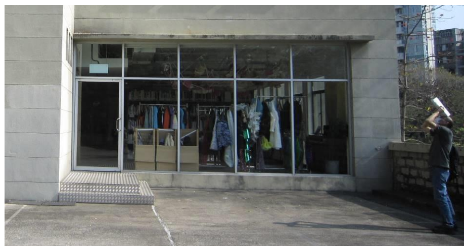
Original wall opening for the old Magistrate's Garage
