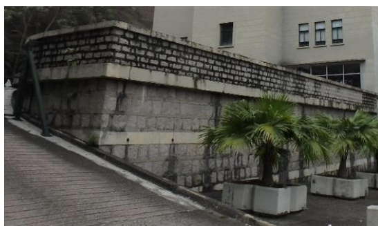
Stone facing low parapet wall at the North Open Forecourt
