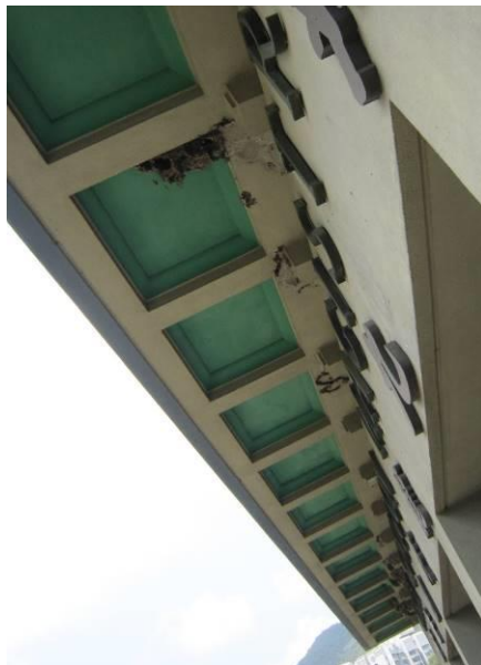
Cornice mouldings at the soffit of the overhanging coping slab
