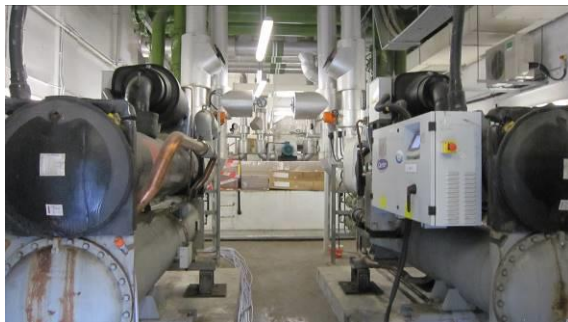
Existing AC Plant Room
