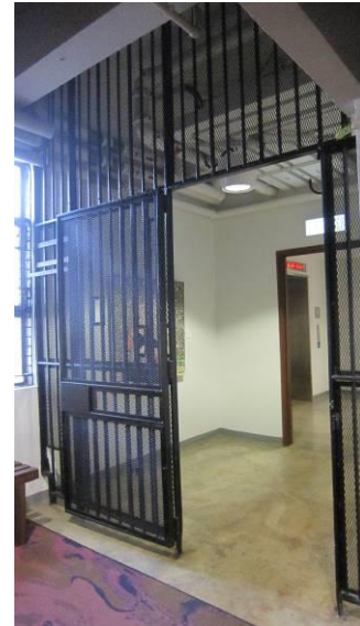
Metal guard bars, grilles and metal gates of the old Detention Cell no. 7
