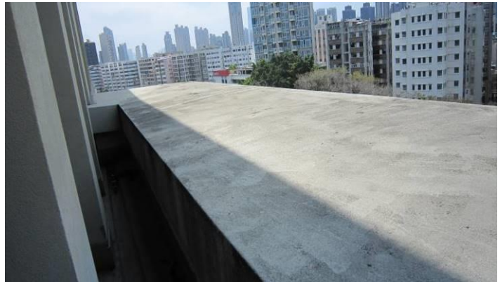
Solid parapet with deep overhanging coping
