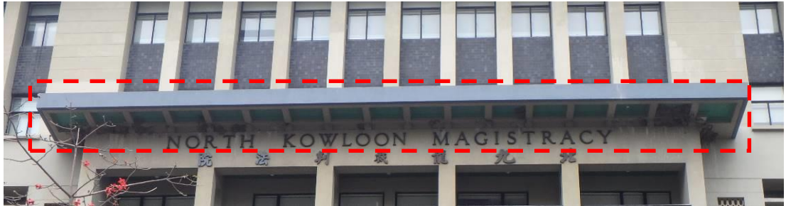
Roof terrace with solid parapet on 4/F
