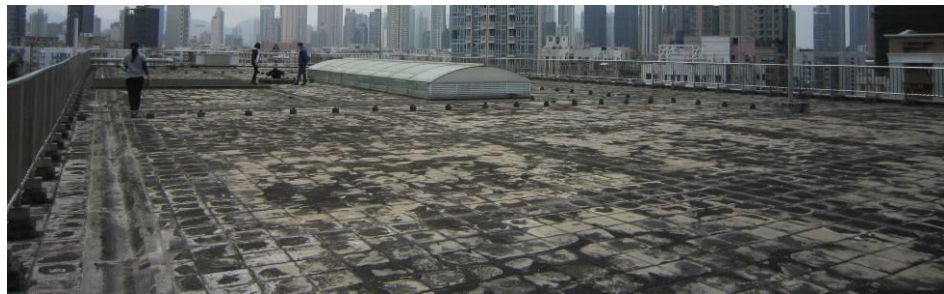
Open flat roof
