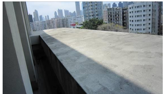
Solid parapet with deep overhanging coping
