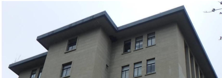
Projecting roof eave
