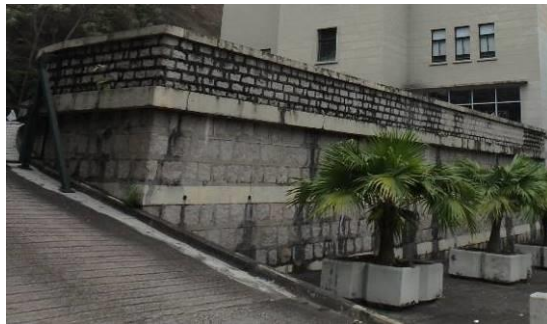
Stone parapet wall at the North Open Forecourt
