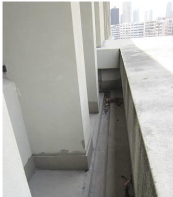
Roof terrace with surface channel
