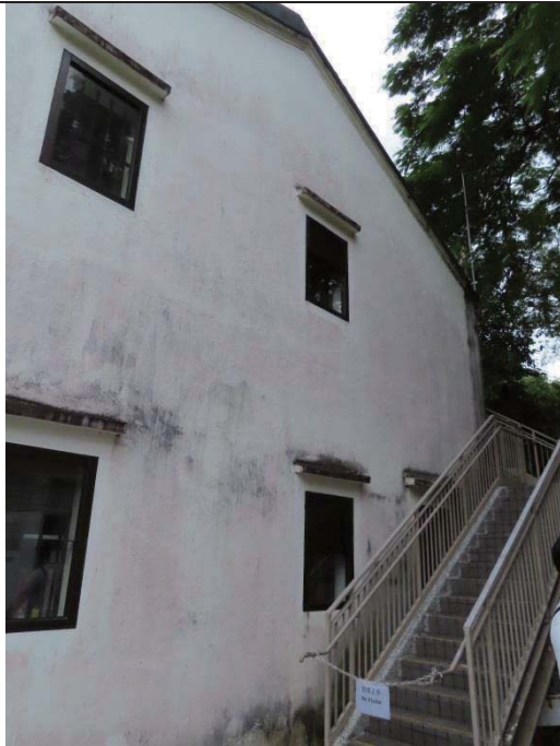
Side Elevation and External Staircase
