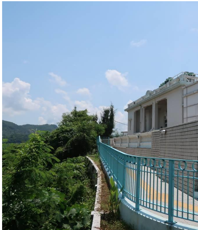
Main Building (Main Entrance, North-East Elevation)
