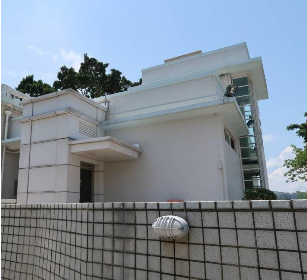
Extension (North-East Elevation)
