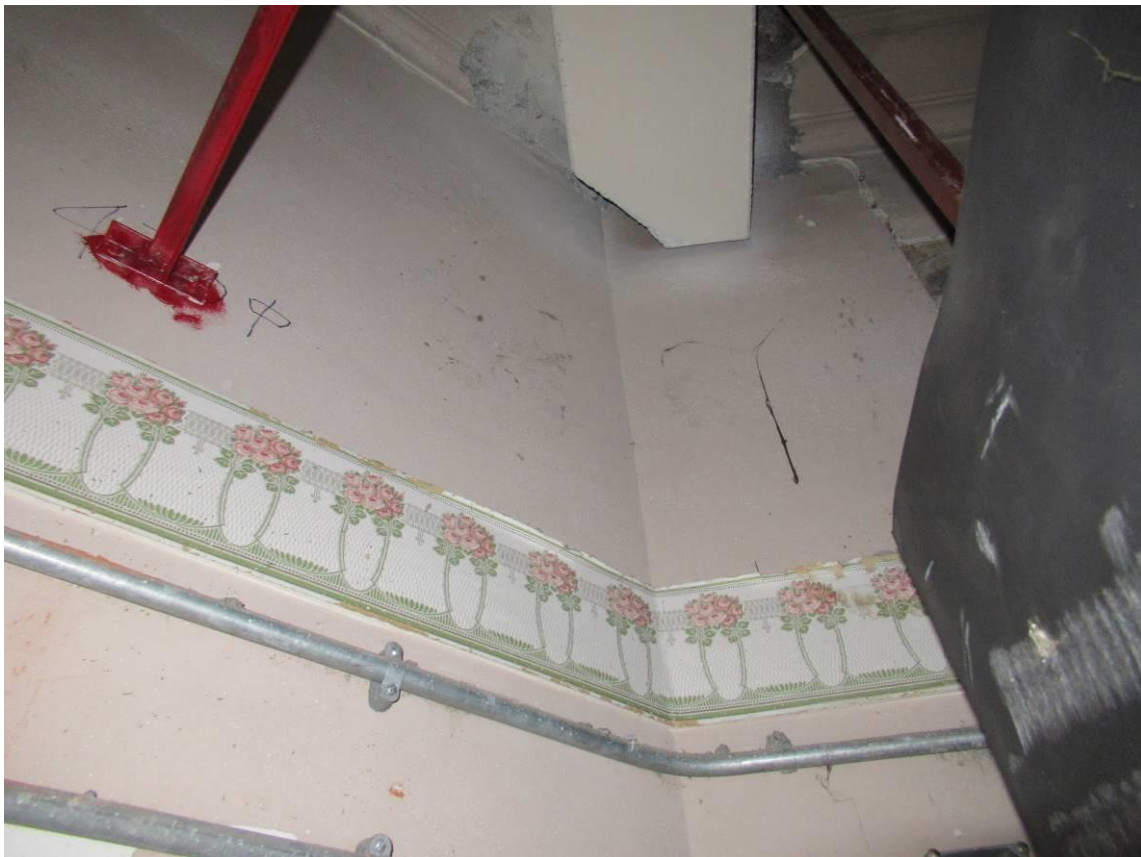
Condition above the false ceiling at Main Building
