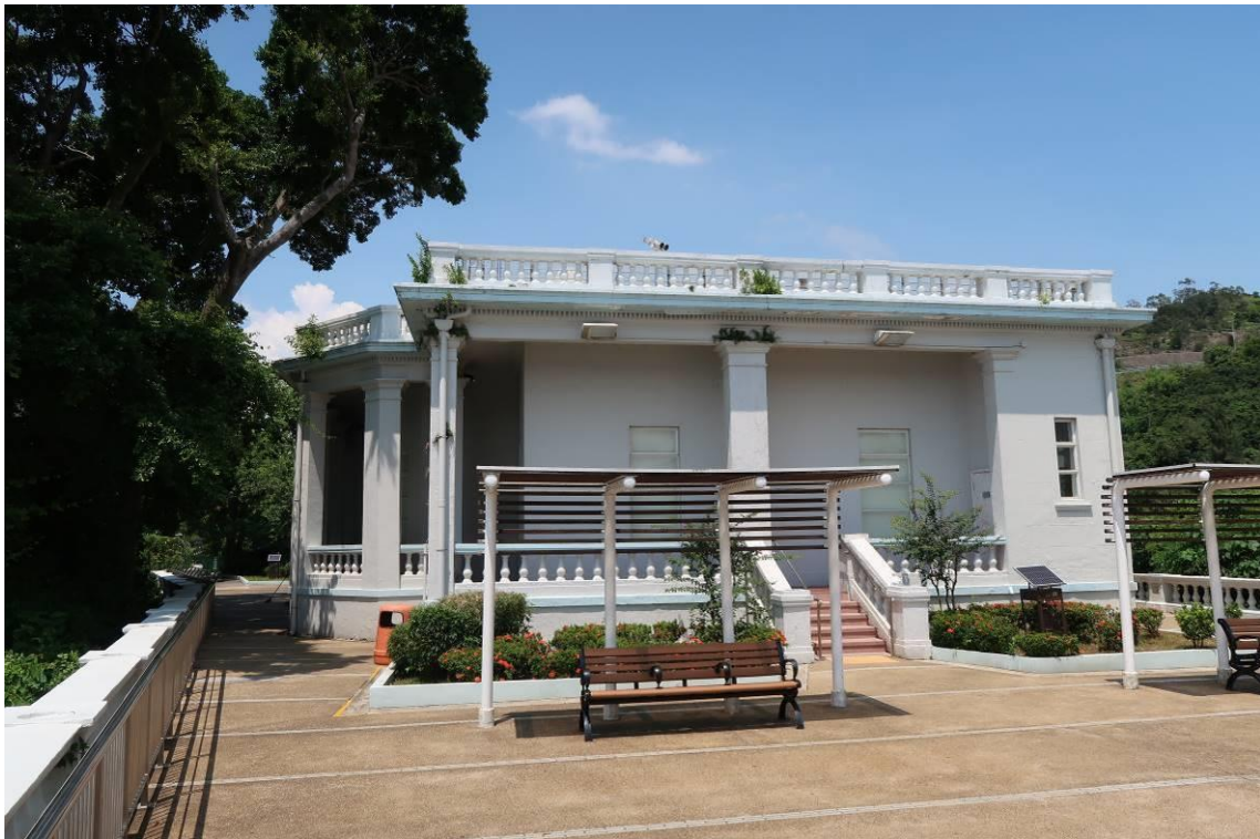
Main Building (South-East Elevation)
