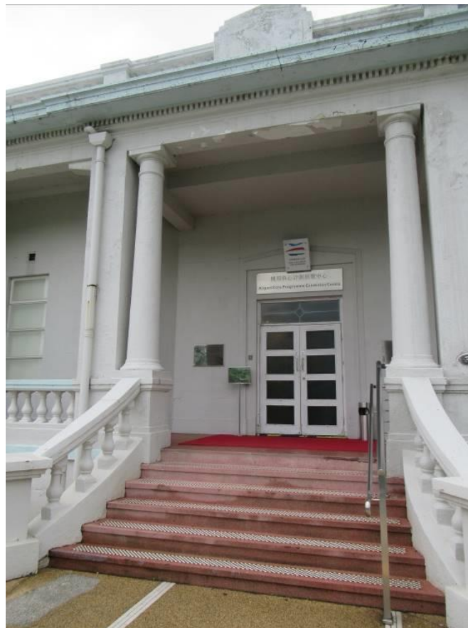
Main Entrance to Main Building
