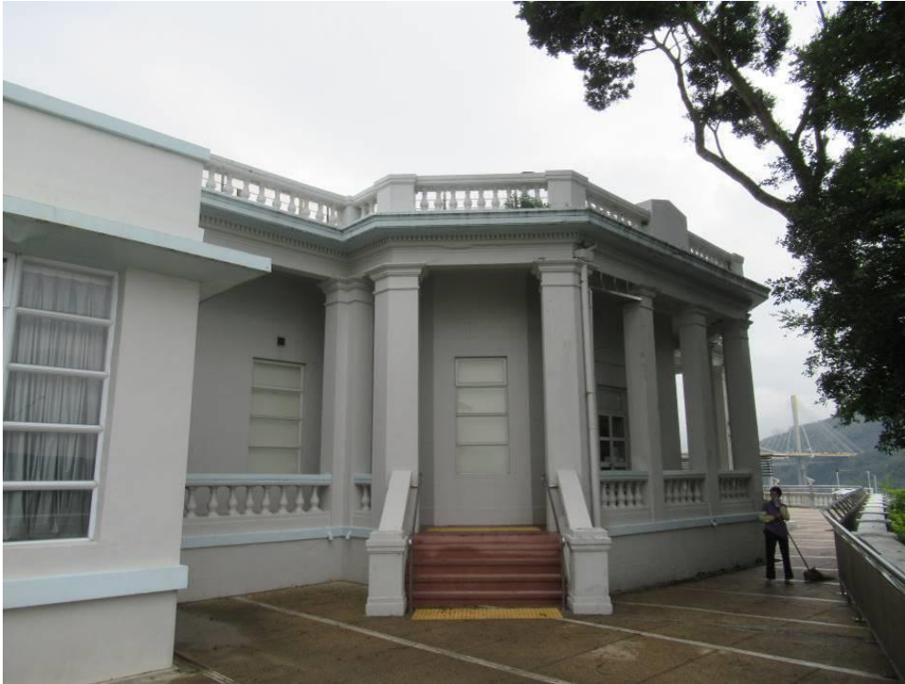
Rear Entrance to Main Building
