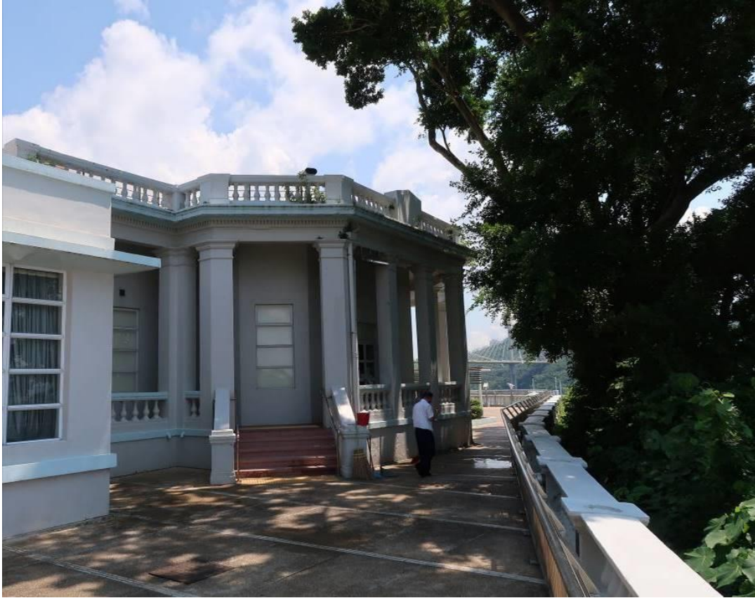
Main Building (South-West Elevation)
