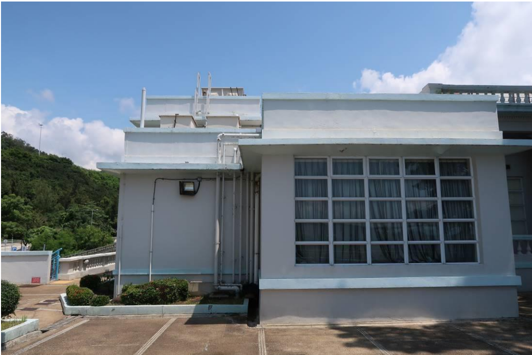
Extension (South-West Elevation)
