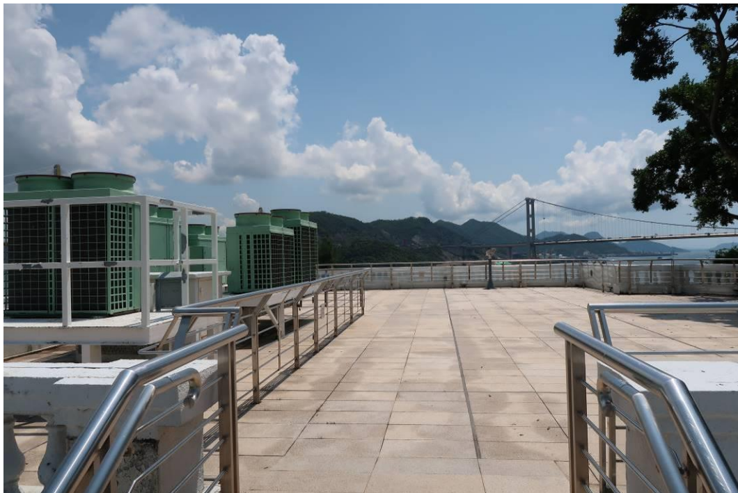
View of Main Roof (Photo taken at roof of Extension)
