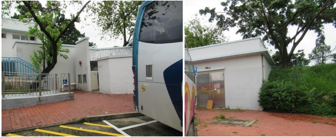
Ancillary Building (R.C.P. & Electrical Substation)
