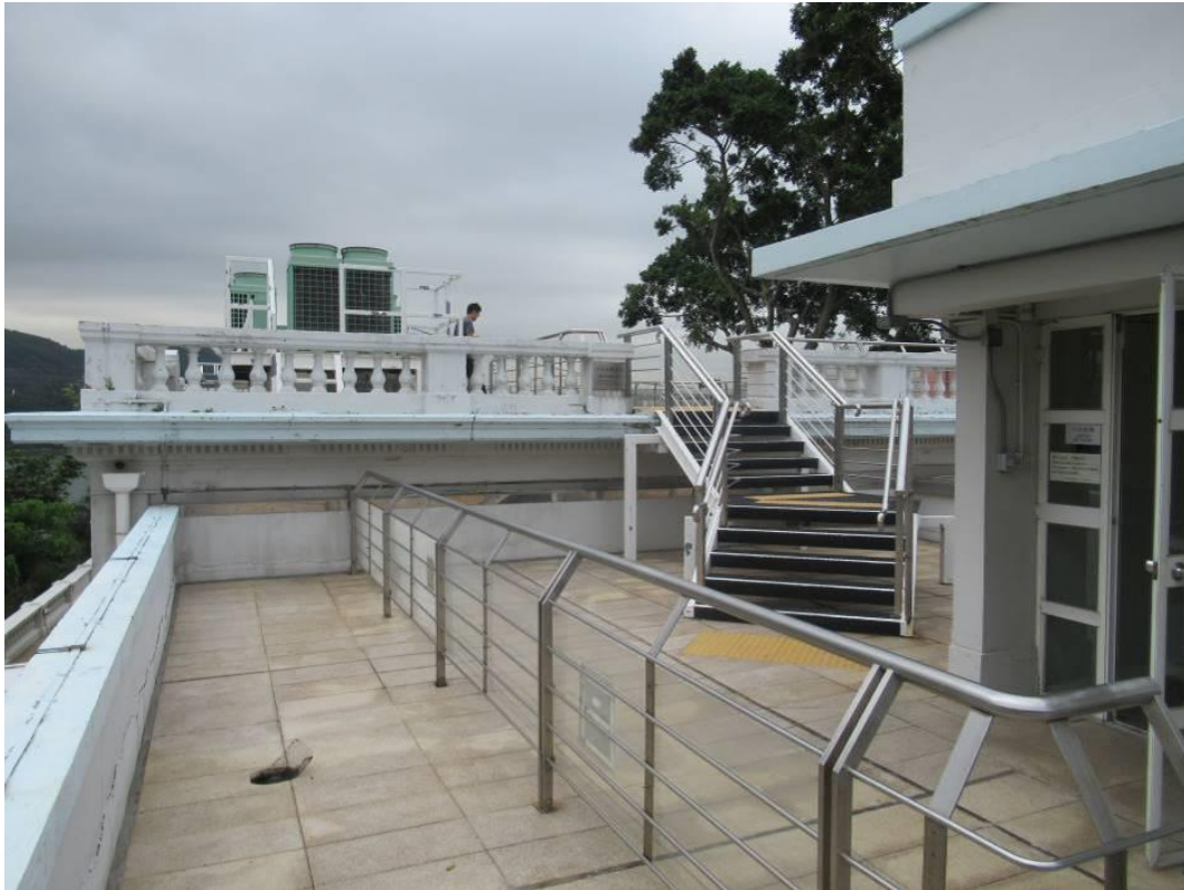
View of Main Roof (Photo taken at roof of Extension)
