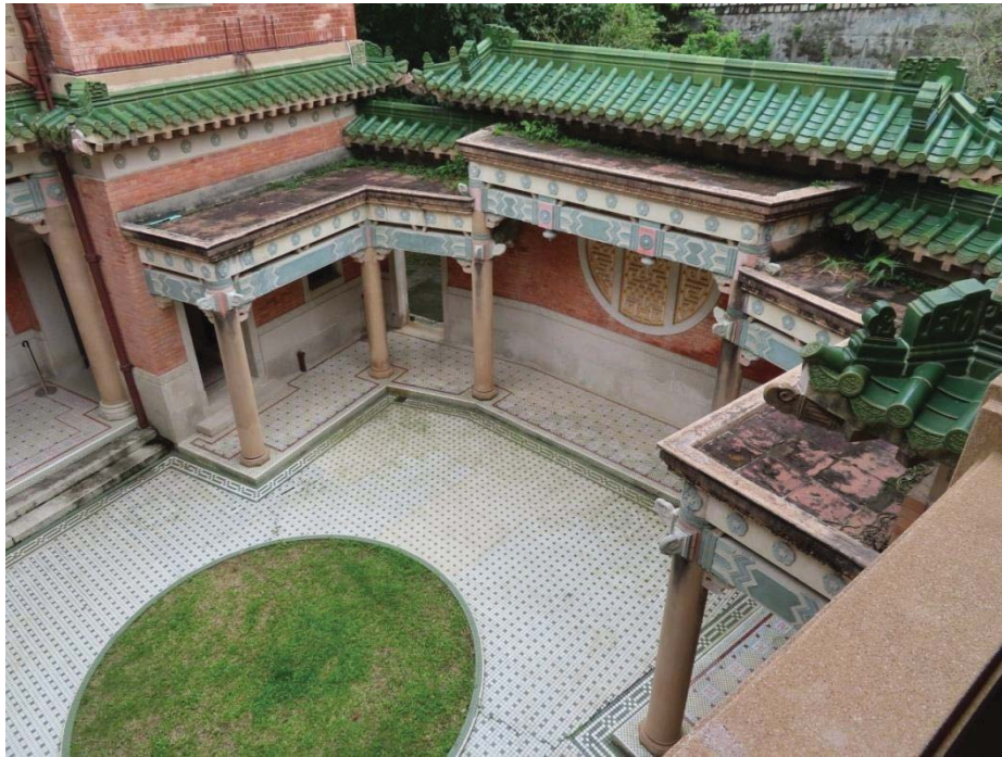
2.9 View of Courtyard of Main Building
