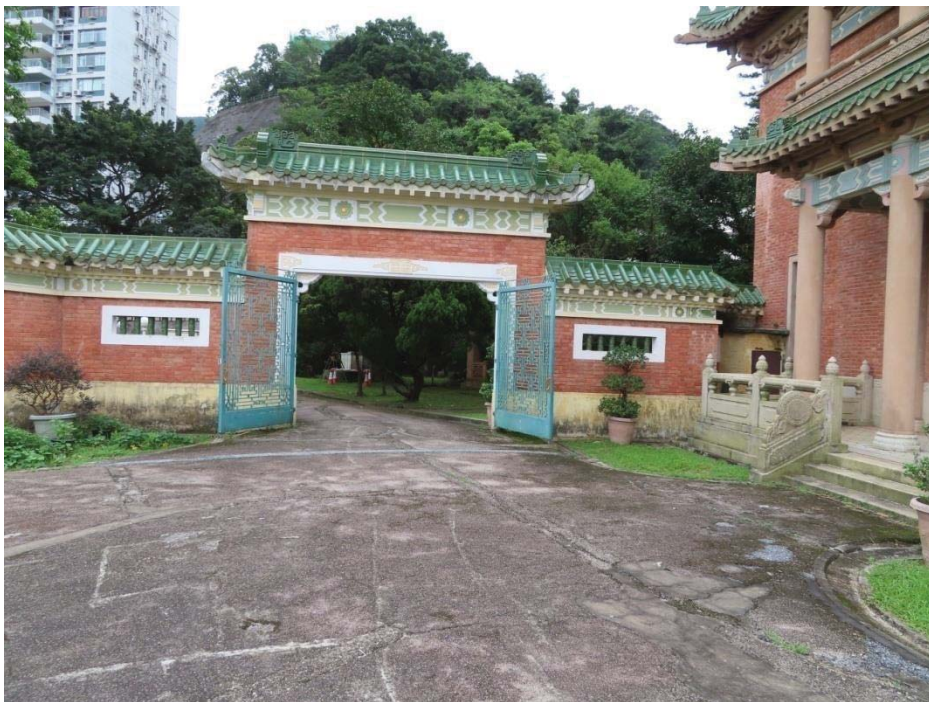
1.6 View of Interior Gateway
