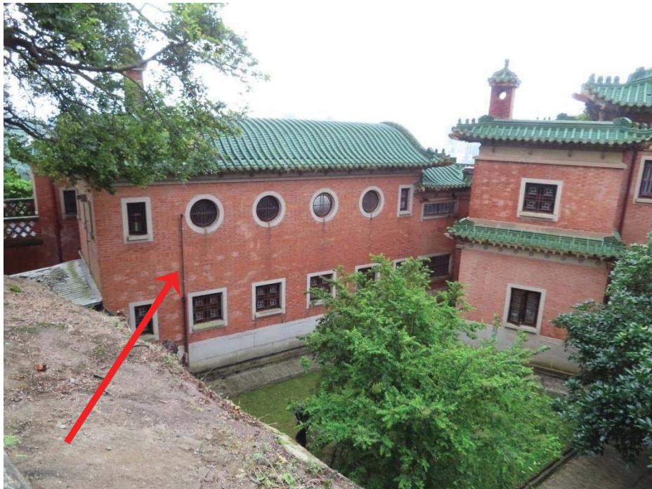
2.4 View of Annex Block from Stubbs Road
