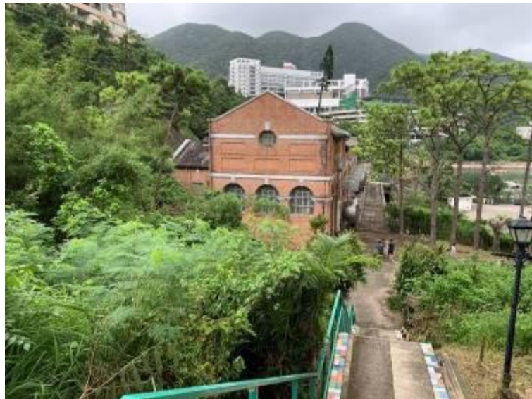
Slope at the west side of Senior Staff Quarters
