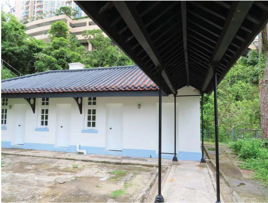
3.1 View of Senior Staff Quarters - Servants' Quarters
