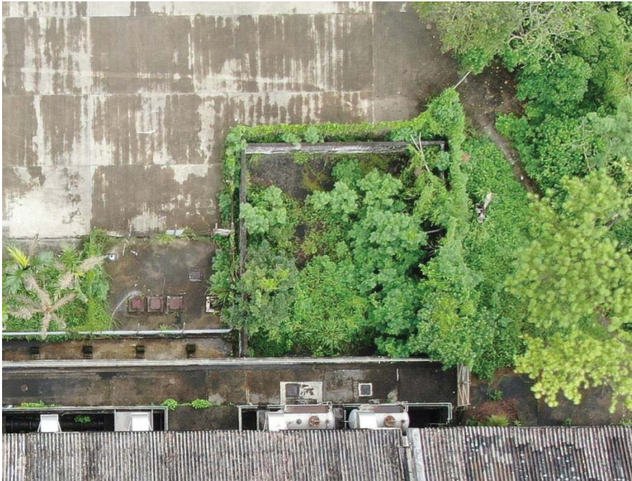
10.1 Aerial view of Fuel Tank
