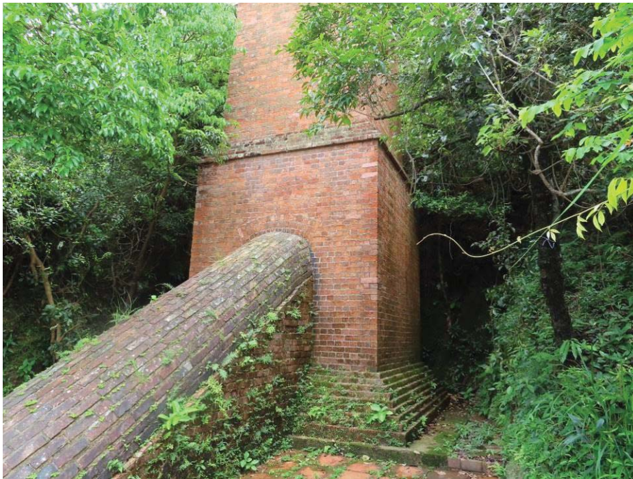
14.2 View of Chimney Shaft and its Flue
