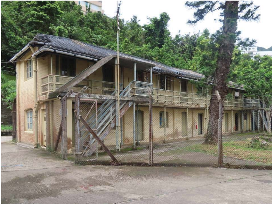
4.1 View of Staff Quarters - Main Building
