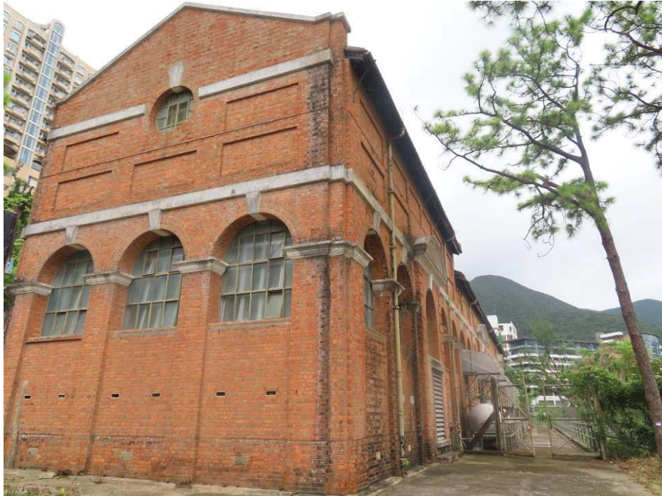
13.3 View of Pumping Station
