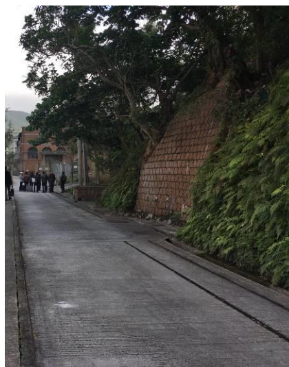
Slopes/ retaining walls at the north side of No. 2 Staff Quarters
