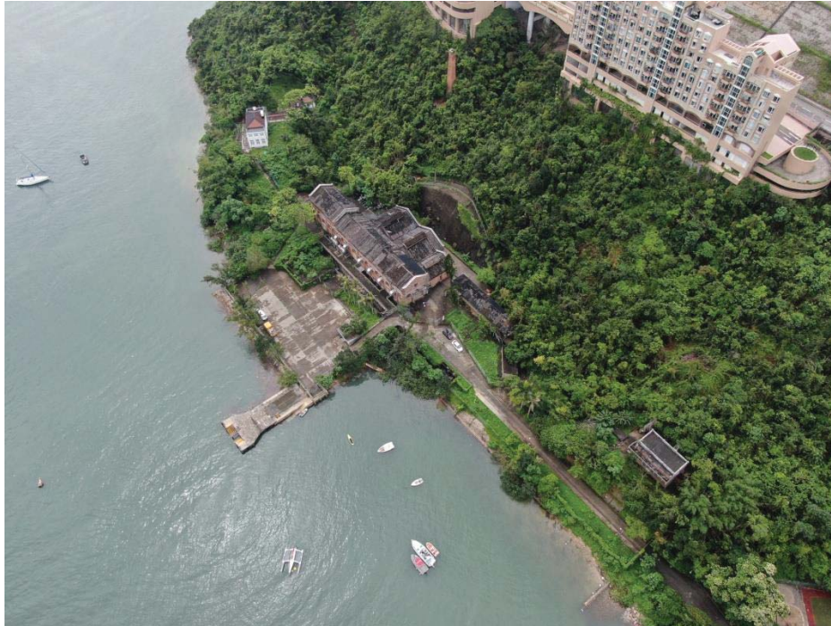
1.1 Aerial View of Tai Tam Tuk Raw Water Pumping Station Staff Quarters Compound
