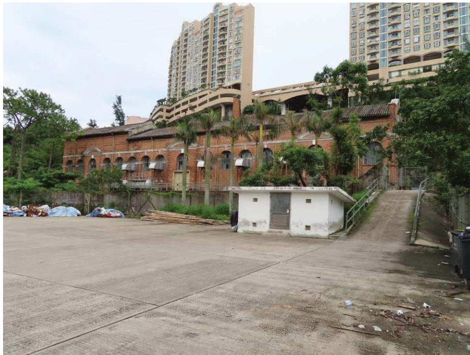
13.4 View of Pumping Station
