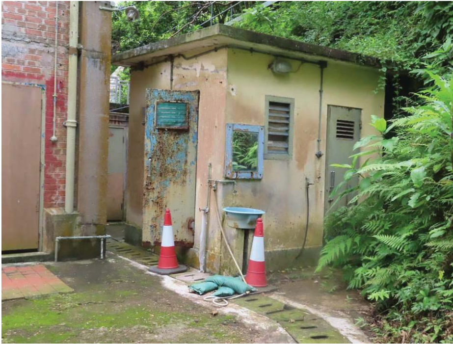
7.1 View of No. 2 Staff Quarters - Outbuilding
