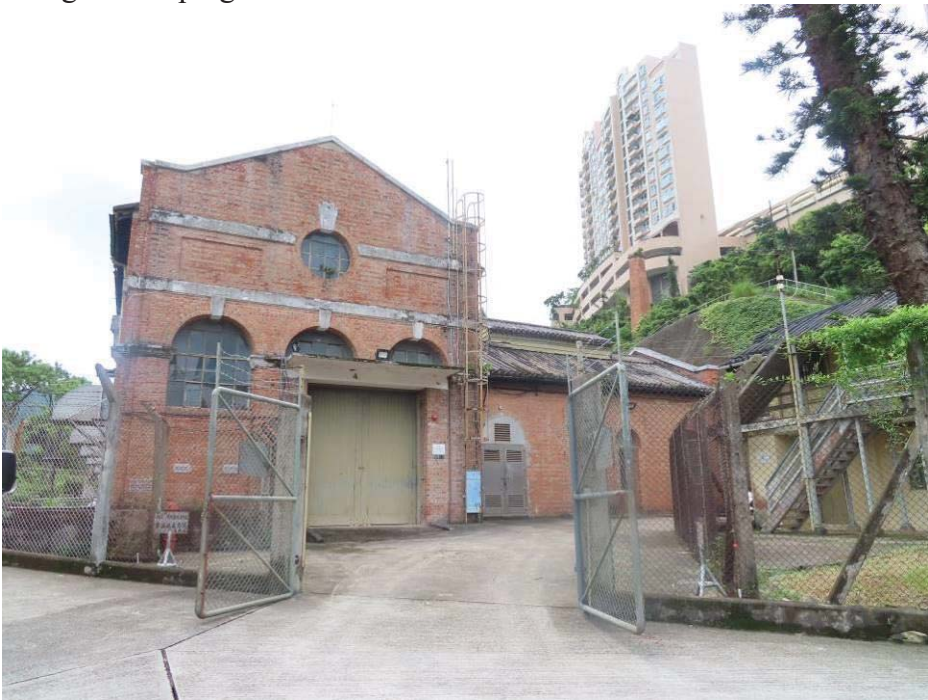
13.1 View of Pumping Station
