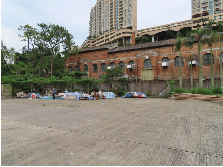
9.3 View of Yard
