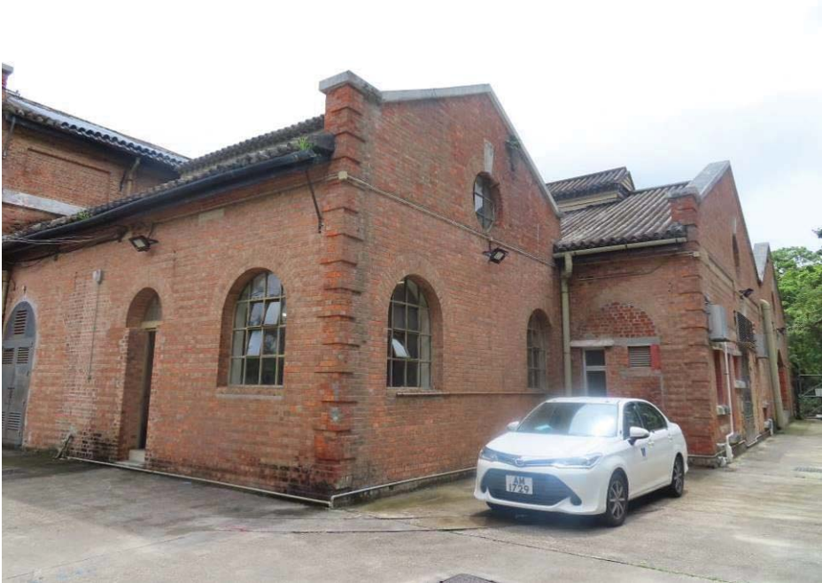
13.2 View of Pumping Station
