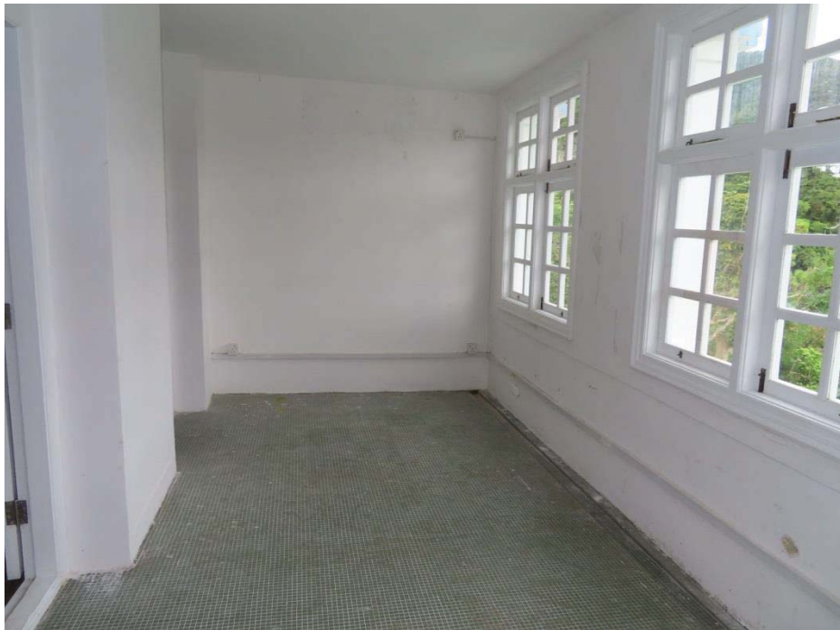
2.4 View of 1/F Hallway 4
