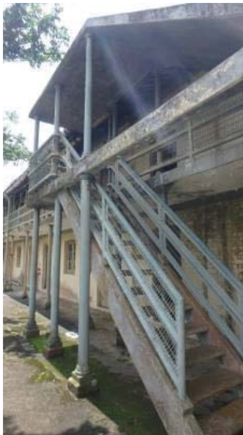
Open staircase on the west end
