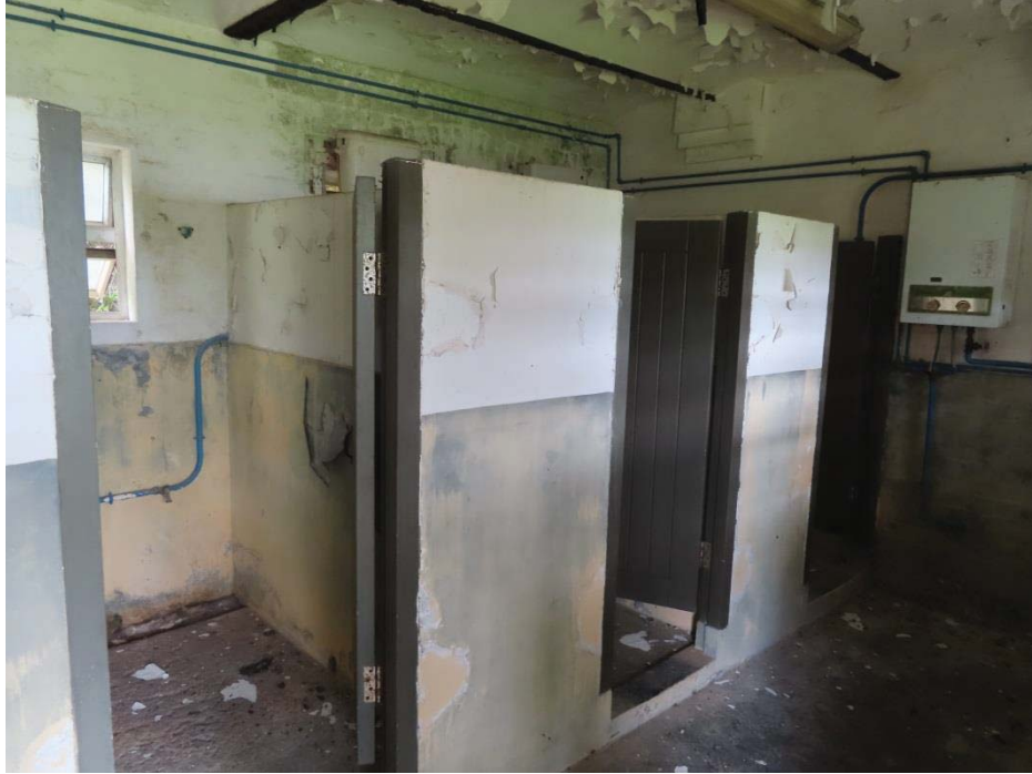
4.3 View of G/F Toilet 1
