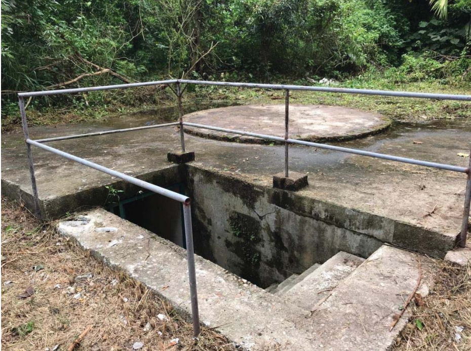
12.1 View of Entrance of Underground Cellar
