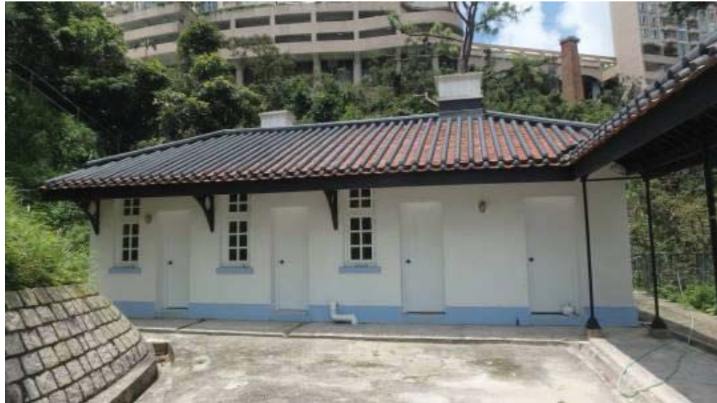
Hipped roof laid with double-layered pan and roll tiles
