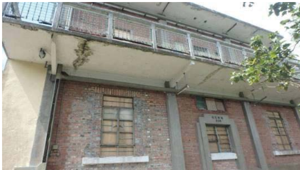
Open verandah at 1/F
