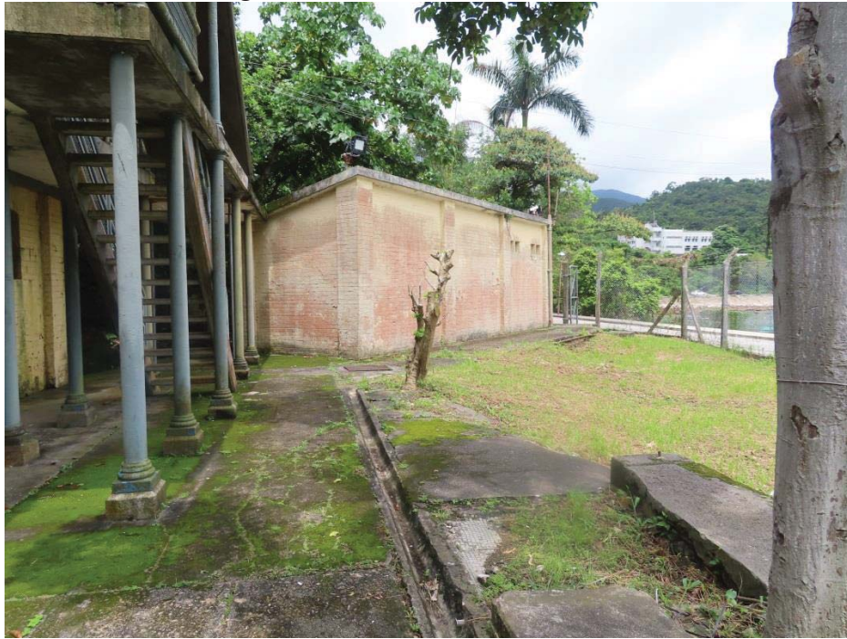
5.1 View of Store Building
