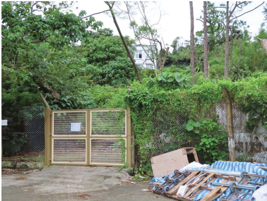
1.4 View of Interior Gate from Yard to Senior Staff Quarters (Main Building & Servant's Quarters)
