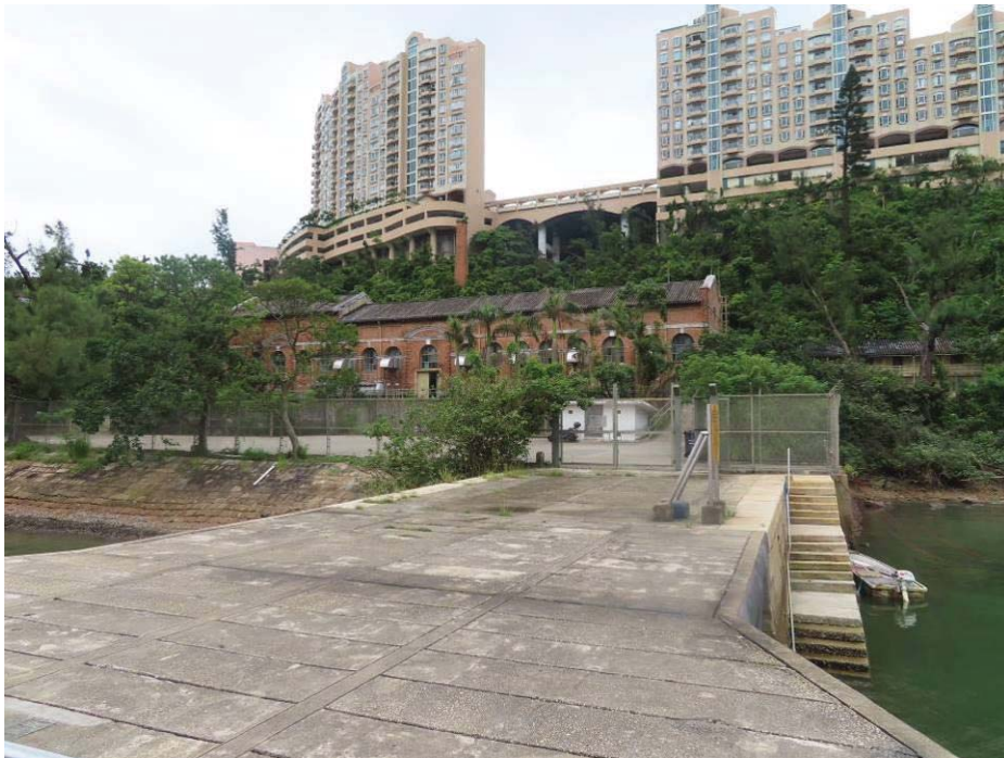
15.2 View of Tai Tam Bay Pier
