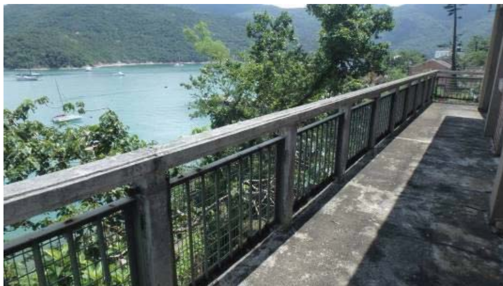
Metal balustrades with concrete railings and posts
