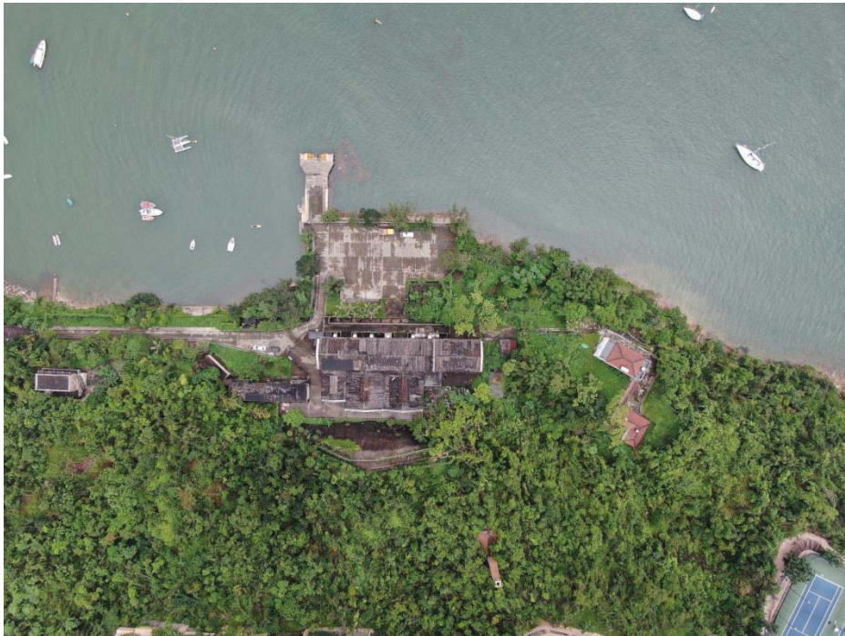
1.2 Aerial View of Tai Tam Tuk Raw Water Pumping Station Staff Quarters Compound
