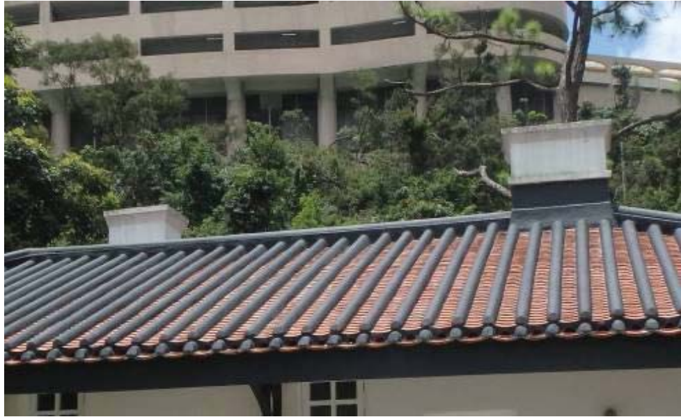
Chimney stacks at roof
