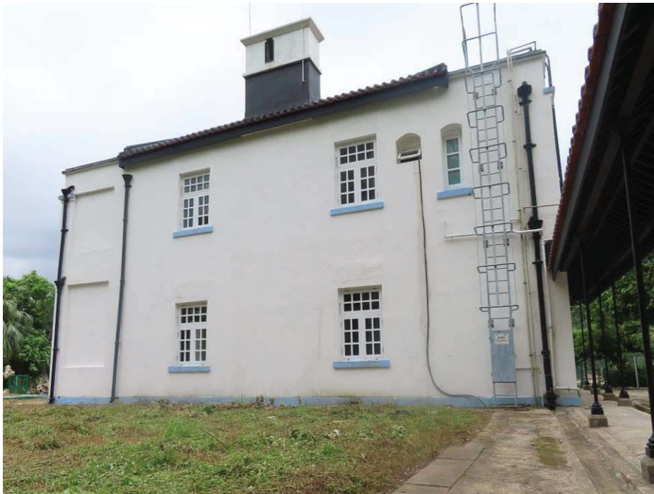
2.2 View of Senior Staff Quarters – Main Building
