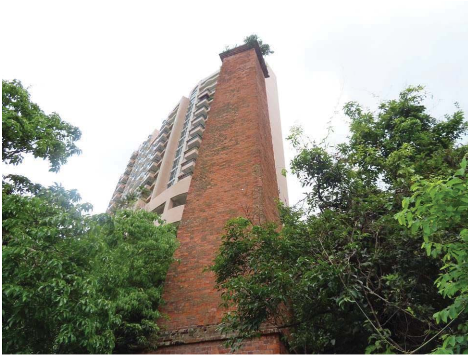
14.1 View of Chimney Shaft
