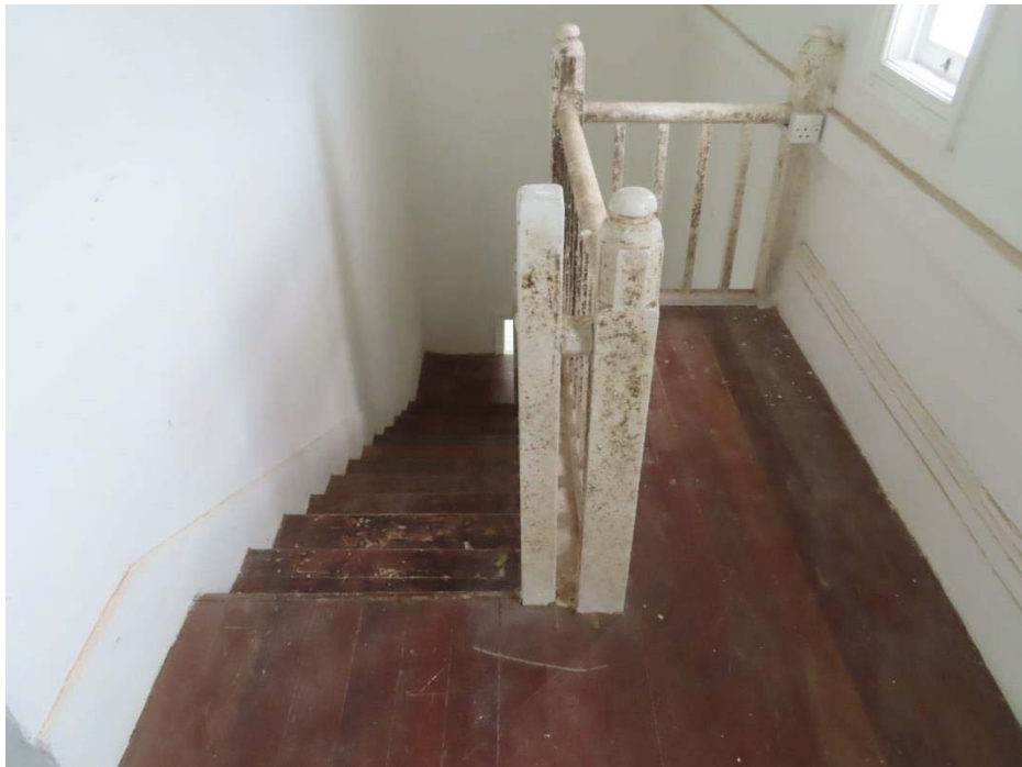
2.6 View of staircase
