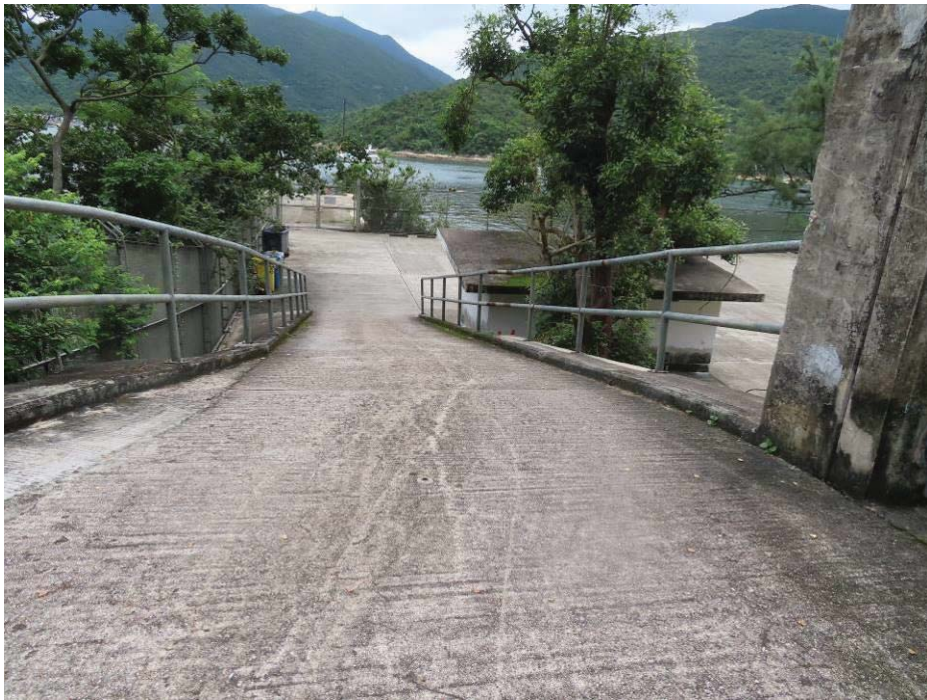
1.6 View of ramp from Tai Tam Reservoir Road to Yard
