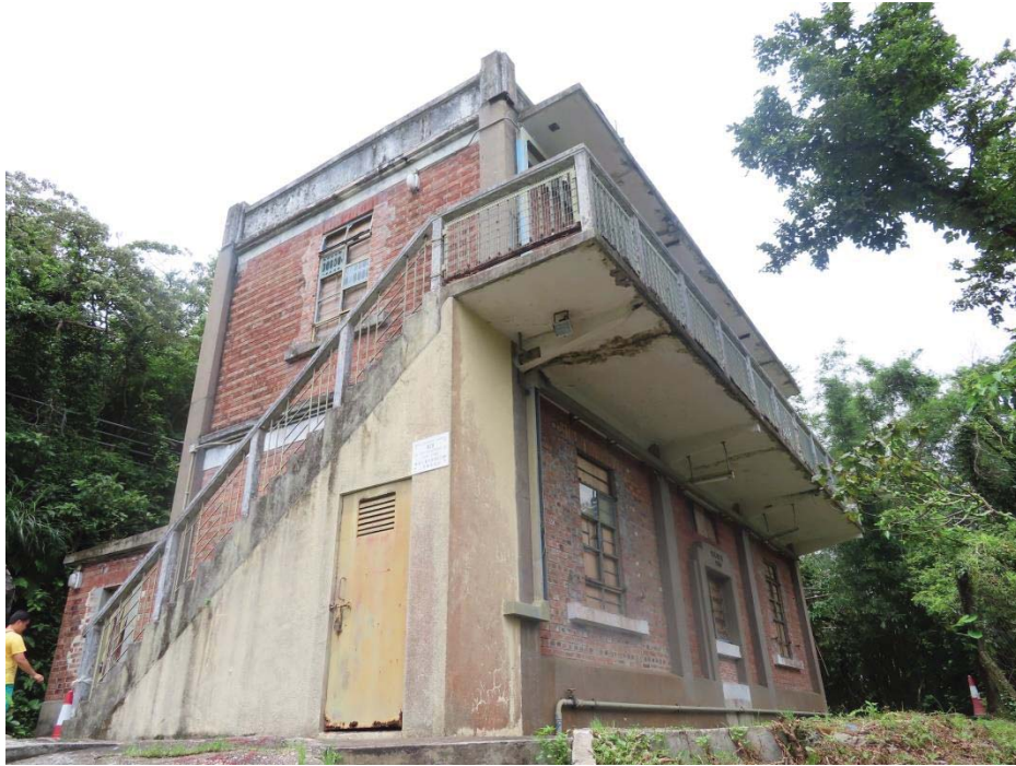
6.1 View of No. 2 Staff Quarters
