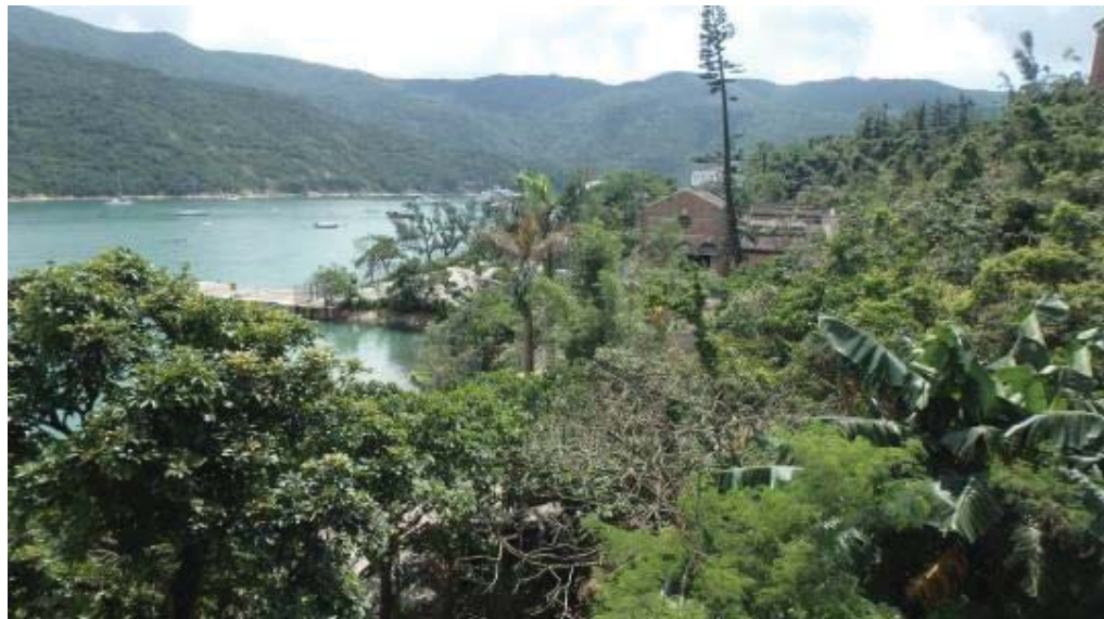
Vistas to the Pumping Station
