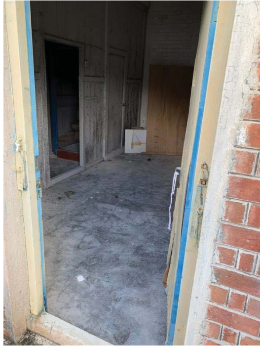
6.3 View of 1/F Room 5
