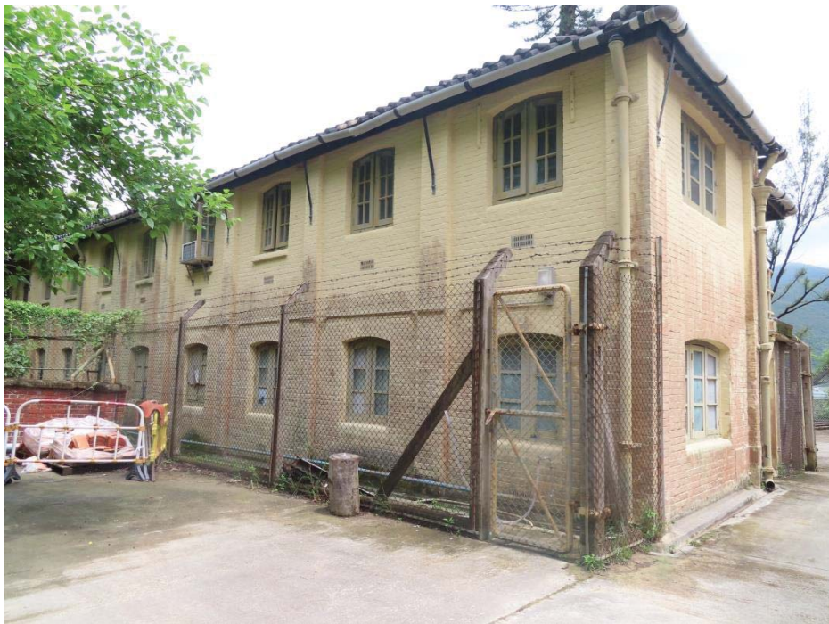
4.2 View of Staff Quarters - Main Building
