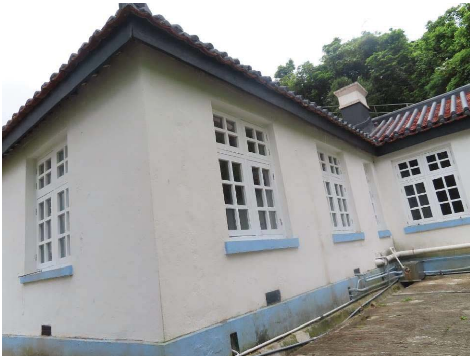
3.2 View of Senior Staff Quarters - Servants' Quarters
