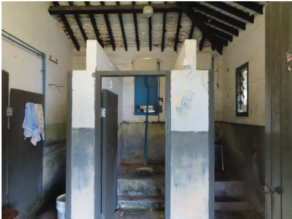
4.8 View of 1/F Toilet 2
