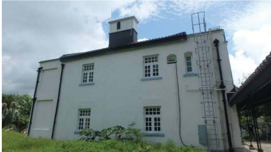
Hipped roof at the central and flat roofs at two sides
