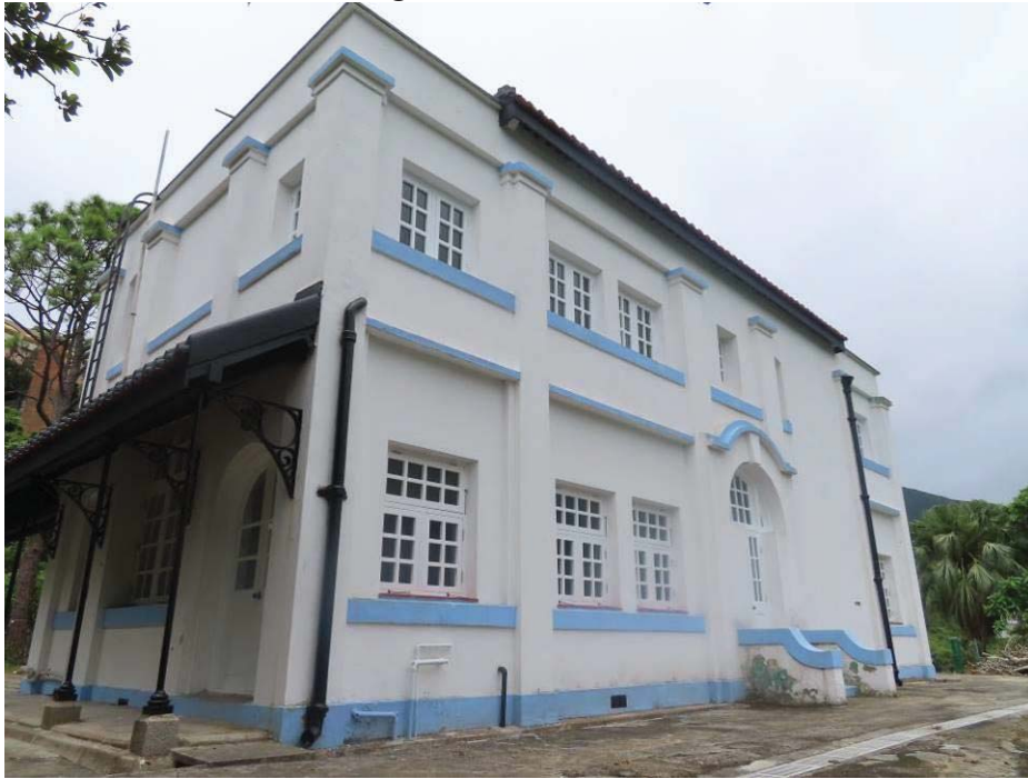
2.1 View of Senior Staff Quarters – Main Building
