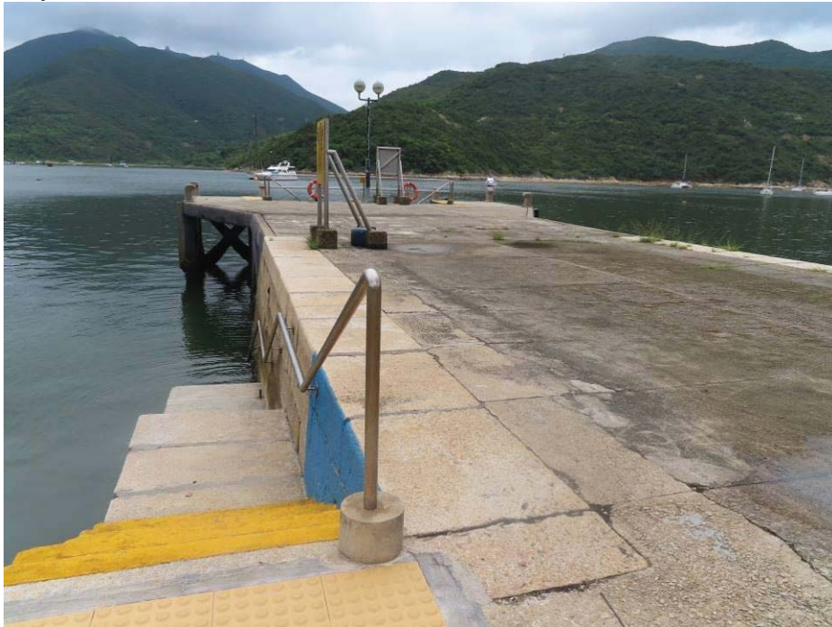
15.1 View of Tai Tam Bay Pier
