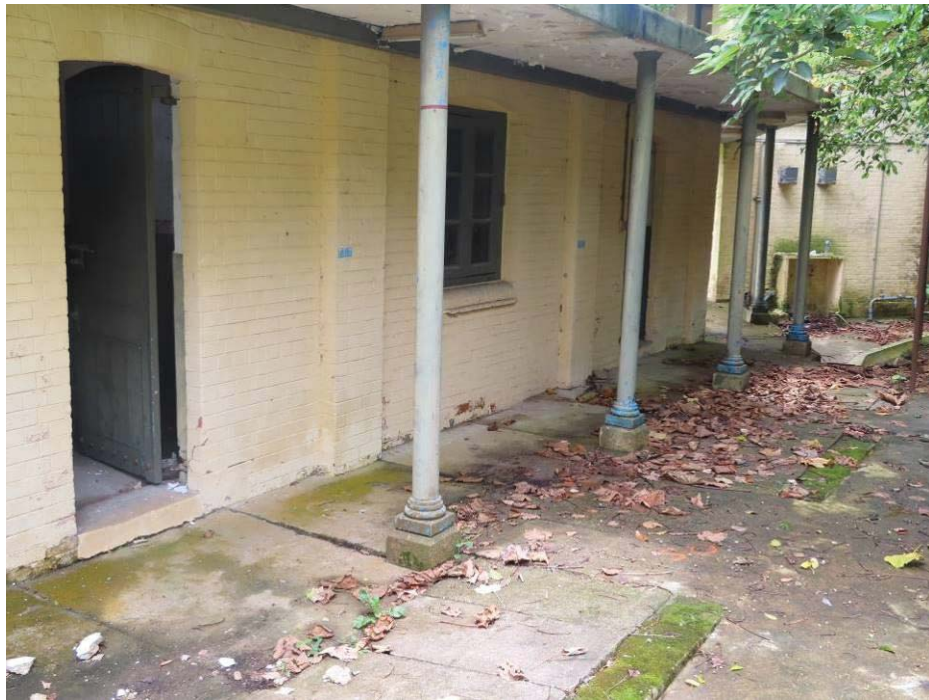
5.2 View of Store Building
