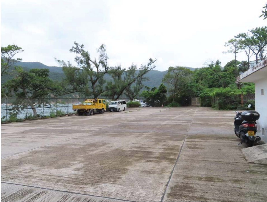
9.1 View of Yard
