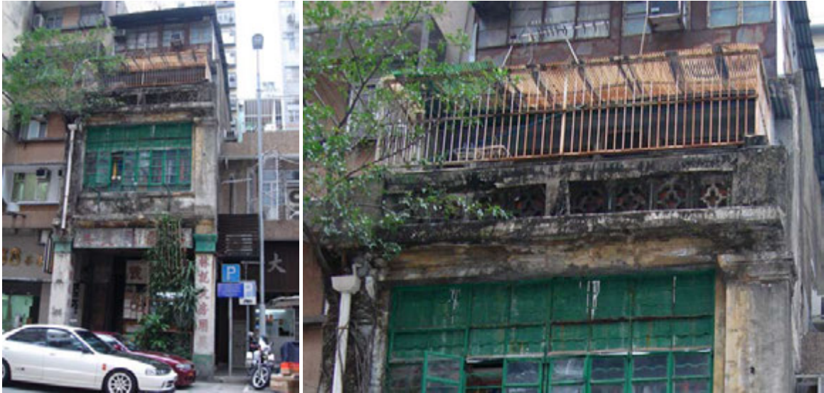
Fig. 292. Parapet with ventilation grilles and column highlighted with classical capitals at No. 65 Ha Heung Road.
