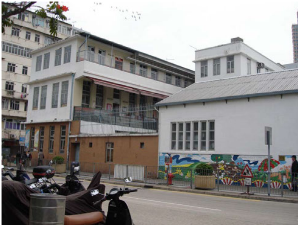
Fig. 220. Overview of Lok Sin Tong Primary School.
