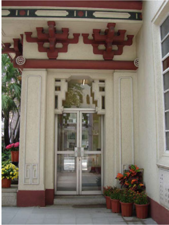
Fig. 141. The entrance porch of the Holy Trinity Church.
