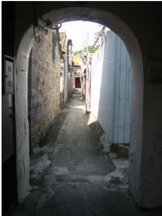
Fig. 187. Semi-circular archway viewing towards the central lane.
