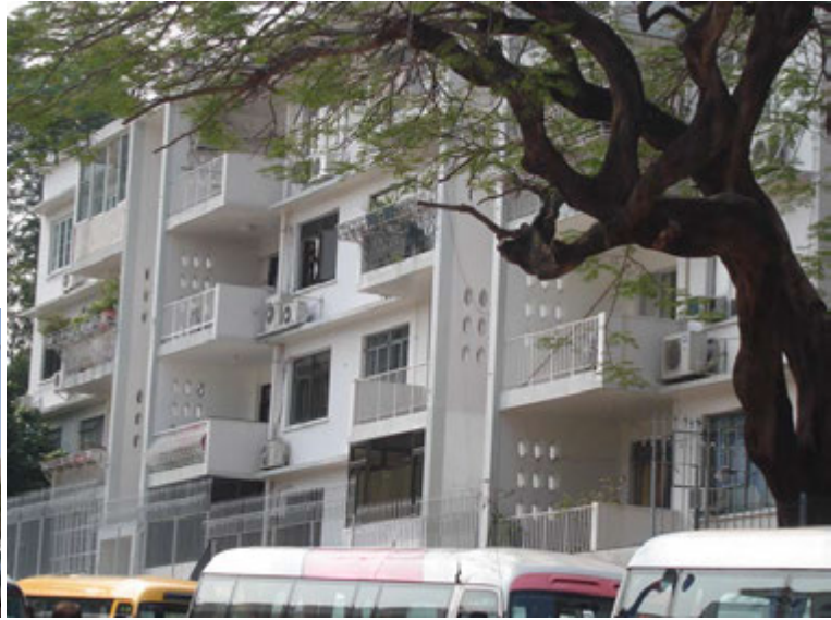
Fig. 249. Walls with vent holes providing sun-shading and ventilation to the balconies at Nos. 16-22 Dumbarton Road.
