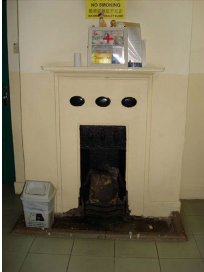
Fig. 69. Fireplace at the 2-storey block.
