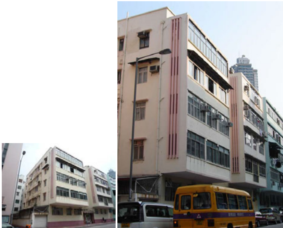
Fig. 168. Cantilevered balconies with balcony walls featured with ventilation grilles at Nos. 12-34 Shing Tak Street.
