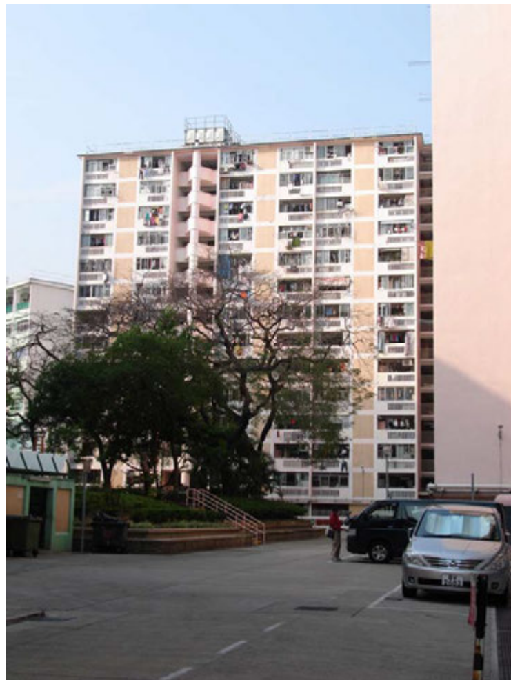
Fig. 158. Exterior view of Ma Tau Wai Estate 馬頭圍邨, 2009.
