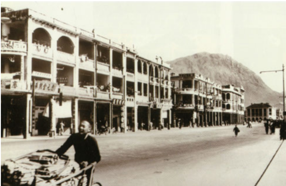
Fig. 21. Tenement houses along Prince Edward Road West. Building located at the end of the road, is likely to be the Kowloon City Police Station, c. 1939. (from Lau Yun Wo 劉潤和, Jiulongchengqu fengwuzhi 九龍城區風物志 [A Guide to the Antiquities of Kowloon City District], 2005, p. 130.)
