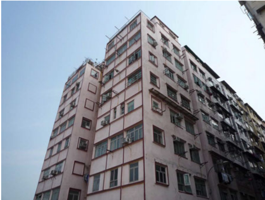
Fig. 97. Residential block at Hing Yan Street.
