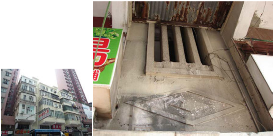
Fig. 290. Rhombus motif at the staircore of Nos. 162-168 Pau Chung Street.
