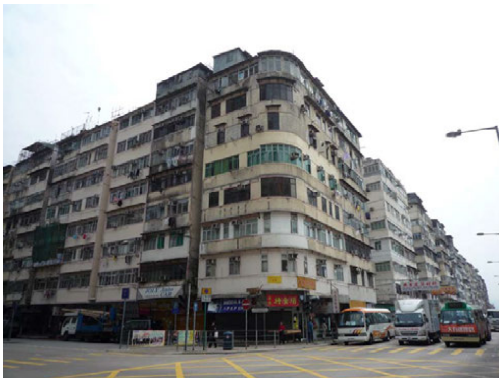
Fig. 81. The residential blocks in 13 streets, 2009.
