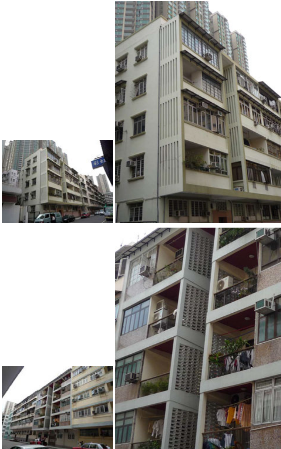
Fig. 287. Walls with vent holes providing sun-shading and ventilation to the balconies at Nos. 38-44 (above) and 106-108 (below) Maidstone Road.
