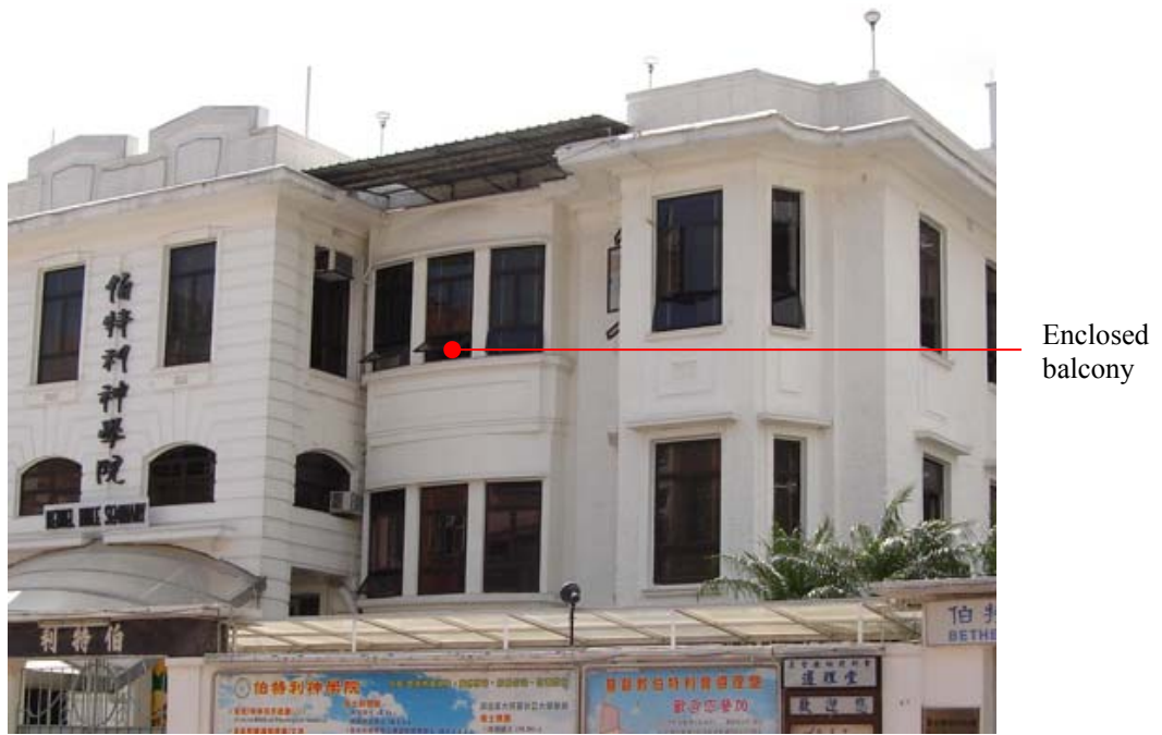
Fig. 226. Original balconies at the front elevation which are now enclosed.
