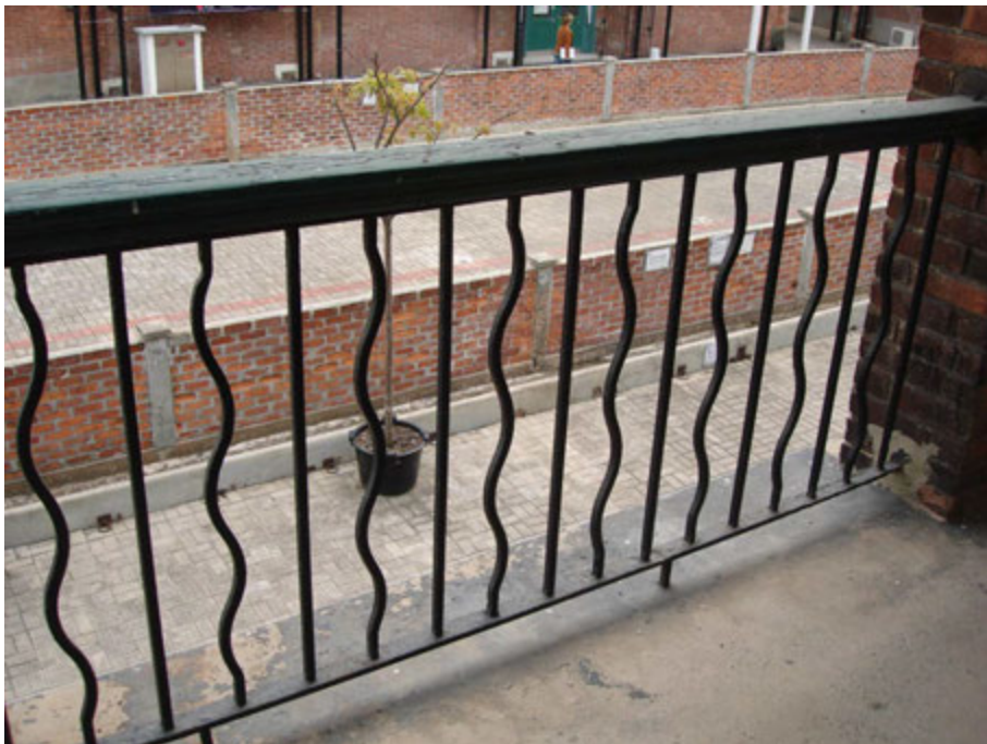
Fig. 70. Ironwork at the balustrade of the 2-storey block.
