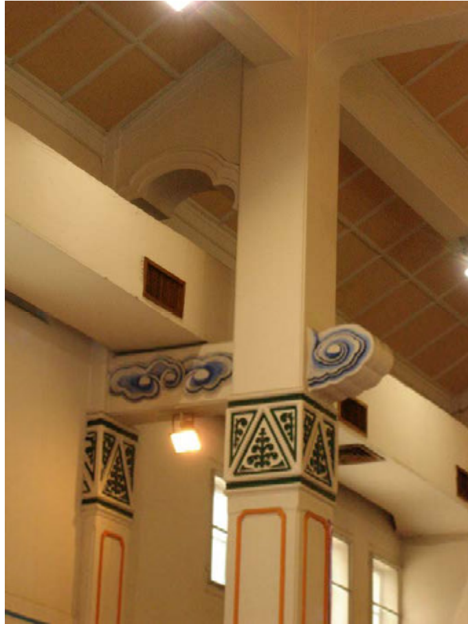
Fig. 143. Cloud-head decoration at the beam of the aisles inside the Holy Trinity Church.
