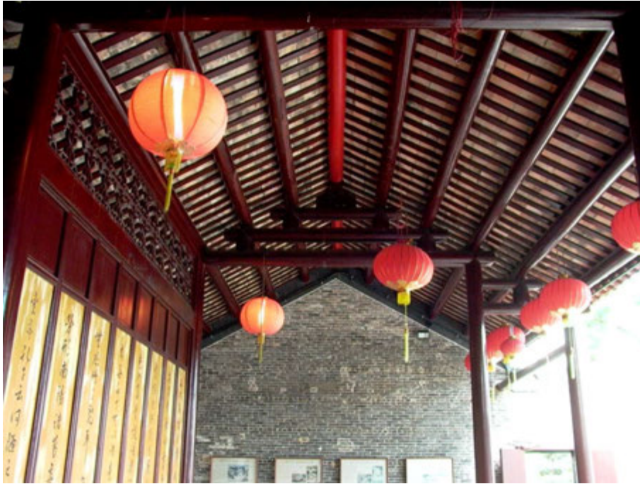
Fig. 201. The column-beams-and-struts system at the main hall.
