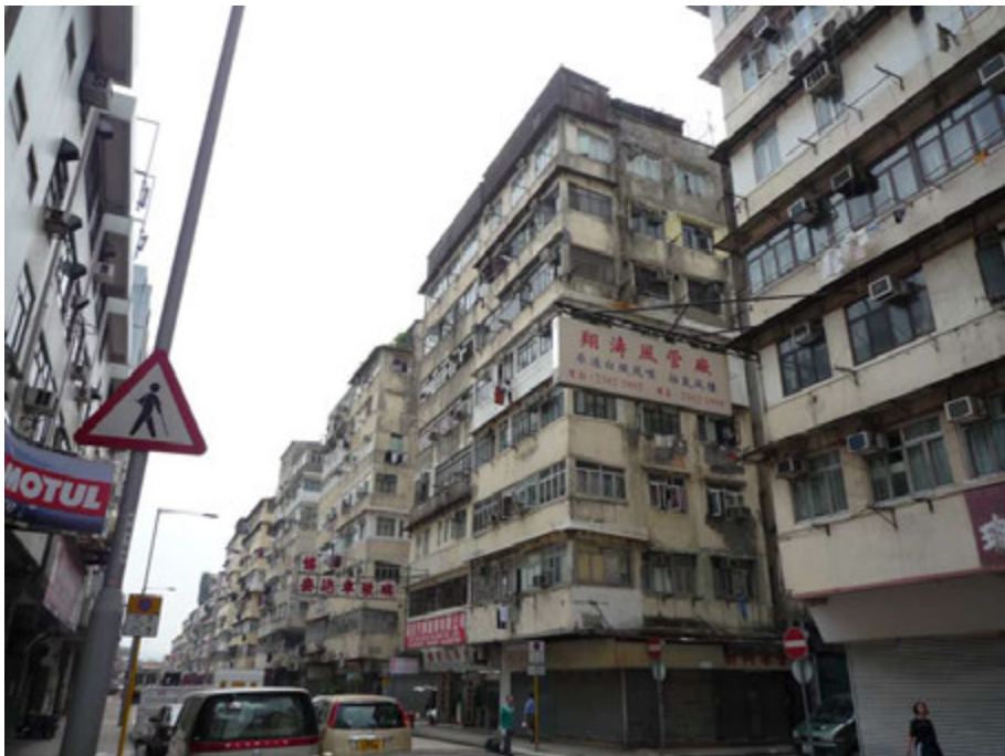
Fig. 84. View of the twelve residential blocks facing Mok Cheong Street.
