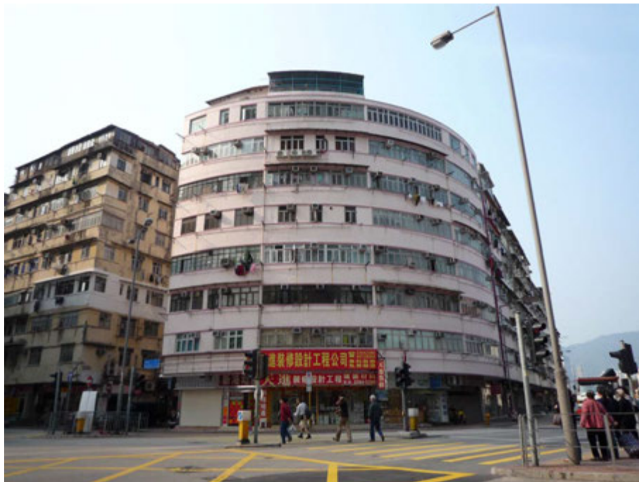
Fig. 86. View of the residential block (originally named block 'A').
