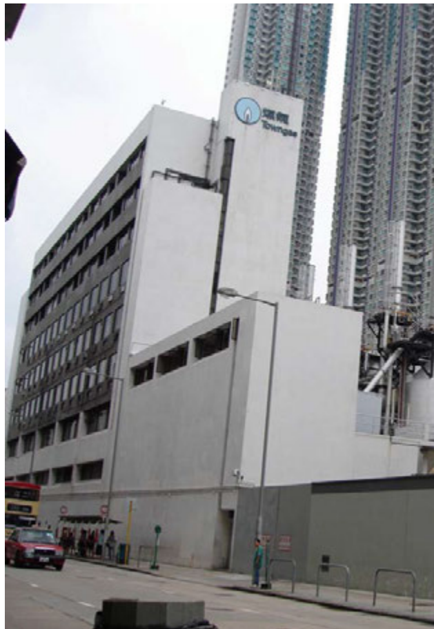
Fig. 76. Front view of the office building of the Mau Tau Kok Gas Plant.
