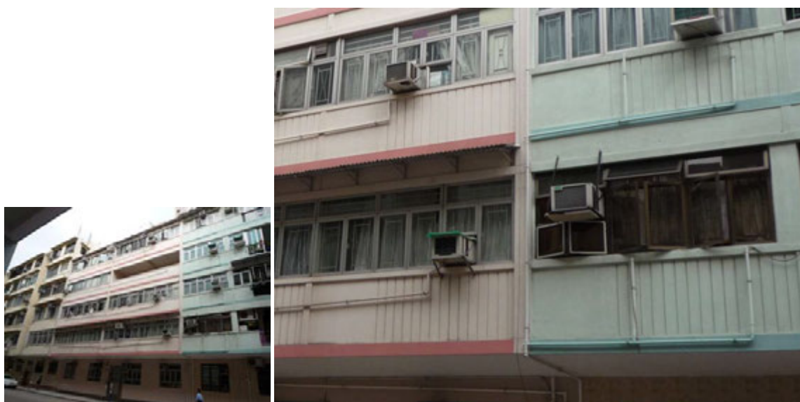
Fig. 286. Vertical banded mouldings at balconies of Nos. 107-109 Maidstone Road.
