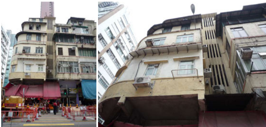
Fig. 121. Ventilation grilles at stair cores, enclosed cantilevered balconies and set-back upper storeys at Nos. 50-52 Ma Tau Kok Road.
