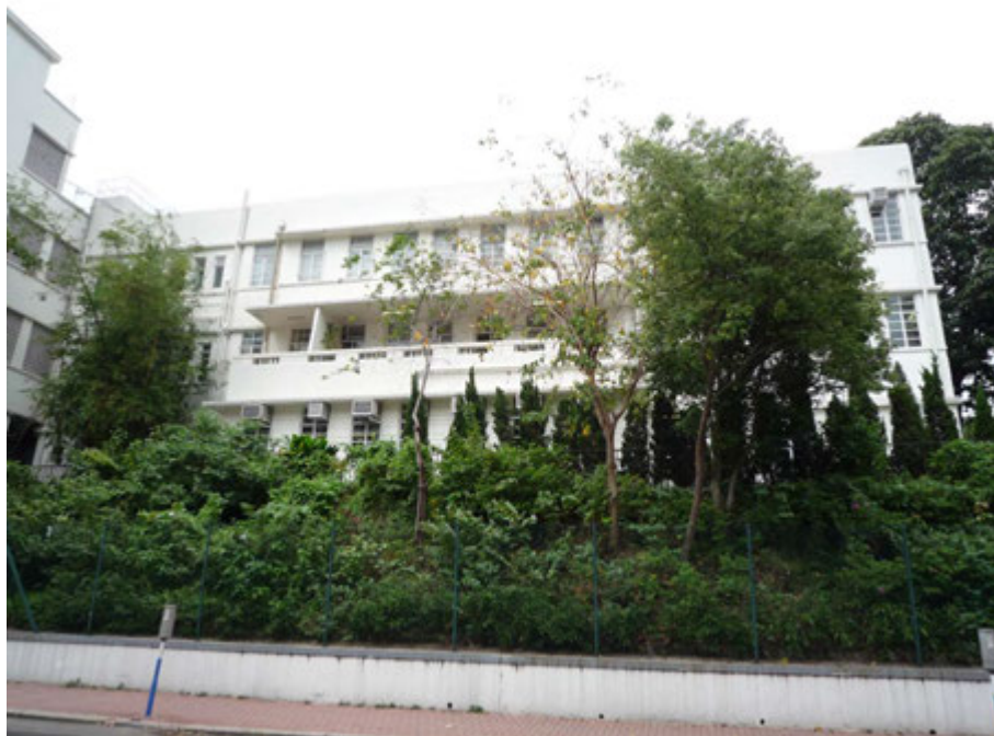
Fig. 263. Side elevation of the main building of Art Deco style facing Farm Road.
