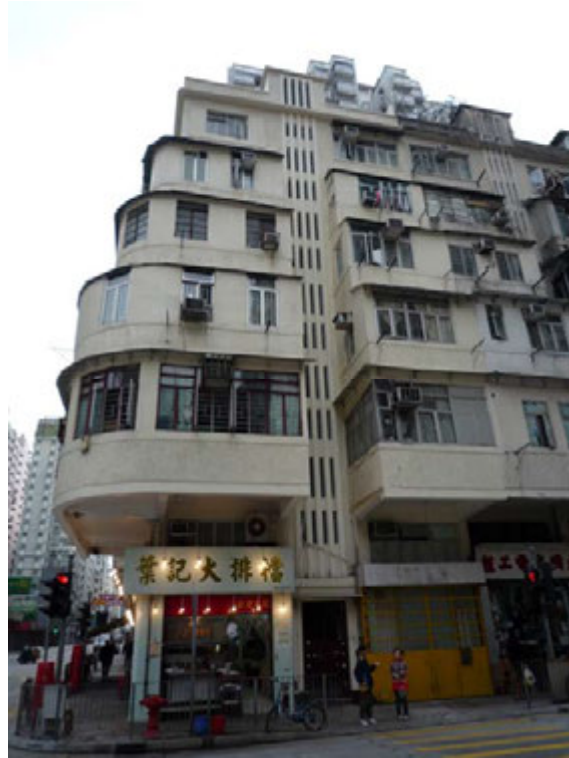
Fig. 169. Common staircase with ventilation grilles and set-back upper stories at Nos. 44-46 San Shan Road.
