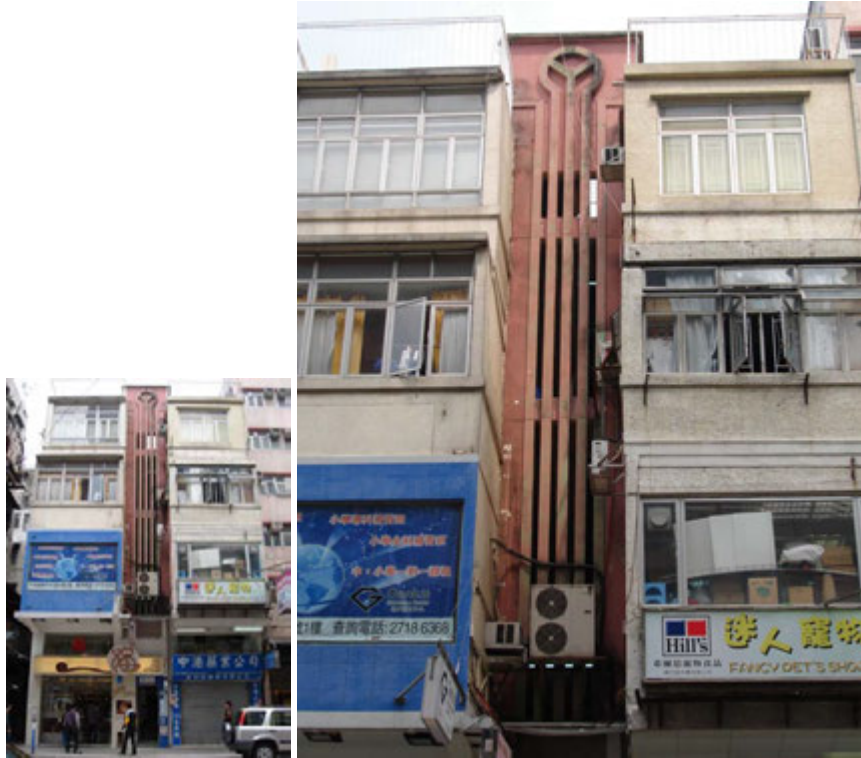
Fig. 252. Articulation at the staircore at No. 42-44 Lion Rock Road.
