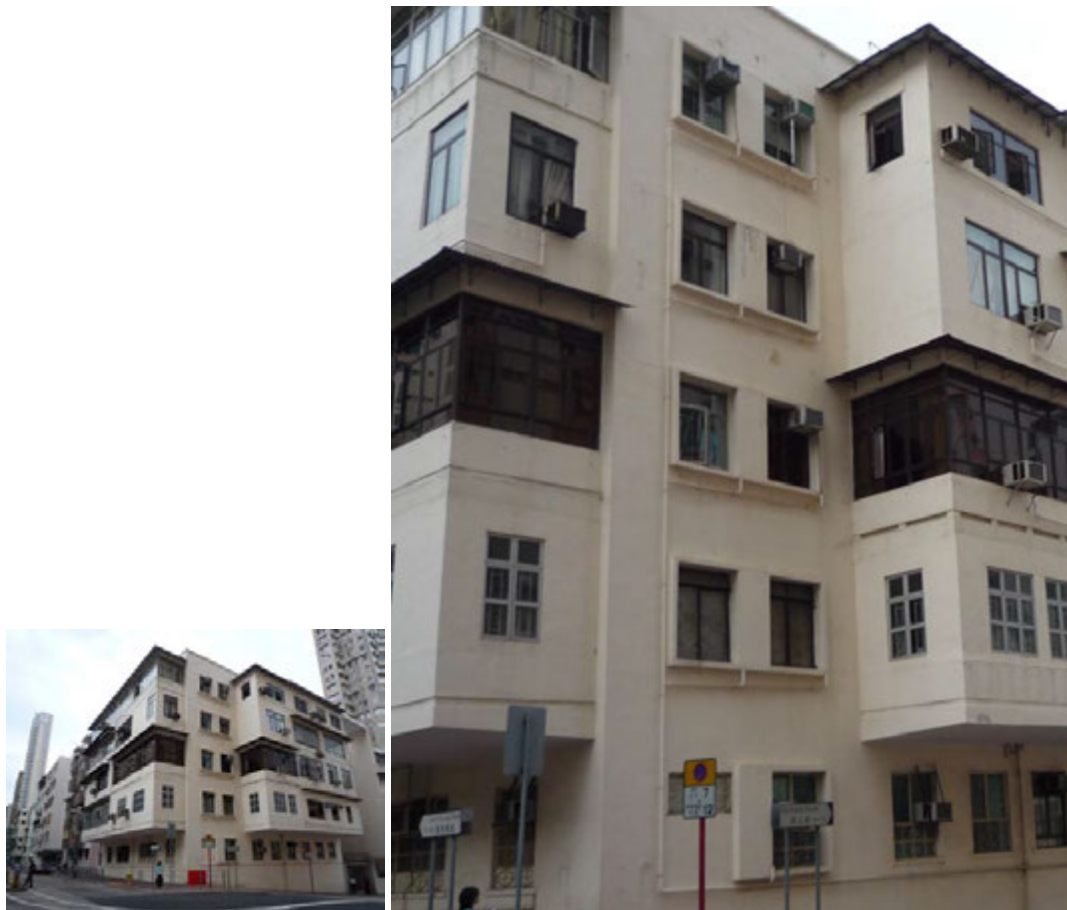
Fig. 285. Architrave surrounding the windows at Nos. 58-58A Chi Kiang Street.
