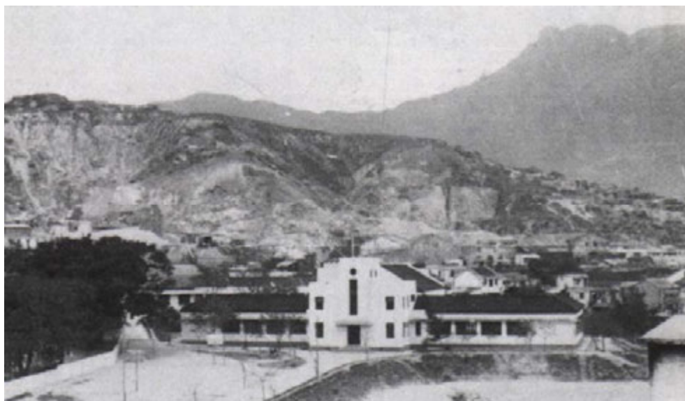
Fig. 235. New campus of Munsang College built in 8 Dumbarton Road 東寶庭道 in 1939. (from Fung Sze Man 馮思敏, Munsang College 75th anniversary, 1926-2001 , Hong Kong, Munsang College, 2001, p. 23.)
