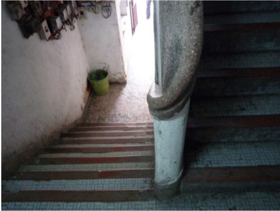
Fig. 91. Staircase at the residential block at the 13 streets.
