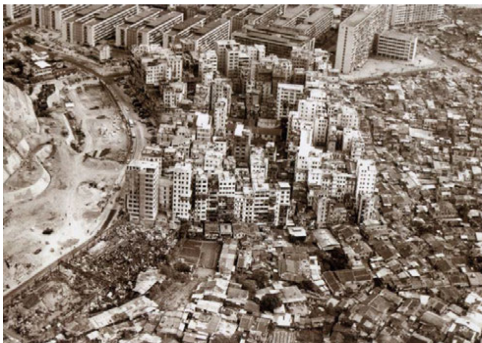
Fig. 198. Tenement houses were built in the Kowloon Walled City, 1972. (from Lau Yun Wo 劉潤和, Jiulongchengqu fengwuzhi 九龍城區風物志 [A Guide to the Antiquities of Kowloon City District], 2005, p. 43.)
