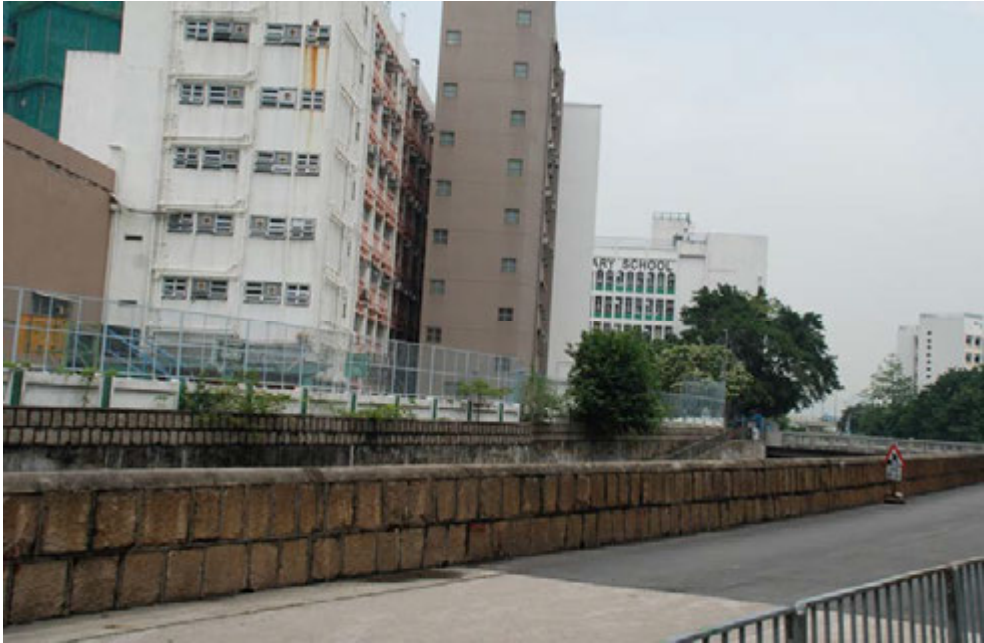
Fig. 300. The masonry parapet of the nullah was constructed by the boulders from the Kowloon Walled City, 2009.
