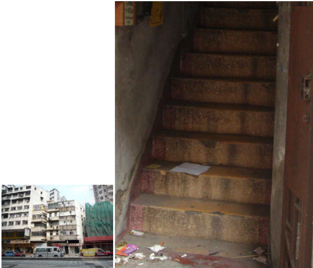
Fig. 291. Concrete staircase finished with terrazzo at Nos. 191-195 Ma Tau Wai Road.
