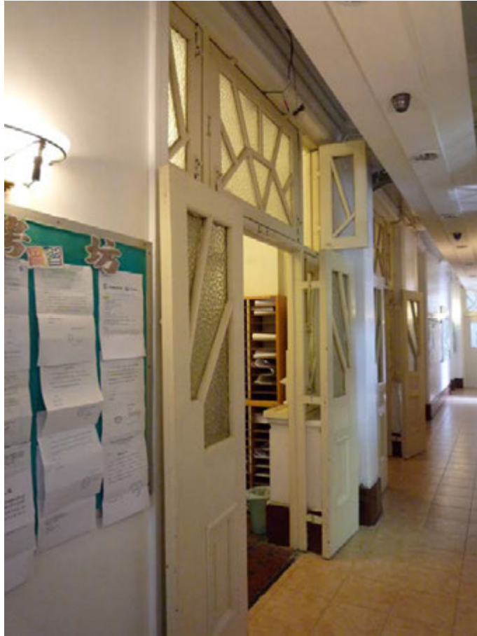
Fig. 230. Original timber doors with sunray motif.
