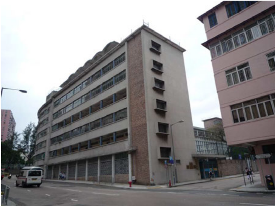
Fig. 278. Front view of block B at Tin Kwong Road.
