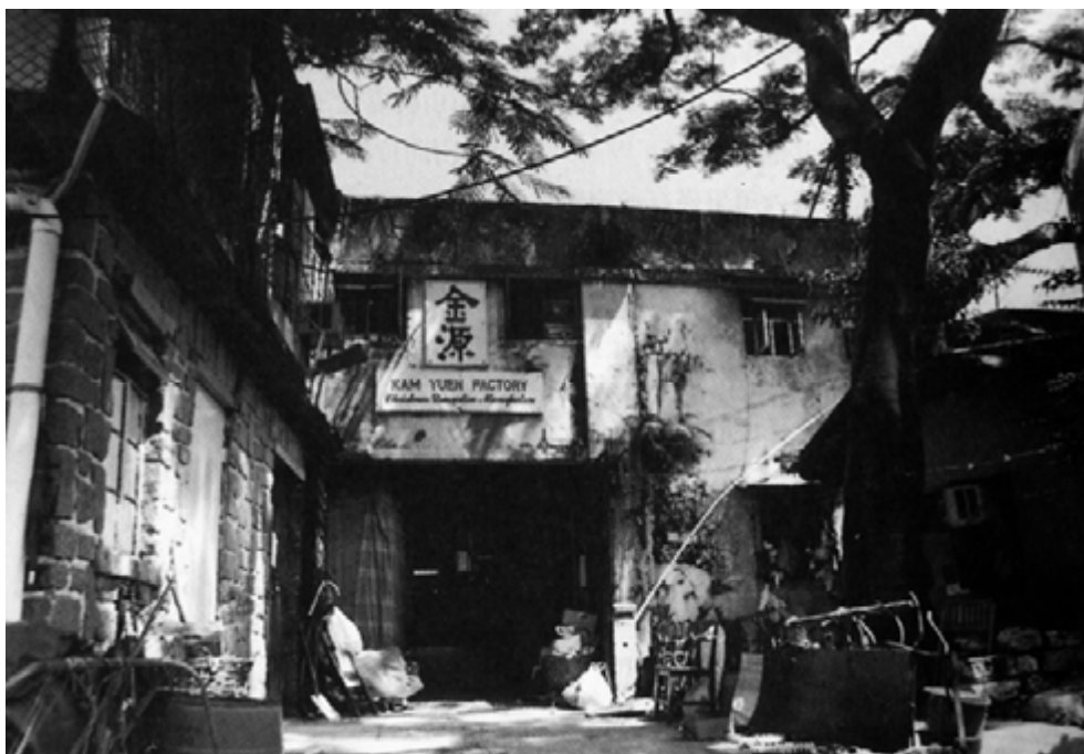
Fig. 242. The building of former Cheung Shing Movie Enterprise Ltd 長城電影公司在 Hau Wong Temple New Village subsequently converted into Kam Yuen Factory. (from Chiu Yu Lok 趙雨樂, Chung Po Yin 鍾寶賢, Regional Study of Hong Kong History: Kowloon City, Hong Kong , Joint Publishing (H.K.) Company Limited, 2001, p. 226.)
