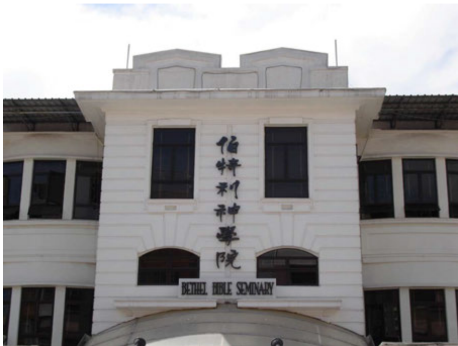
Fig. 229. Stylized gables, segmental arched windows and the banded rustication on the front elevation of Bethel Bible Seminary.
