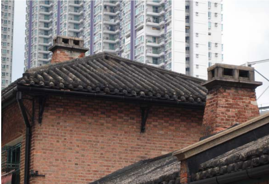
Fig. 67. Tapered chimneys, brackets, and Chinese pan and roll tiled roofs of the row building at the front.
