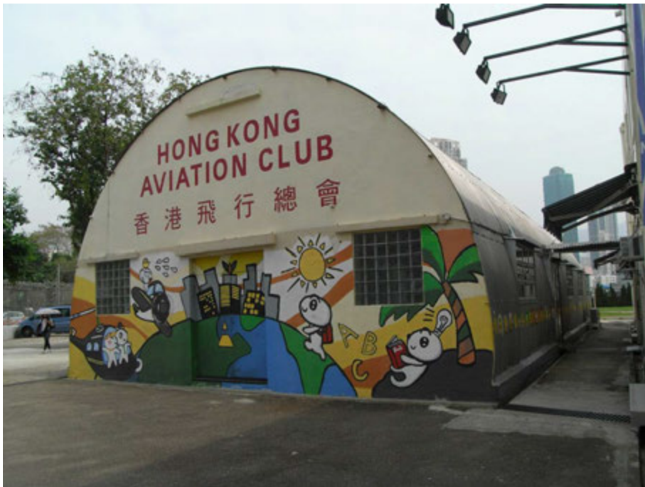
Fig. 148. External view of the Nissen Hut facing Sung Wong Toi Road.
