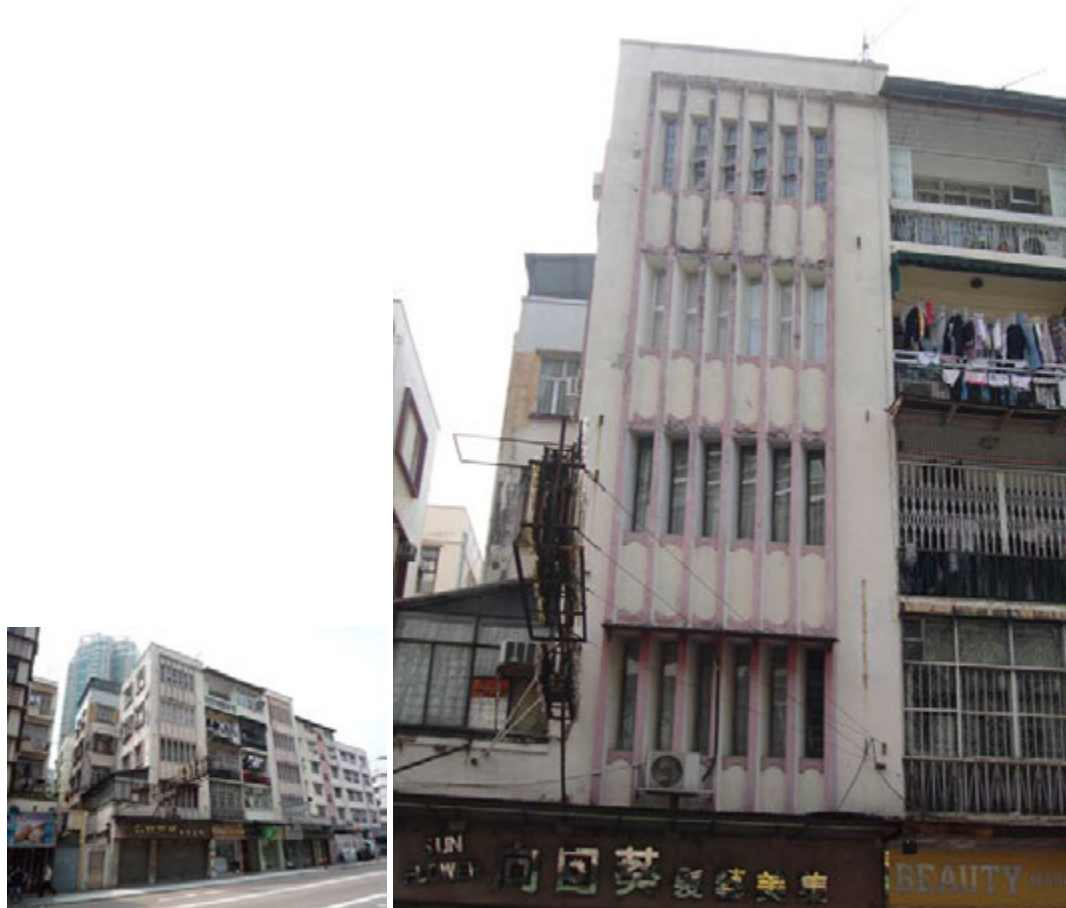
Fig. 248. Deep vertical fins beside windows at Nos. 7-7C Junction Road.
