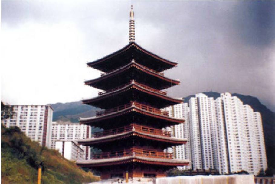
Fig. 323. Pagoda of Ten Thousand Buddha. (from Xianggang Zhi lian jing yuan fang Tang jianzhu yingzao 香港志蓮淨苑仿唐建築營造 [Hong Kong Chi Lin Nunnery modeled after Tang dynasty architecture construction], 1999, p. 19.)
