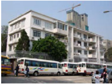
Fig. 249. Walls with vent holes providing sun-shading and ventilation to the balconies at Nos. 16-22 Dumbarton Road.
