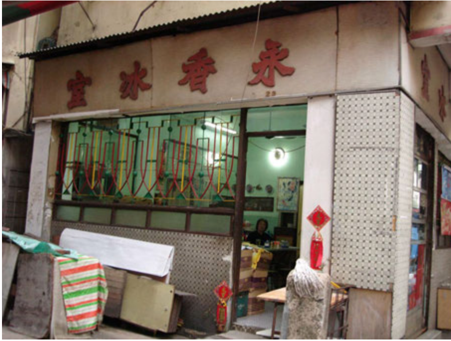
Fig. 331. Side view of No. 29 Wing Yiu Street.
