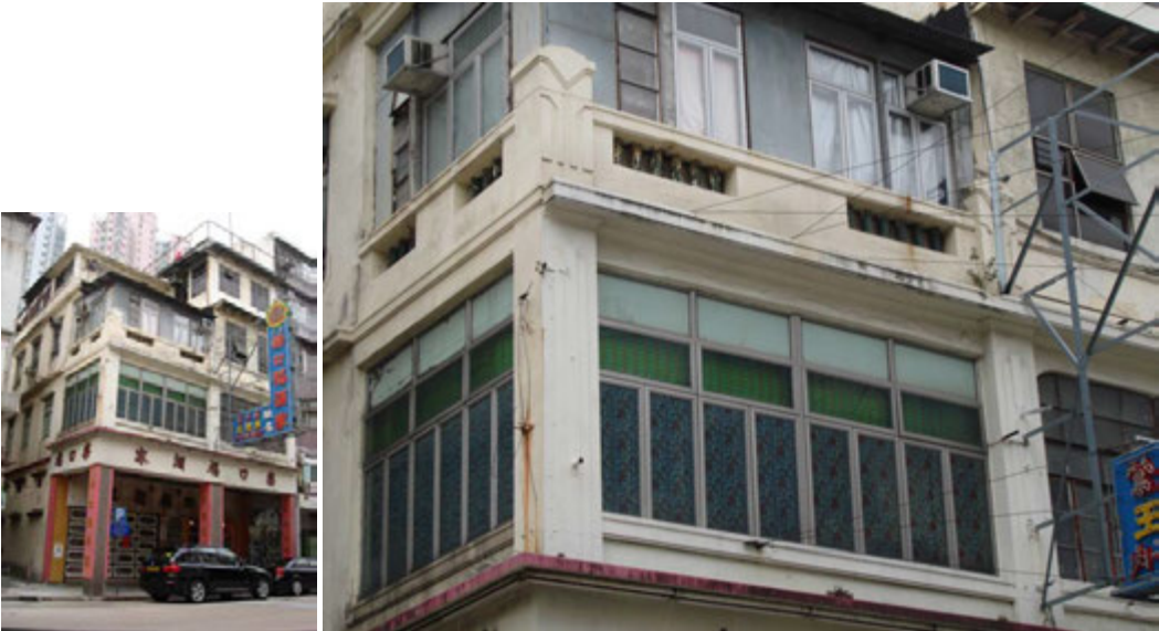
Fig. 257. Bamboo-shaped balusters and column capitals sculpted with art deco pattern at Nos. 1-3 Hau Wong Road.
