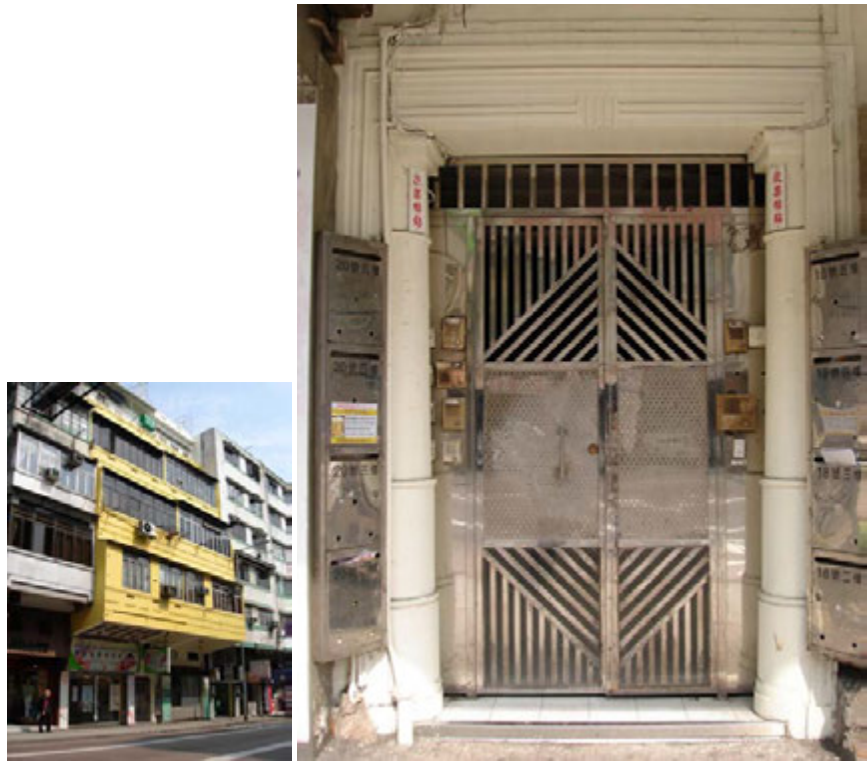
Fig. 254. Classical columns and moulded door surround at Nos. 18-20 Junction Road.
