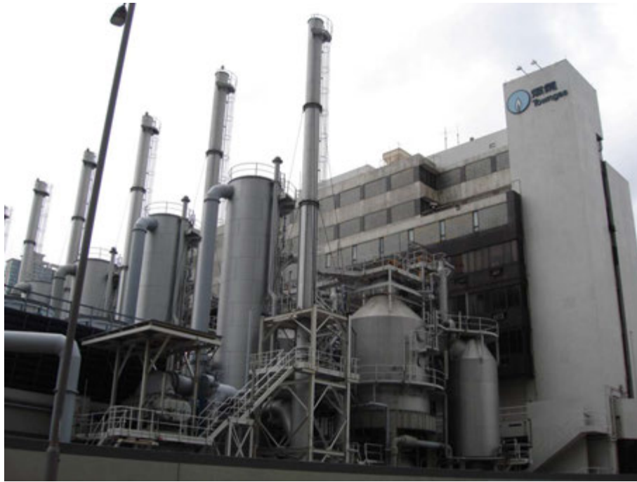
Fig. 77. The rear view of the office building of the Ma Tau Kok Gas Plant.
