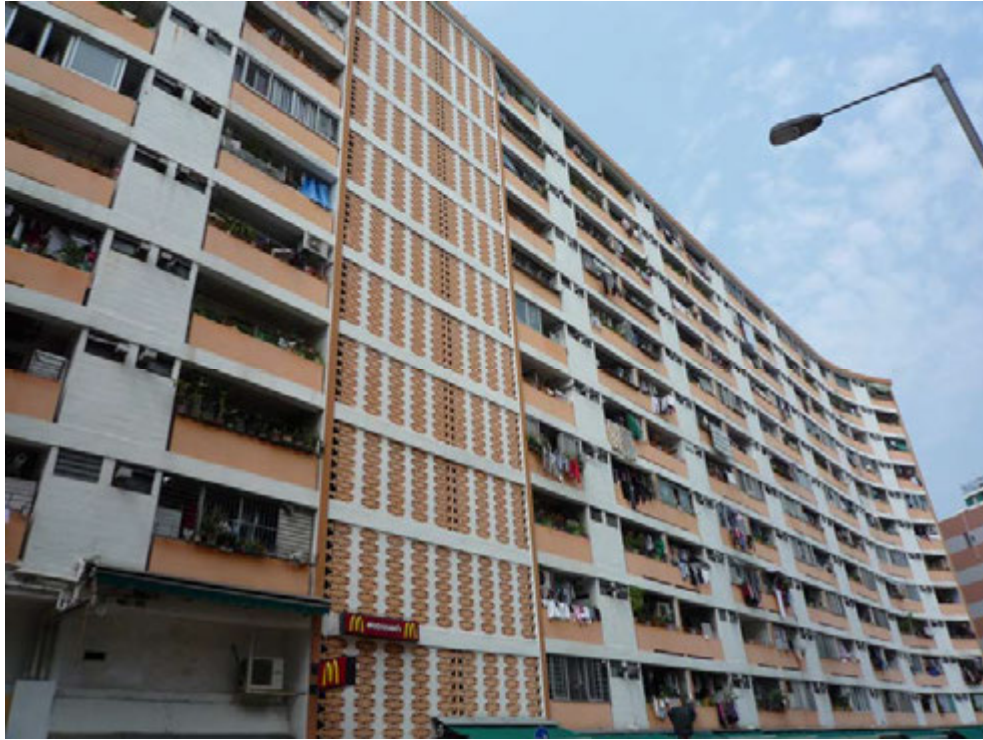
Fig. 159. Exterior view of Chun Seen Mei Chuen, 2009.
