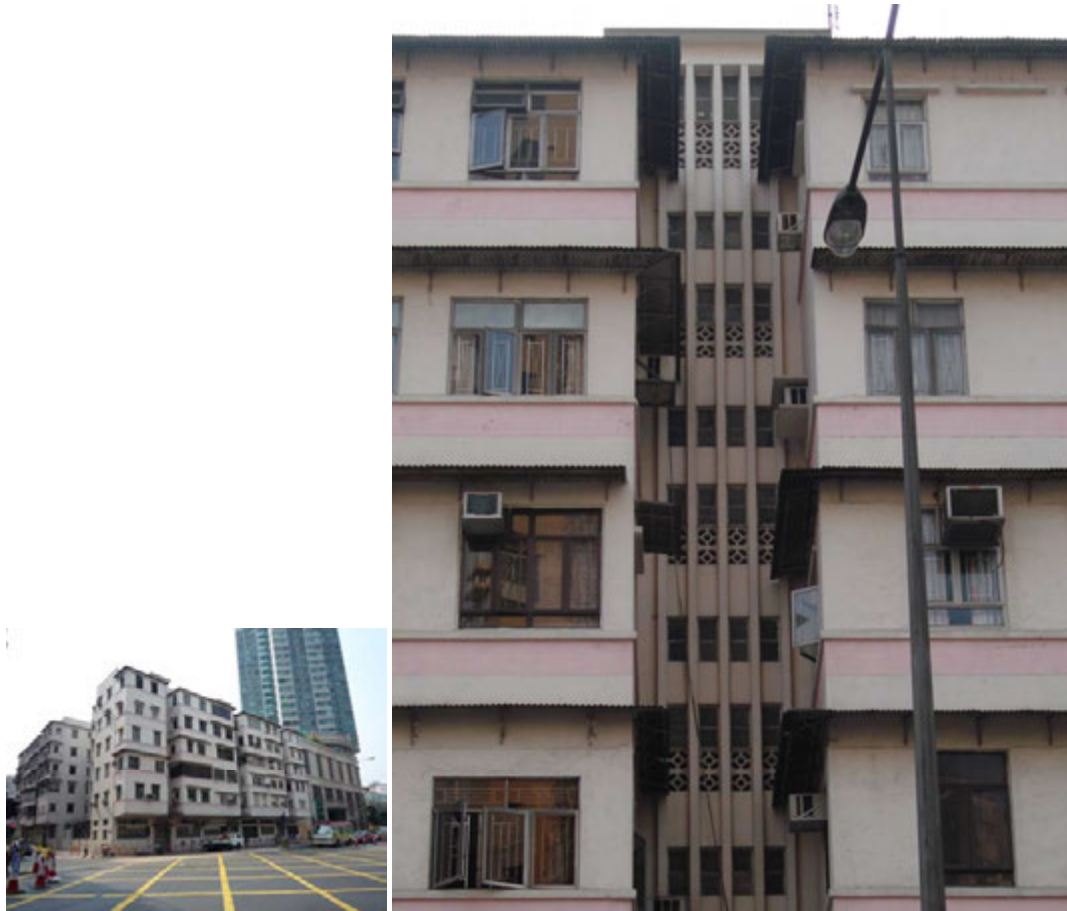
Fig. 288. Staircore on the main elevation at Nos. 452-462 Ma Tau Wai Road.
