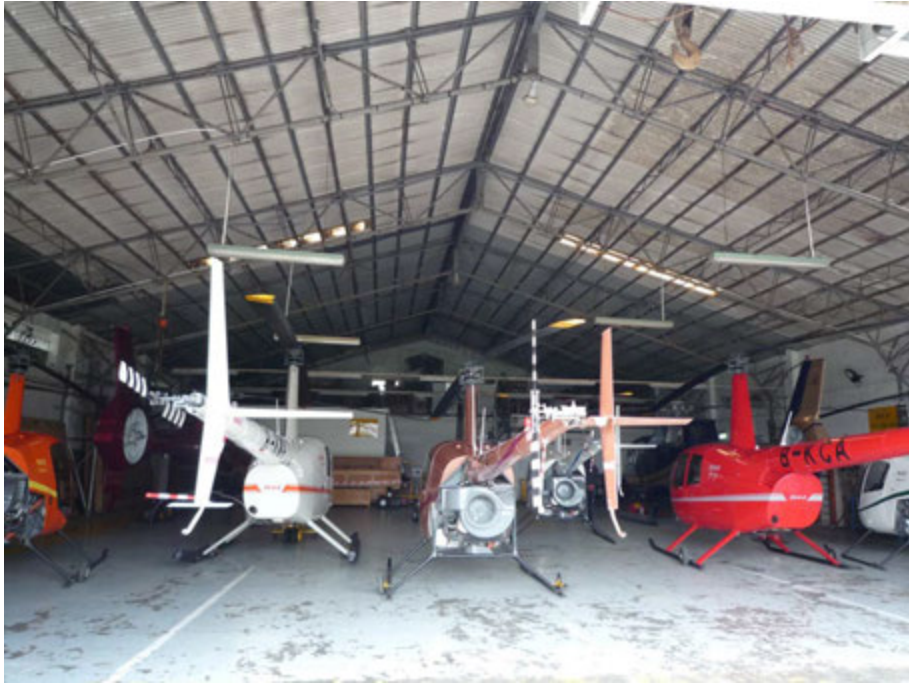
Fig. 151. Interior view of the Hanger.
