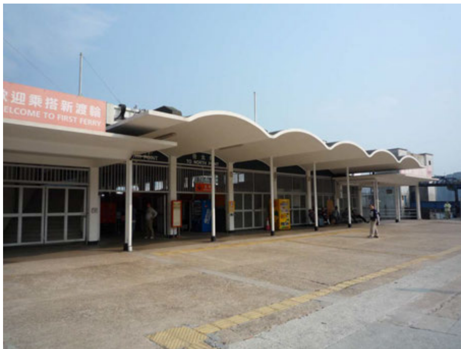
Fig. 110. The entrance canopy of the Kowloon City Ferry Pier.
