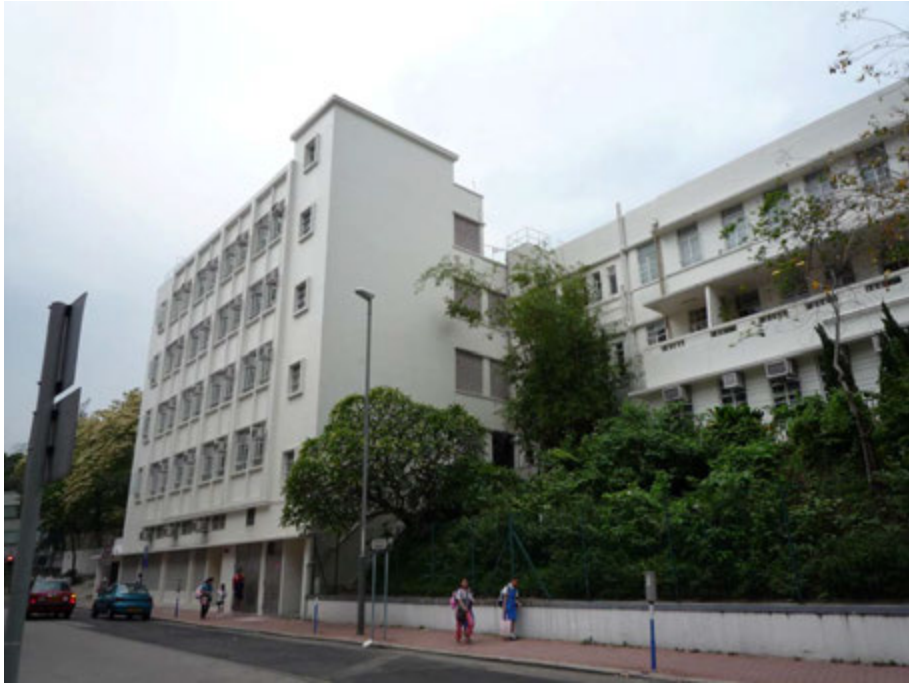
Fig. 264. Annex of modern style at the main building facing Farm Road.
