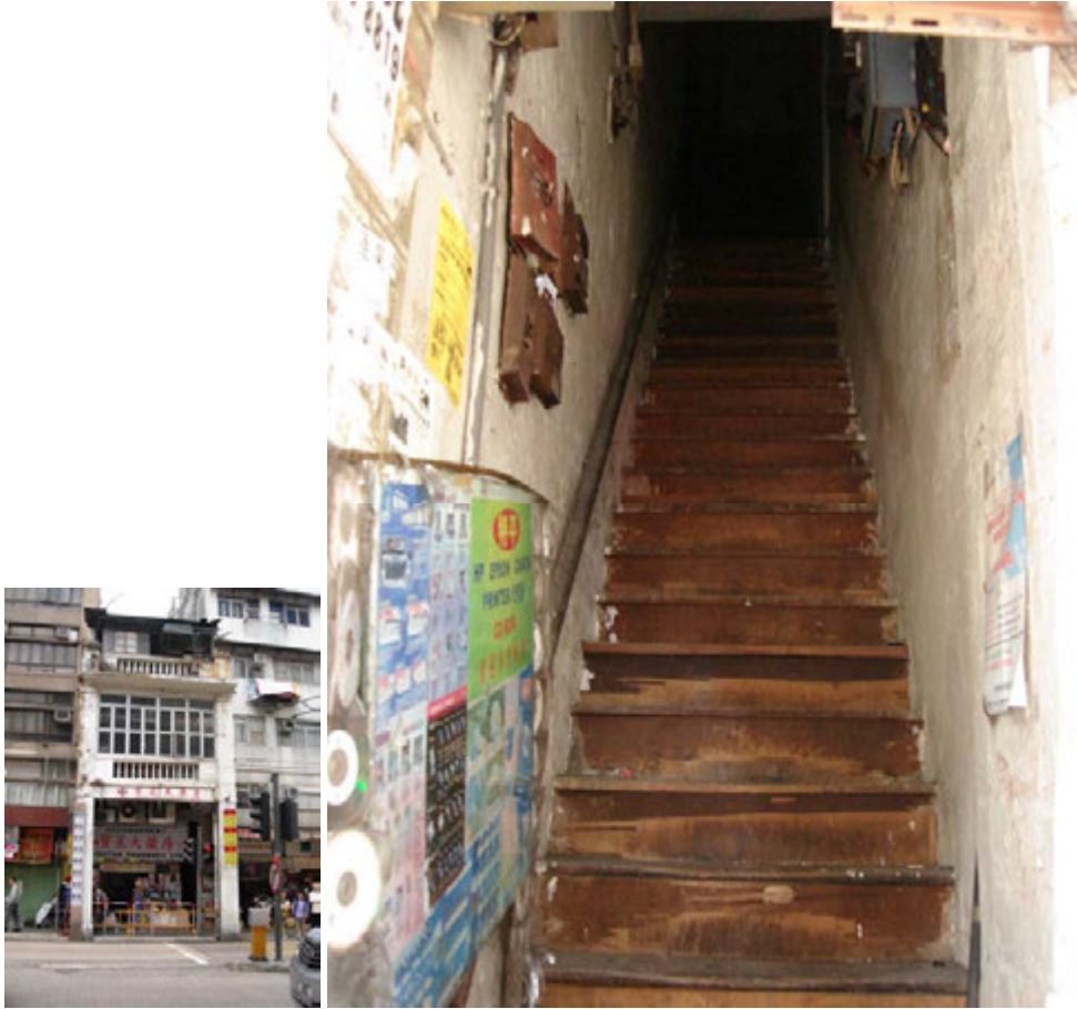
Fig. 258. Timber staircase at No. 68 Nga Tsin Wai Road.
