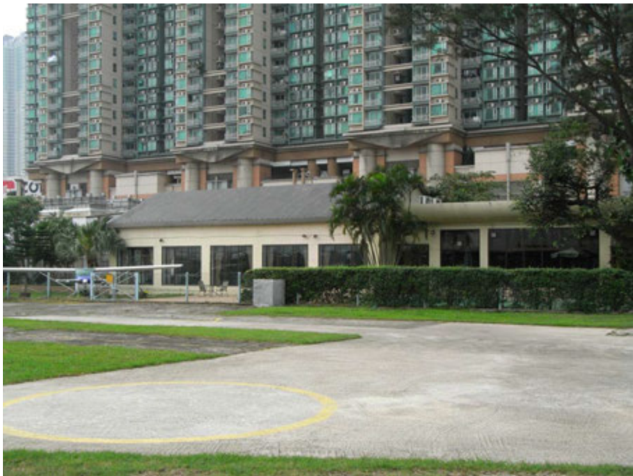
Fig. 152. External view of the Club House building facing the airfield.
