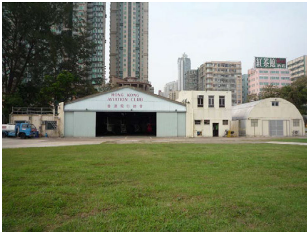
Fig. 145. Nissen Hut (right) and Hanger with an office block (left) at the former Far East Flying School, 2009.
