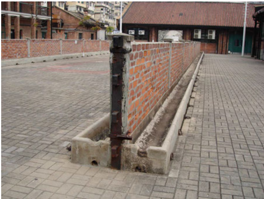
Fig. 66. Original trough at the open ground.
