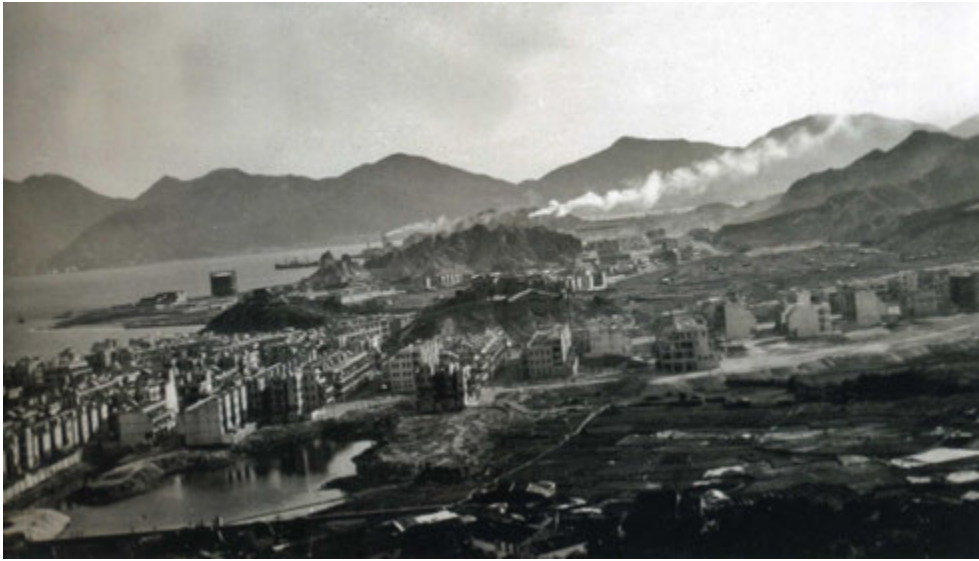
Fig. 20. Rows of tenement houses were built to the south of Kowloon Walled City, c. 1936. (from Zheng Baohong 鄭寶鴻, Early Hong Kong's Kowloon Peninsula , Hong Kong, University Museum and Art Gallery, The University of Hong Kong, 2007, p. 169.)
