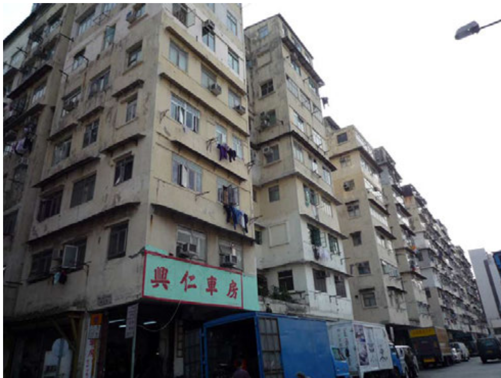
Fig. 96. The residential blocks in 3 streets, 2009.
