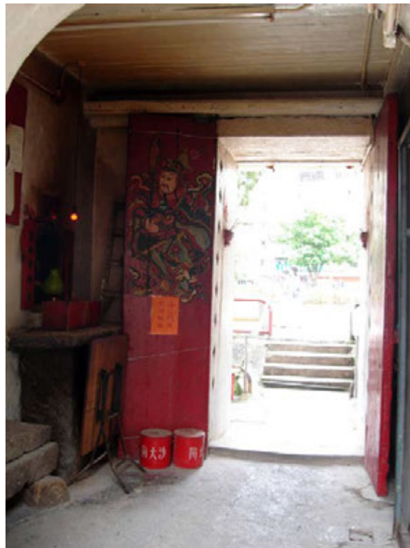
Fig. 185. Interior of the Gatehouse viewing towards the entrance gate.
