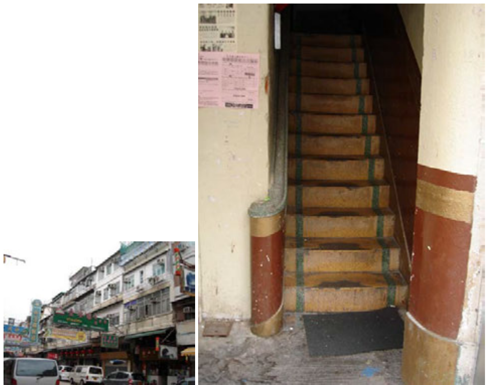
Fig. 255. Concrete staircase finished with terrazzo at Nos. 58-60 Nam Kok Road.
