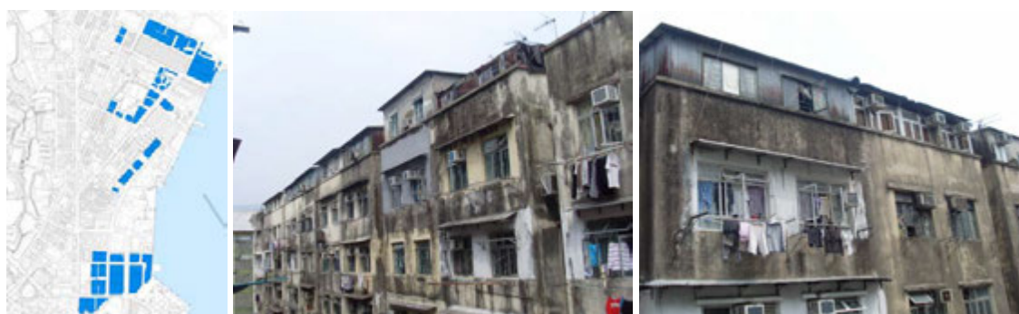
Fig. 49. Industrial block and working class residential buildings-13 Street.
