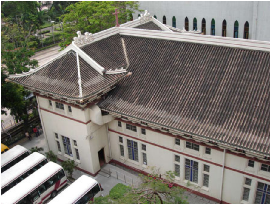
Fig. 138. An aerial view of the roof of the Holy Trinity Church.
