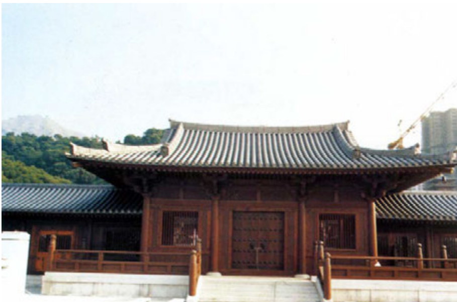
Fig. 324. Mountain gatehouse. (from Xianggang Zhi lian jing yuan fang Tang jianzhu yingzao 香港志蓮淨苑仿唐建築營造 [Hong Kong Chi Lin Nunnery modeled after Tang dynasty architecture construction], 1999, p. 14.)
