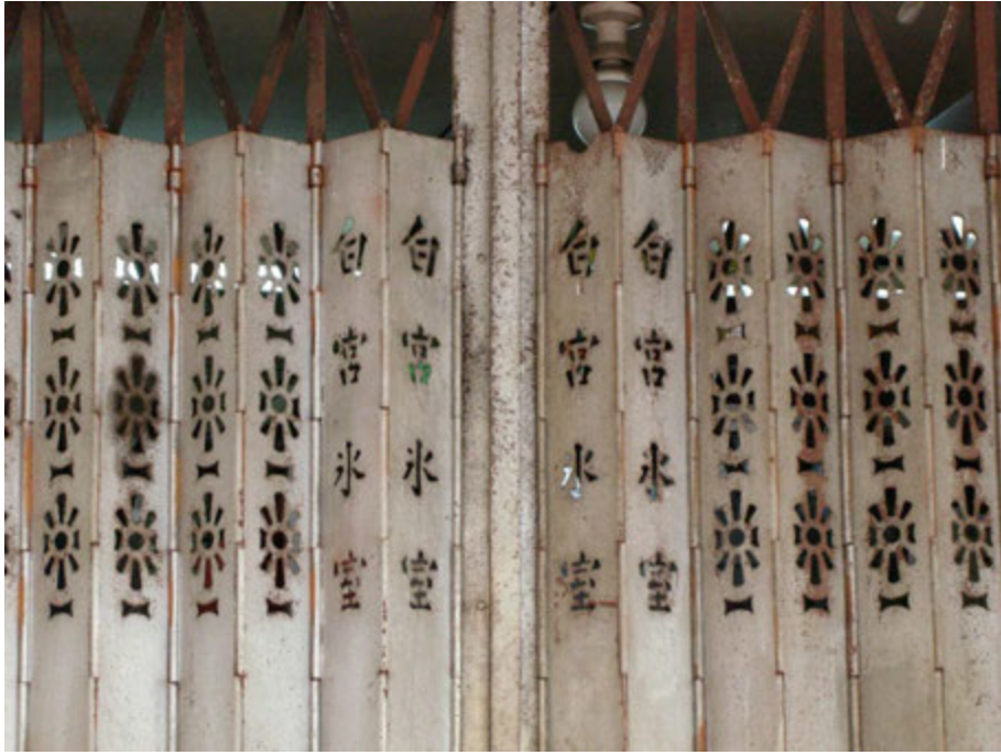
Fig. 105. Collapsible metal gate with perforated with the Chinese name of the cafe.
