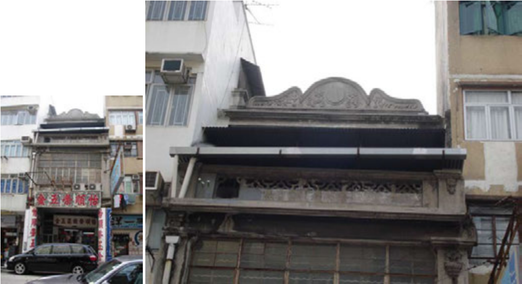
Fig. 256. Pediment with exquisite decoration and mouldings at column capitals with details at No. 3. Nam Kok Road.
