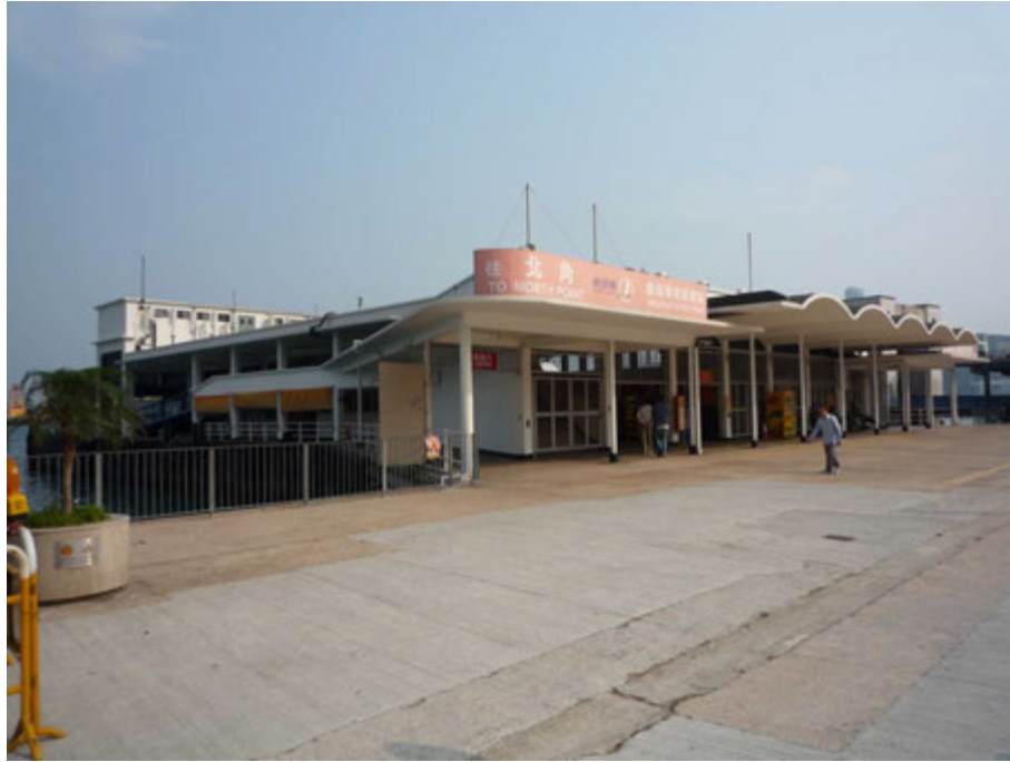
Fig. 109. Flat roof supporting on slender columns of the Kowloon City Ferry Pier.
