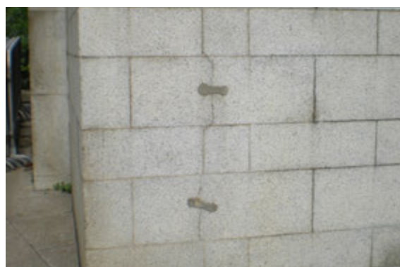
Cracks in the granite walling
