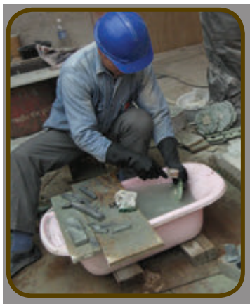
工人採用上海水磨批盪粉飾技術修復景賢里。 Workers applying the craft of Shanghai plasters finishing in the restoration of King Yin Lei.
