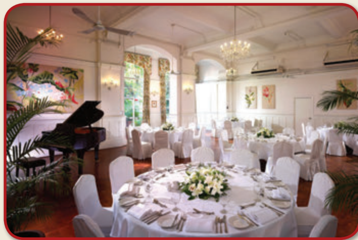
維修資助計劃使花園廳內的保養牆身工程得以進行。 The Financial Assistance Scheme enables maintenance works to be applied to the Garden Room's walls.
