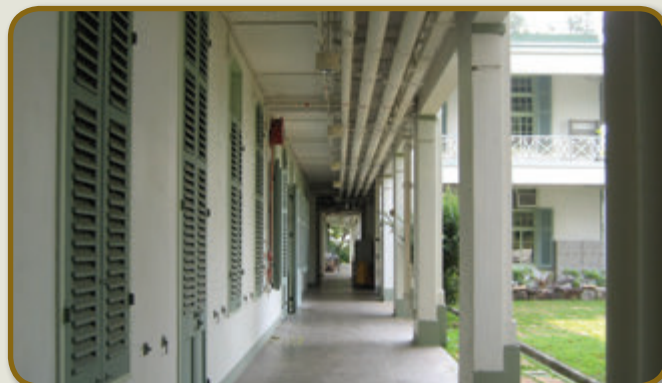
走廊有助對流、採光及通風。 The verandah enables good circulation, natural lighting and ventilation.
