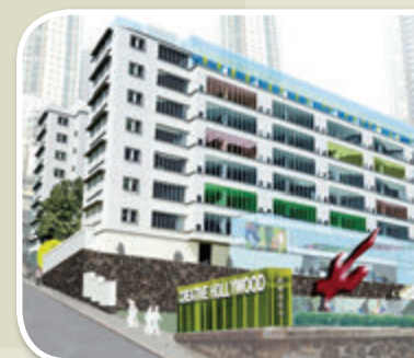
荷李活道已婚警察宿舍 Police Married Quarters at Hollywood Road
