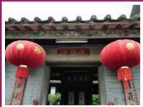
復修前 Before restoration
