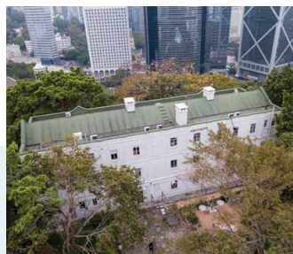
「母親的抉擇」堅尼地道辦公室 (舊域多利軍營蒙高瑪利樓) Kennedy Road Office, Mother's Choice (Montgomery Block, Old Victoria Barracks)
